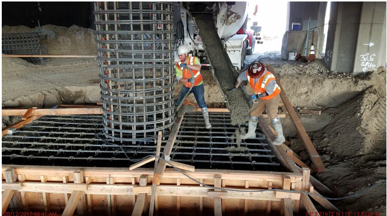
Pouring footing for Ped Bridge C5.
