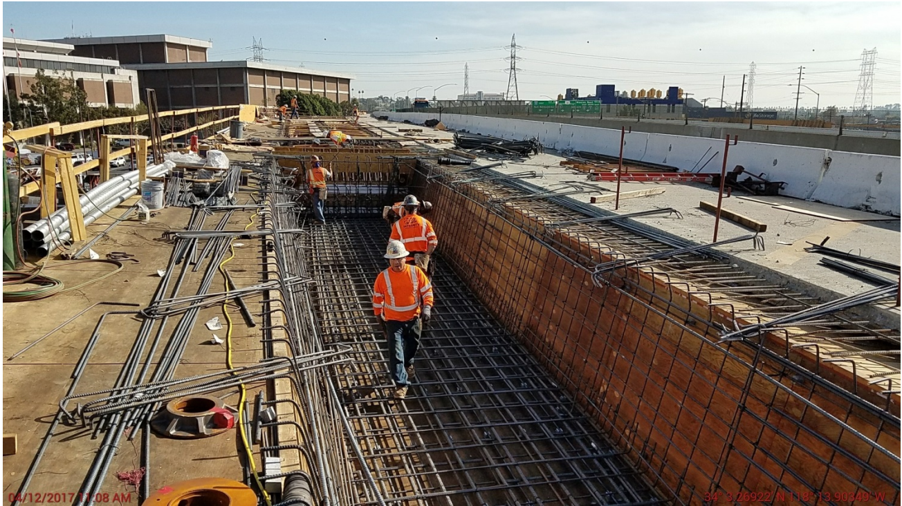
Frame 1 left rebar installation.
