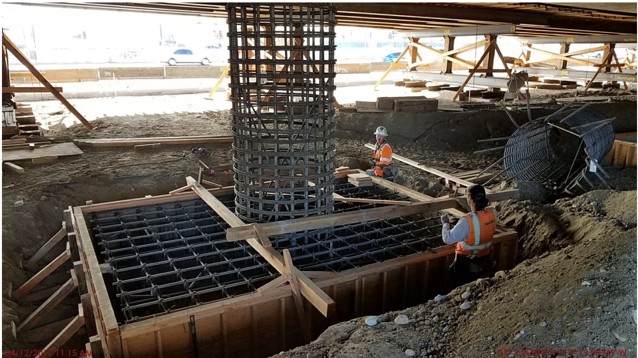
Addition of Kickers at Bent C6.
