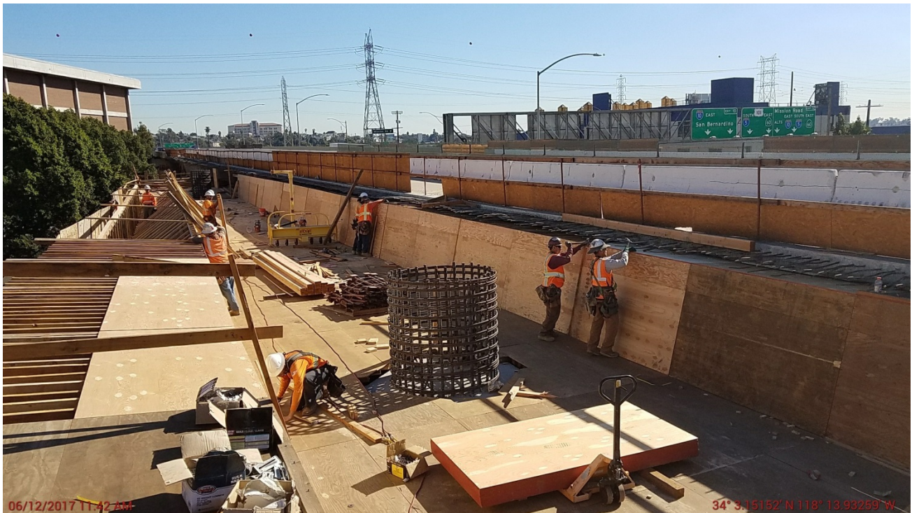
Forming exterior soffit stems.
