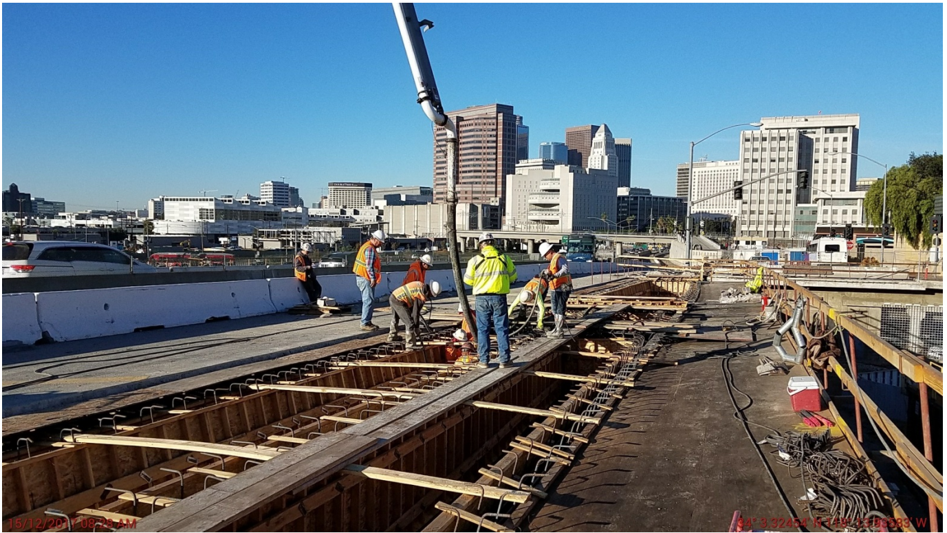
Pouring stems and soffit at Frame 2 Left.
