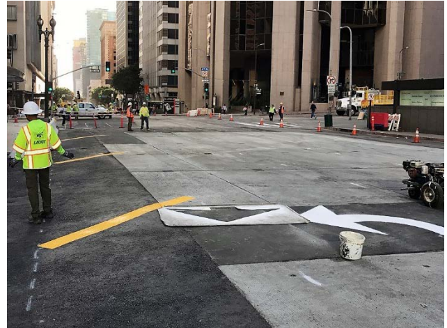
6 th Street Re-opening (Flower Street looking South)
