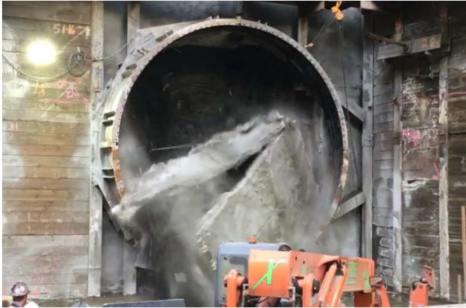
TBM Breakthrough at Grand Av Arts/Bunker Hill Station
