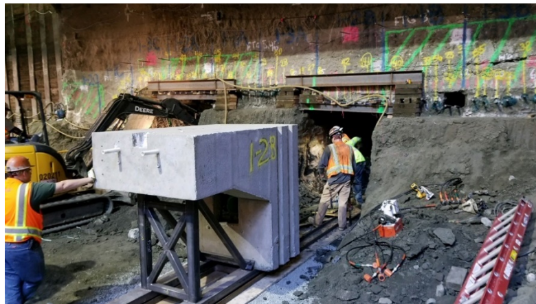
Underpinning of LA Times building Historic Broadway Station
