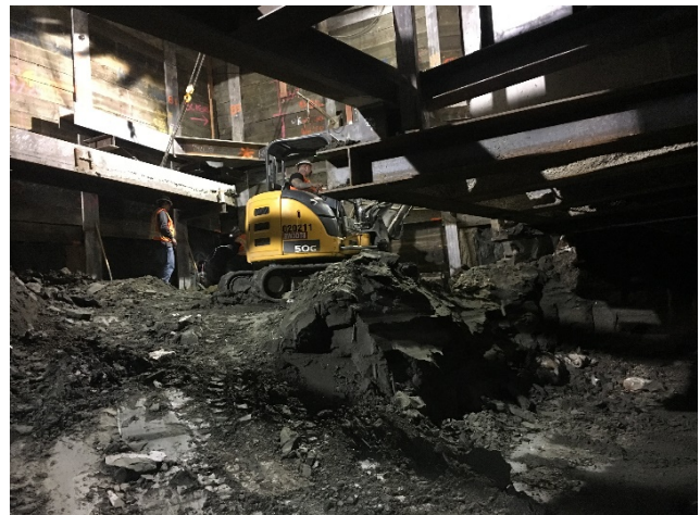
Excavation under decking on Flower Street
