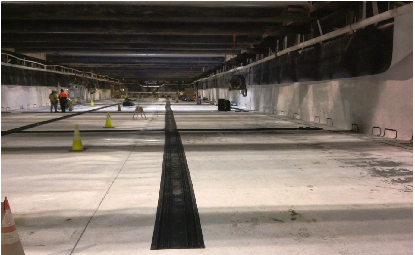
Wilshire/La Brea Station HDPE Installation Looking East
