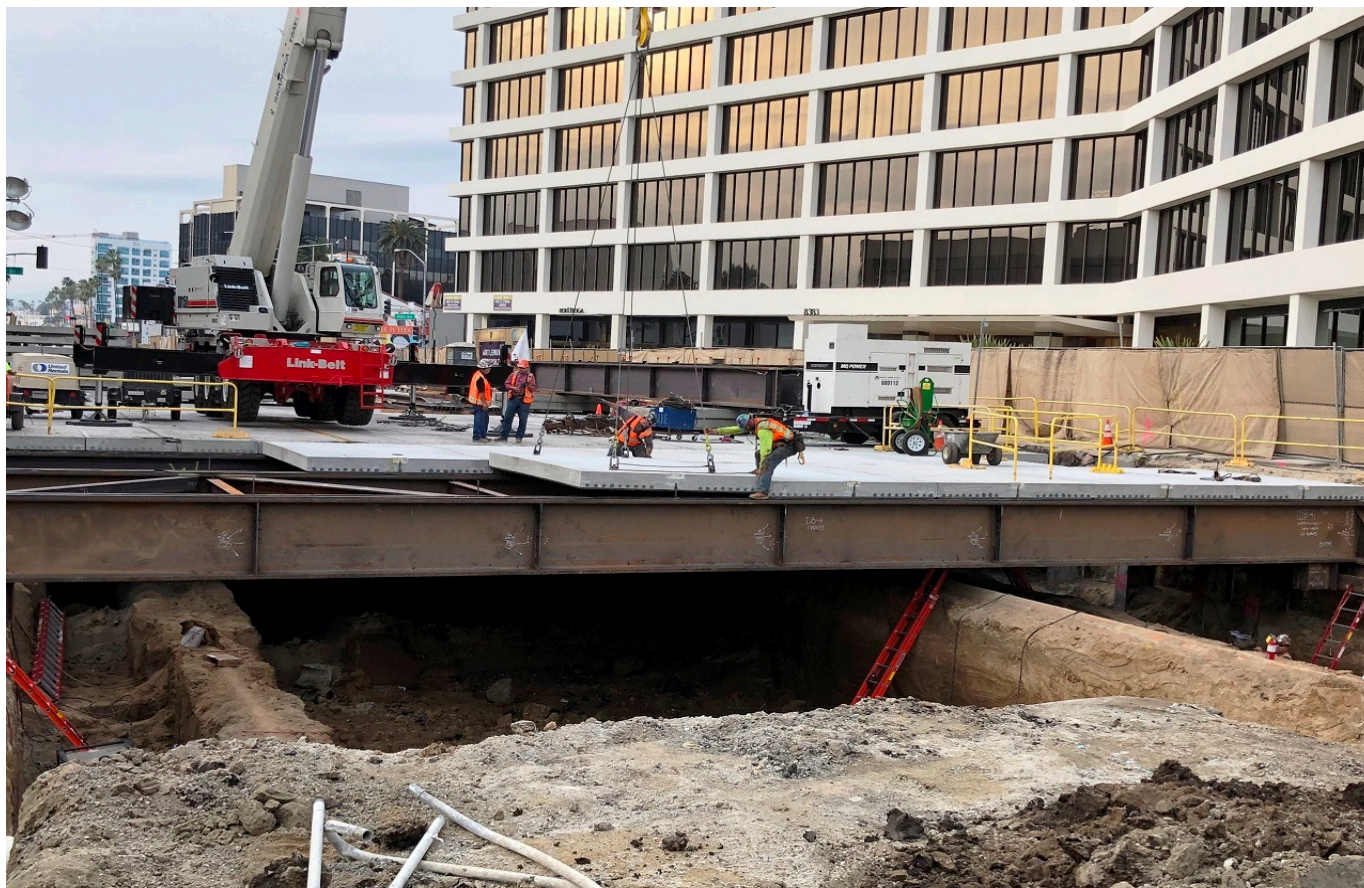
Wilshire/La Cienega Station Street Decking Operation
