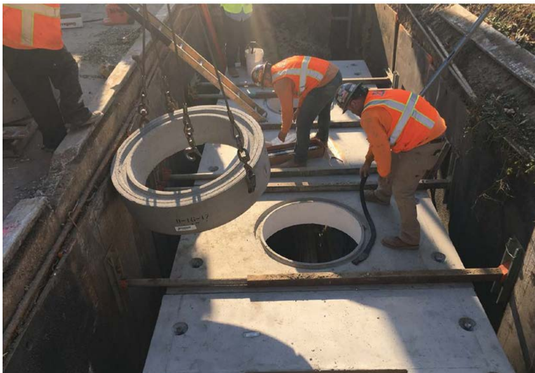
AT&T Manhole Installation in Century City
