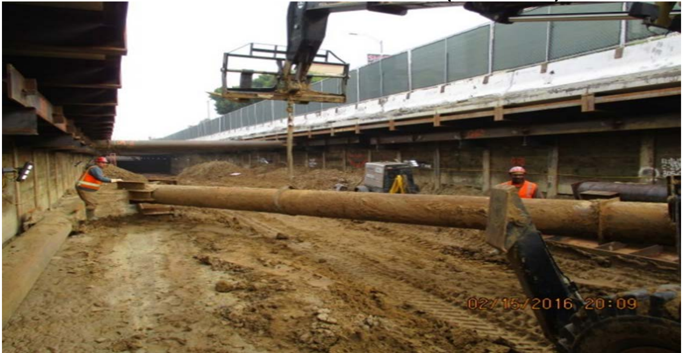
UG#3 – Installation of struts near 60th St.
