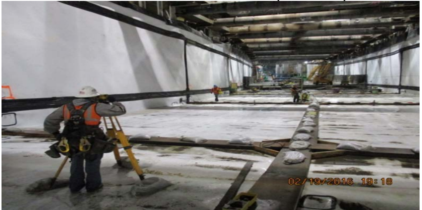
UG#4 – Waterproofing near Leimert Park Station.
