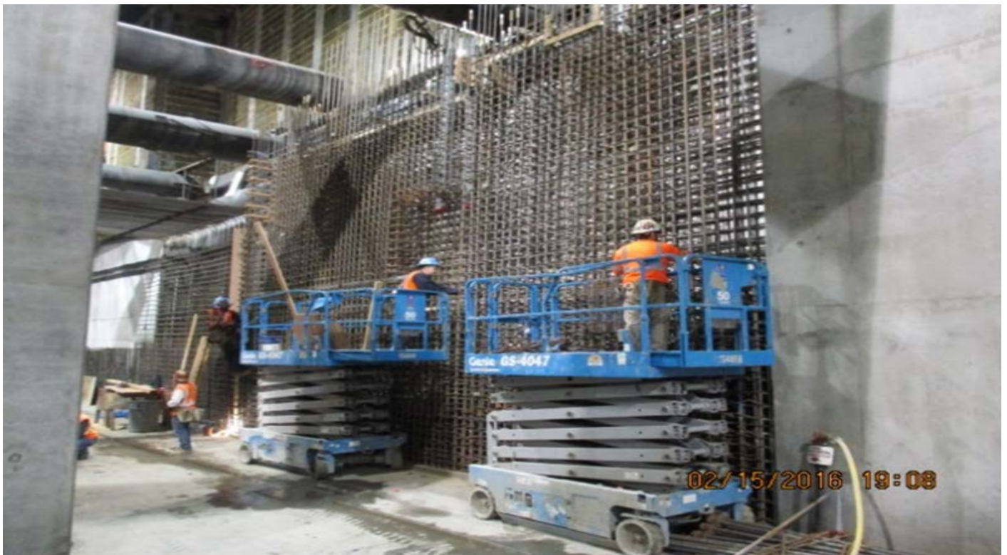
LEIMERT PARK STATION – Preparing lower wall for concrete placement.
