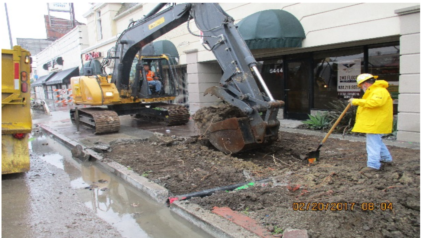
PARK MESA – Removal of east sidewalk north of 57th St.
