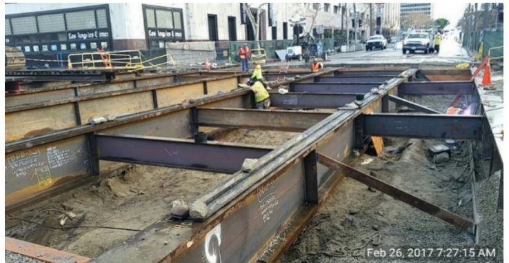
Decking at the 2nd/Spring Intersection
