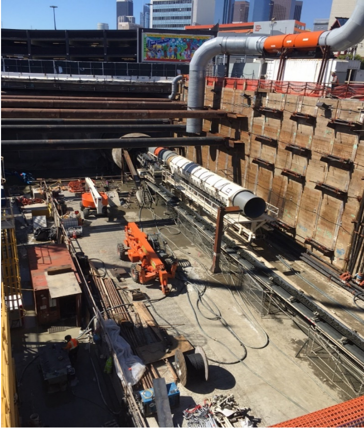
Tunneling operations underway
