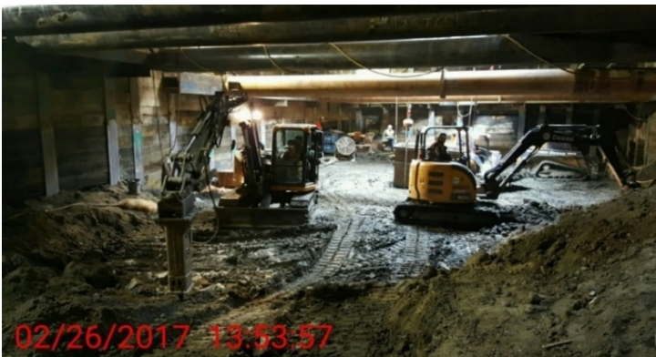
Demolition of abandoned Pacific Electric Tunnel and Shaft Excavation
