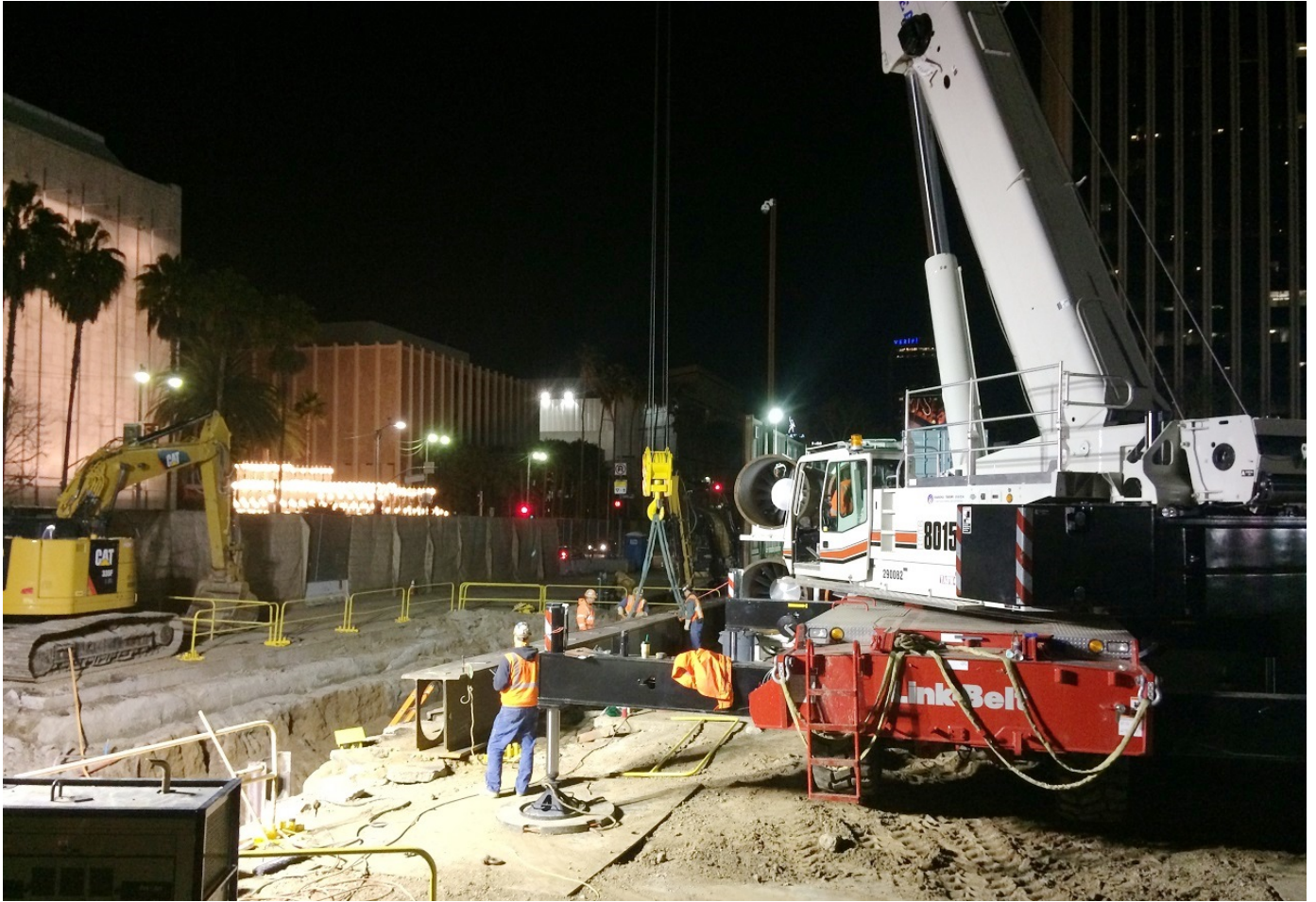
Wilshire/Fairfax Station Deck Beam and Decking Installation Activities
