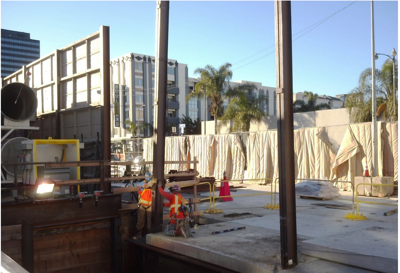
Soundwall Installation at Wilshire/La Brea Station South Muck Shaft
