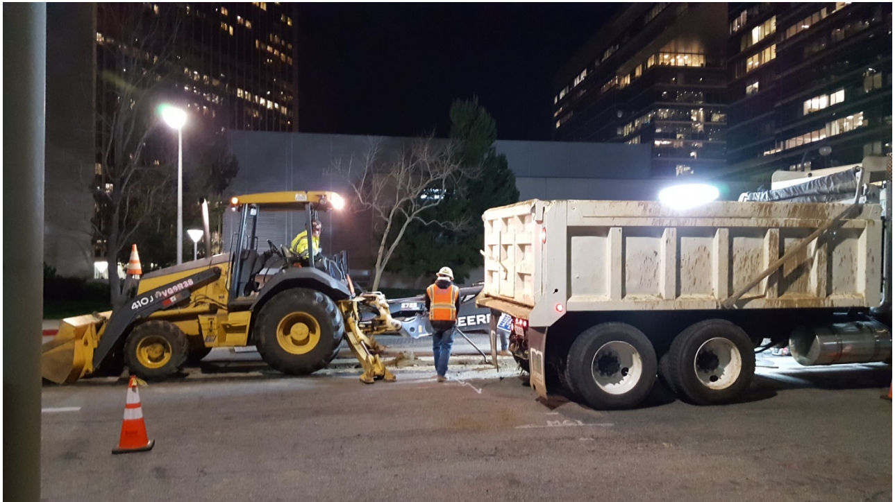
Century City Constellation Joint Trench
