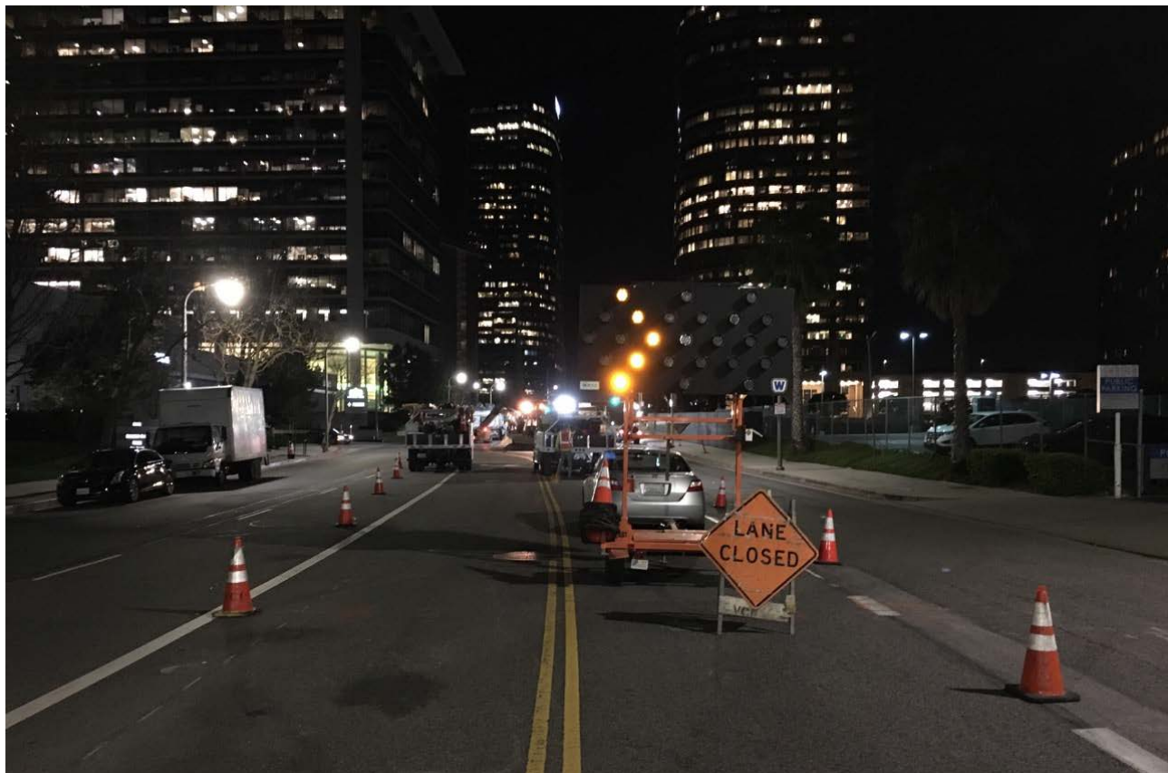
Century City Constellation Joint Trench
