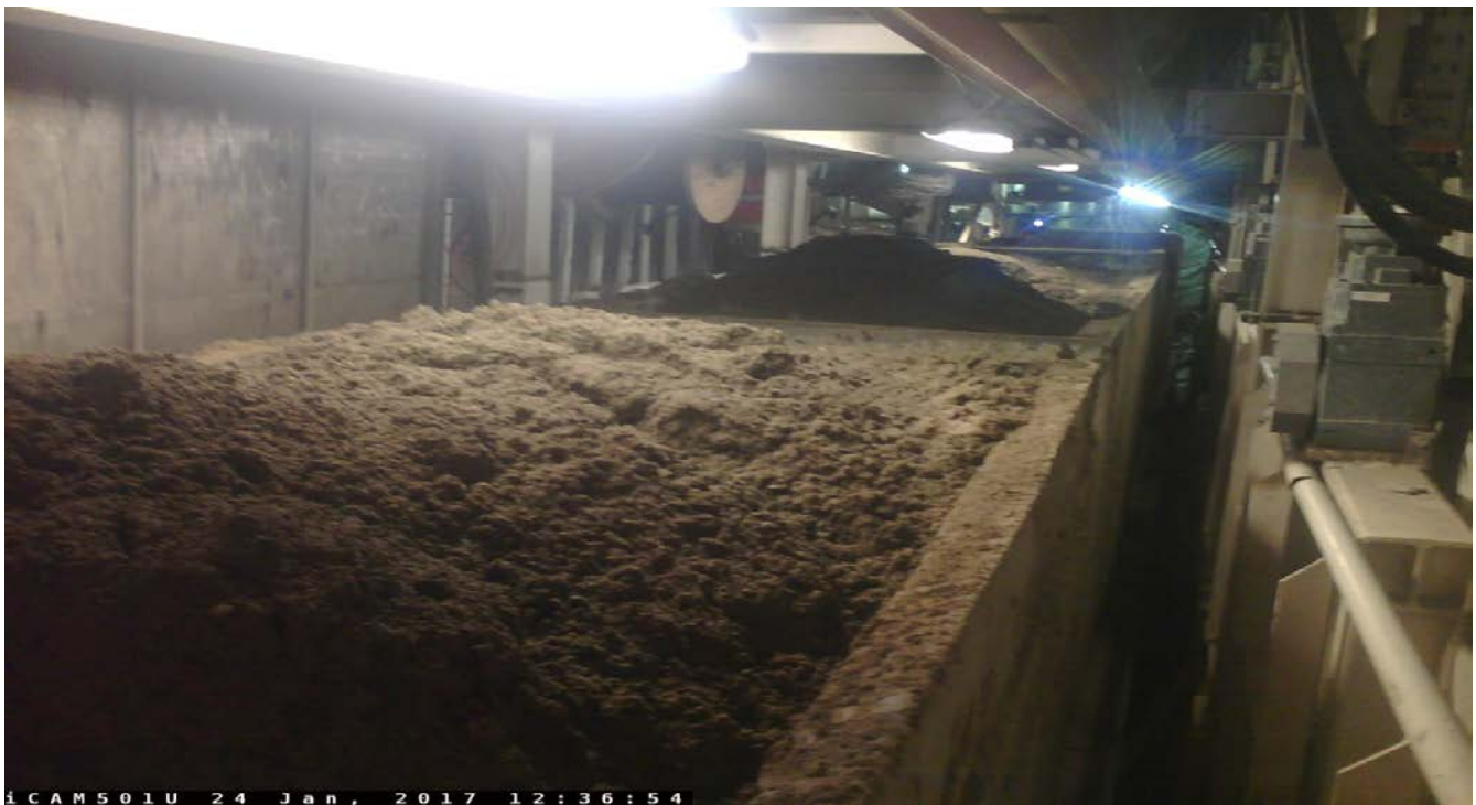
TUNNELING – Removing muck from TBM advance.
