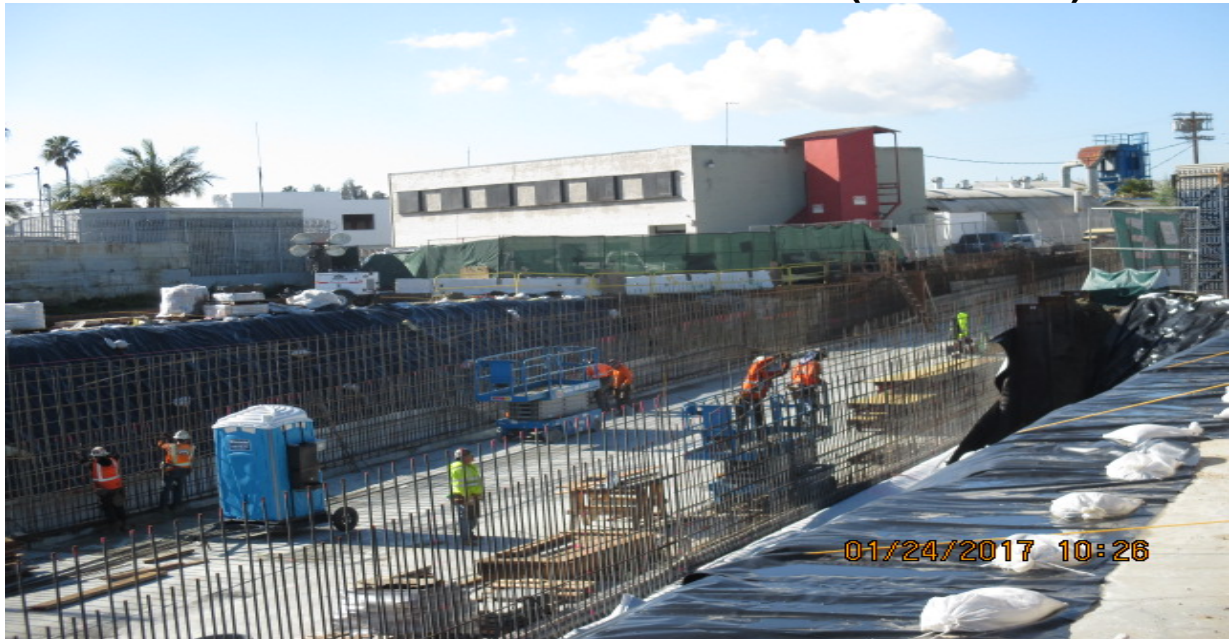
UG#3 – Installation of rebar for U-channel walls at south portal.
