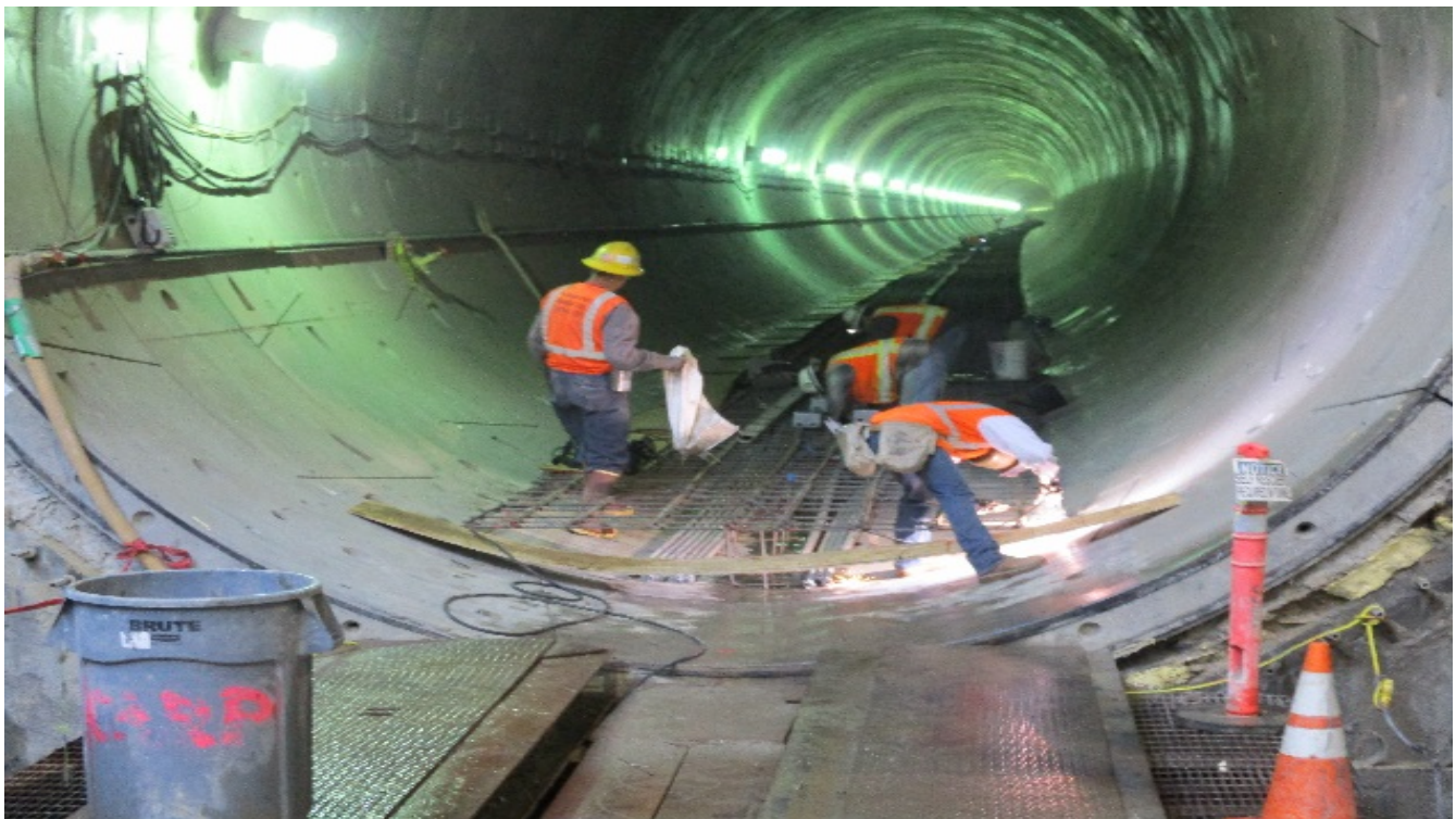
TUNNELING – Preparing SB Tunnel for invert.
