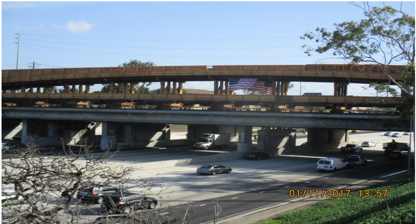
(AG-5) I-405 Bridge – View of AG-5 from the I-405.
