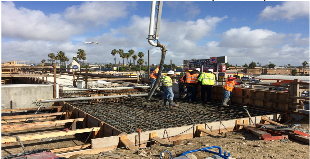
AVIATION/CENTURY BRIDGE – Concrete placement complete for both approach slabs at abutment 1.
