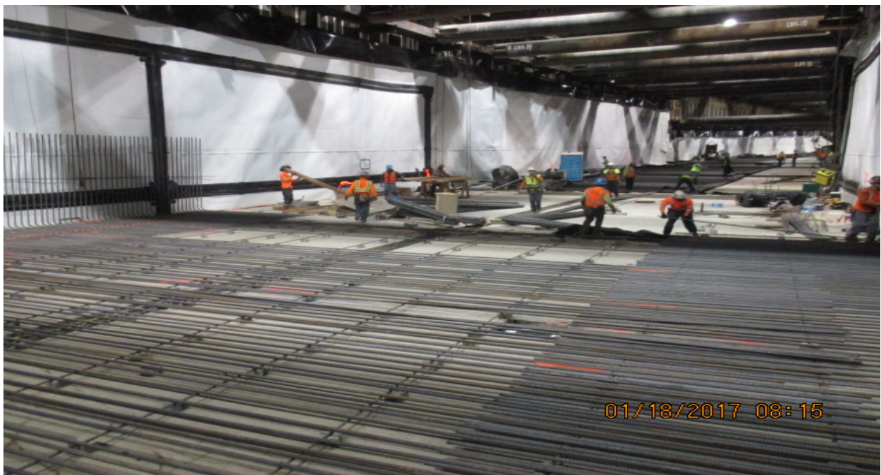
UG#4 – Installation of rebar for invert section I-27 at north portal.
