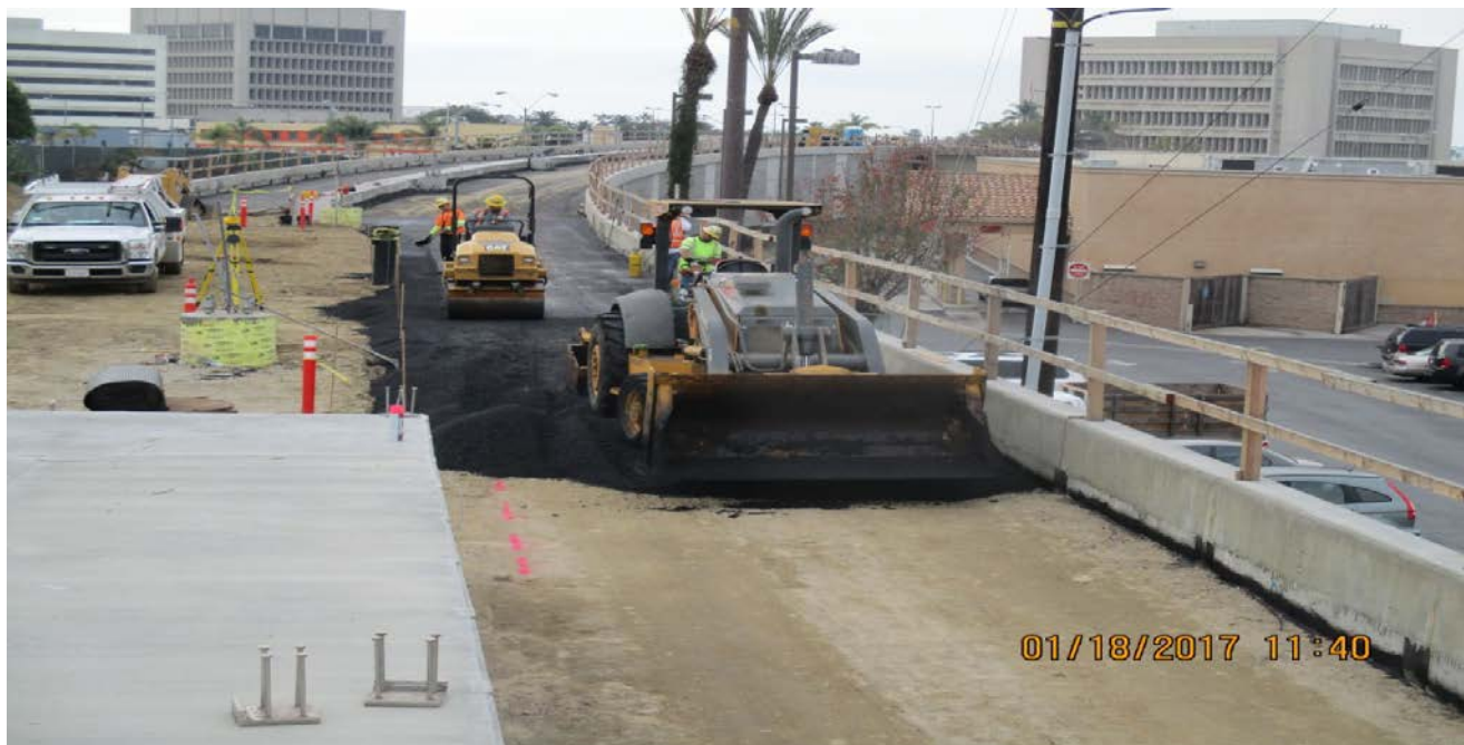
(AG-6) LA BREA BRIDGE –. Crews worked on placing the Asphalt cap.
