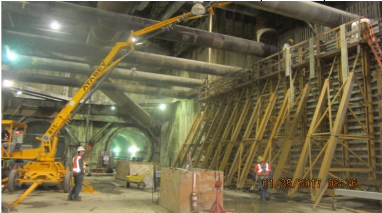
MARTIN LUTHER KING JR. STATION – Placement of lower wall section LW-4.
