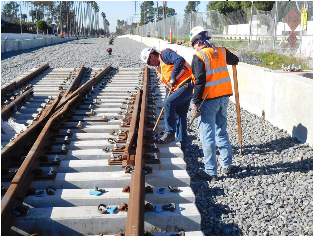
Bottom ballast being placed and start of ballasted special track work.
