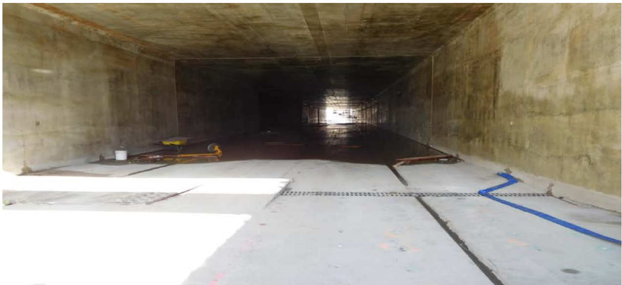
UG#1 -C&C Tunnel STA 45+00 to 50+00.
