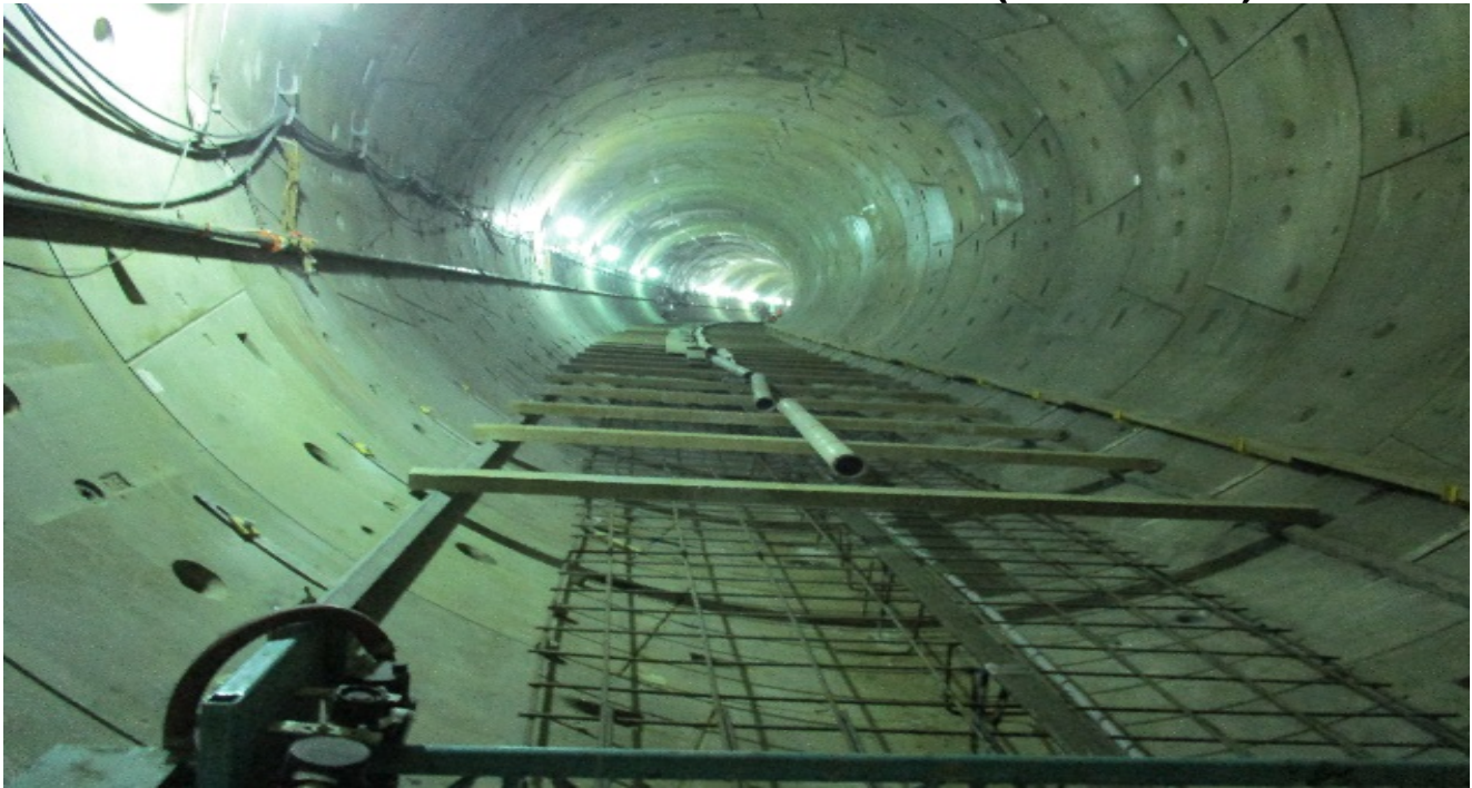
TUNNELING – Installation of electrical conduits and SB Tunnel Invert rebar
