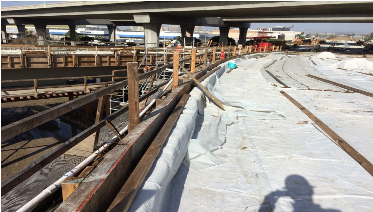
GREENLINE UNDERPASS – Frame 1: Deck concrete cure.
