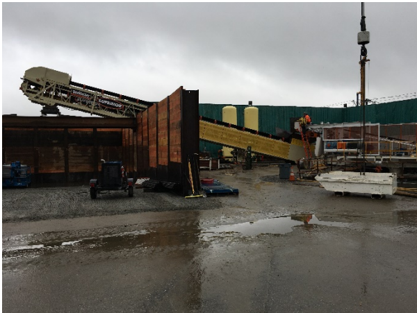
Muck conveyor at Mangrove/Launch Pit
