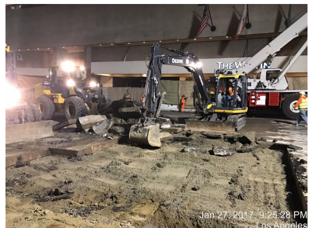
Removal of asphalt for Decking along Flower
