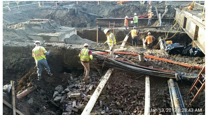
Excavation and utility exposure in 2 nd Street
