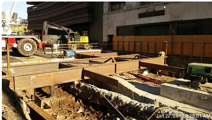
Decking on 2 nd Street
