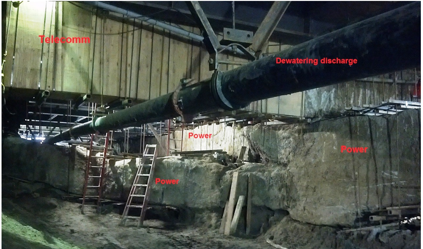
Support of Utilities under the Deck at Wilshire/La Brea Station
