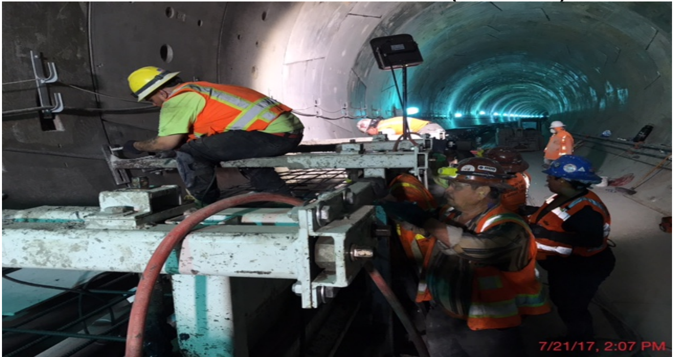
TUNNELING – Placement of SB Tunnel Walkway section 7a.
