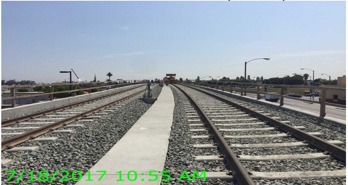
MSE 192 - Wall complete, ballasted trackwork in-place (surface & line and de-stressing complete).
