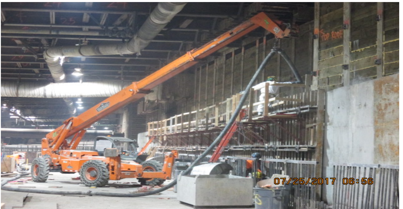
LEIMERT PARK STATION - Completed placement of west concourse level sand wall.
