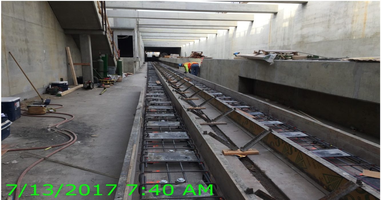
UG1 - Forming plinths.
