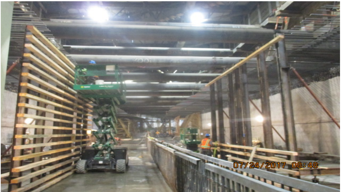
UG4 – Fabrication of Center Wall formwork.
