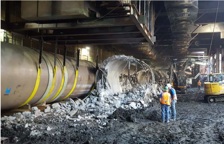
LA County storm drain demolition adjacent to Hobas
