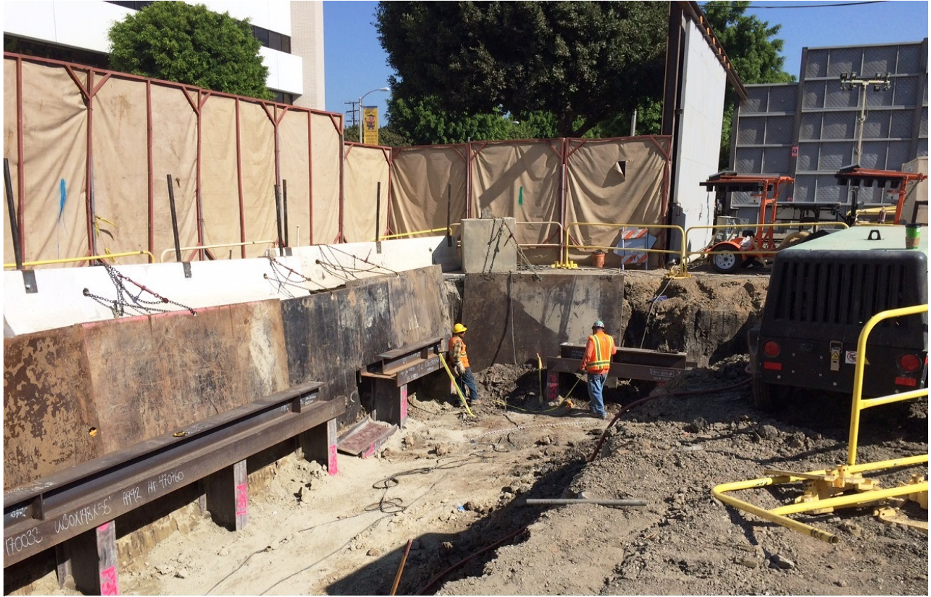
Securing Cap Beams at Wilshire/La Cienega Station
