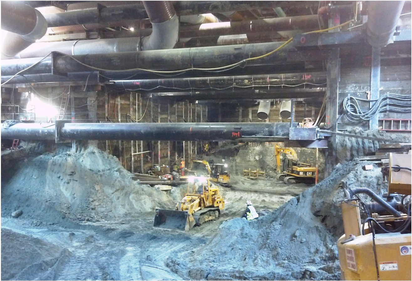
Under Deck Excavation at Wilshire/La Brea Station
