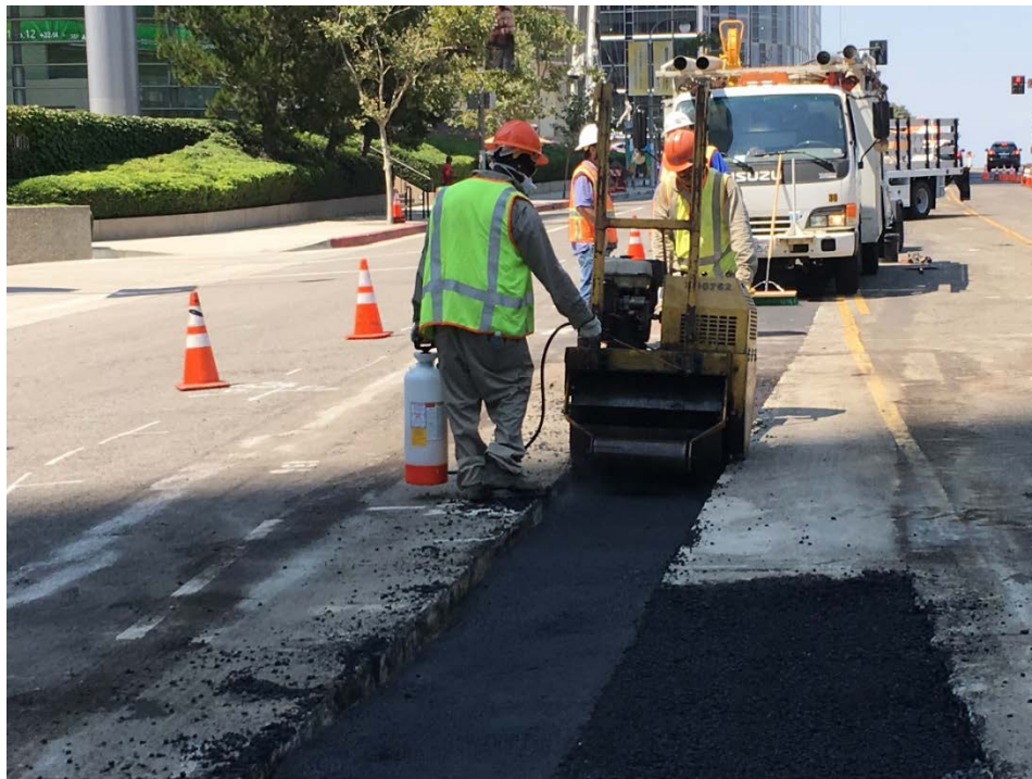
LAWDP Power relocation work in Century City
