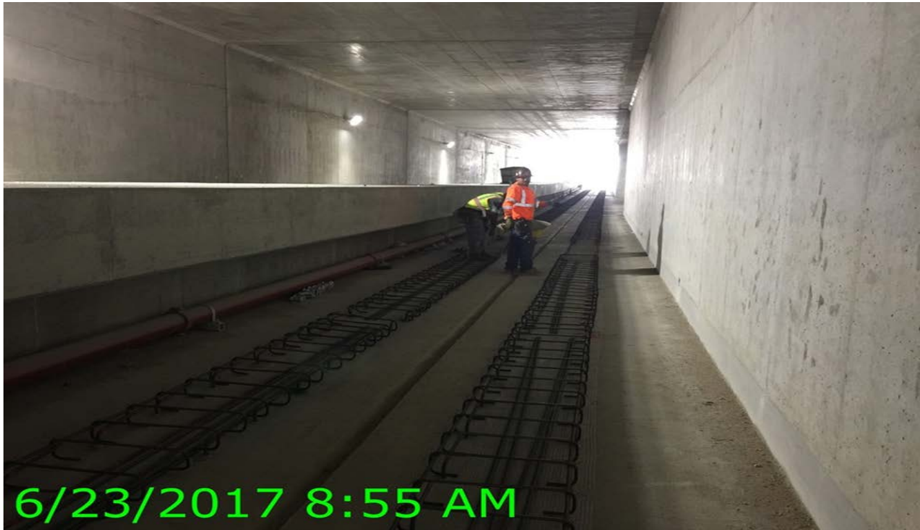
UG#1 – UG1 plinth construction underway.
