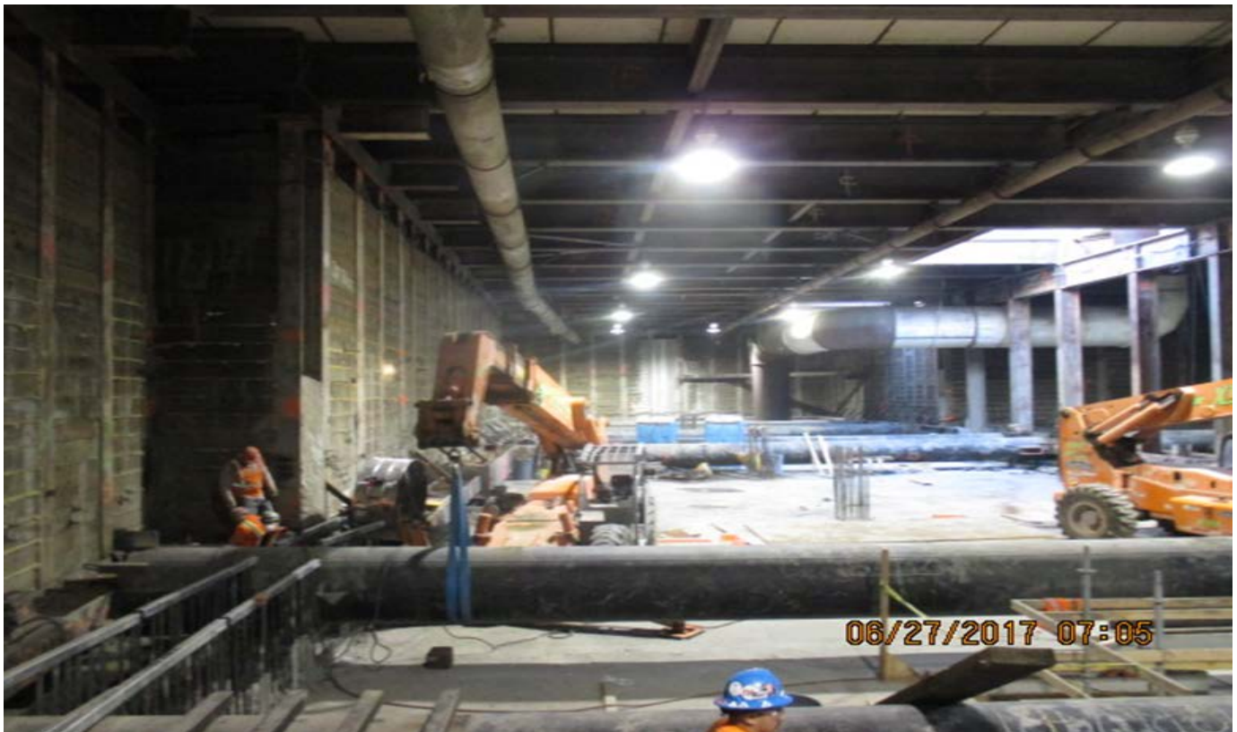
LEIMERT PARK STATION – Removing Tier-2 struts.
