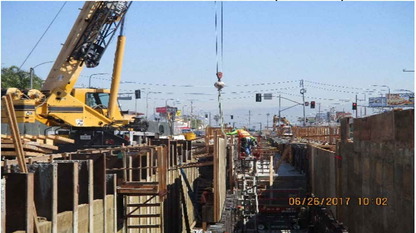
HYDE PARK STATION - Installation of formwork for walls at TC&C room.
