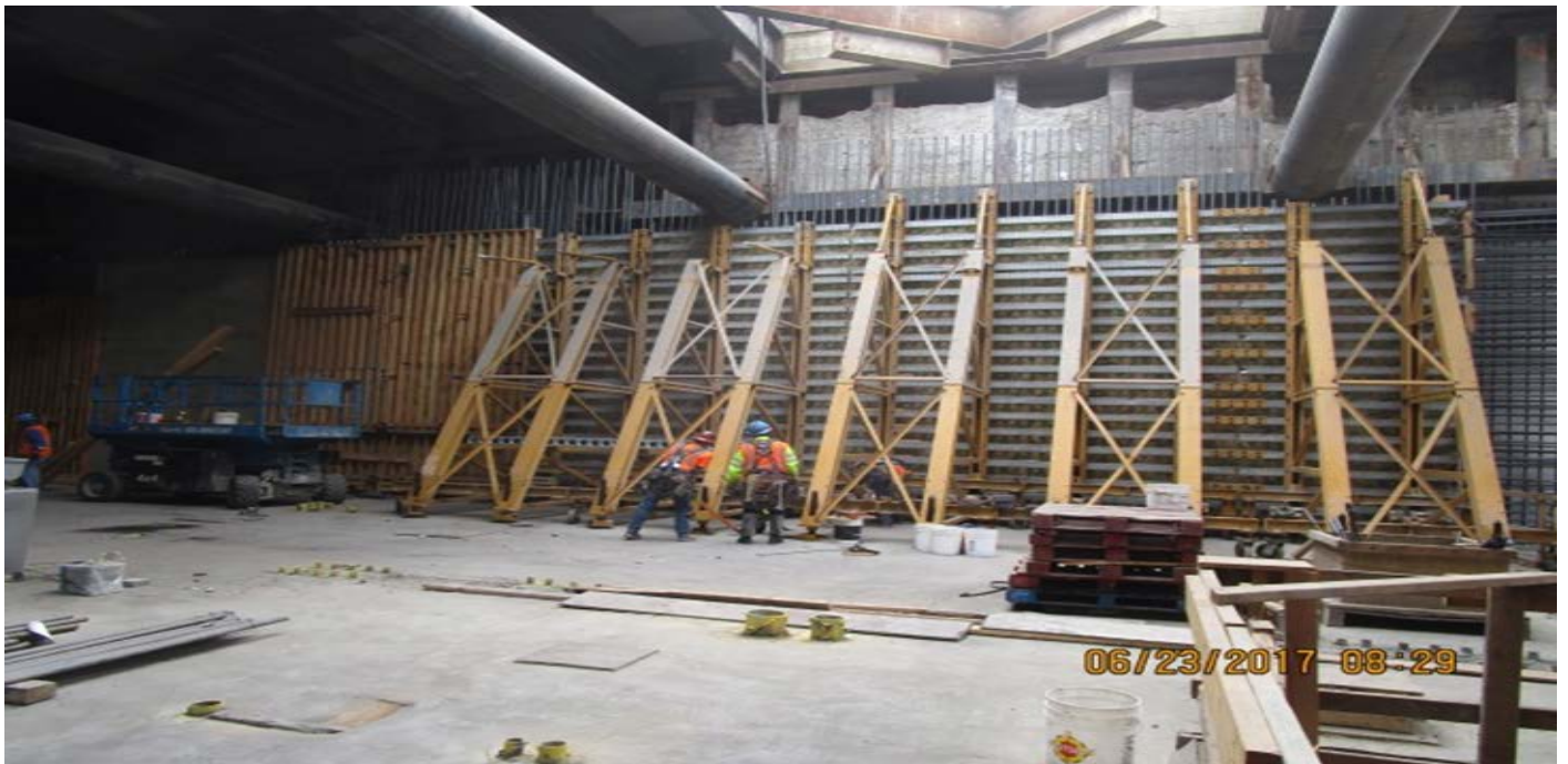
EXPOSITION/CRENSHAW STATION – Installation of formwork for concourse level wall section G-28.
