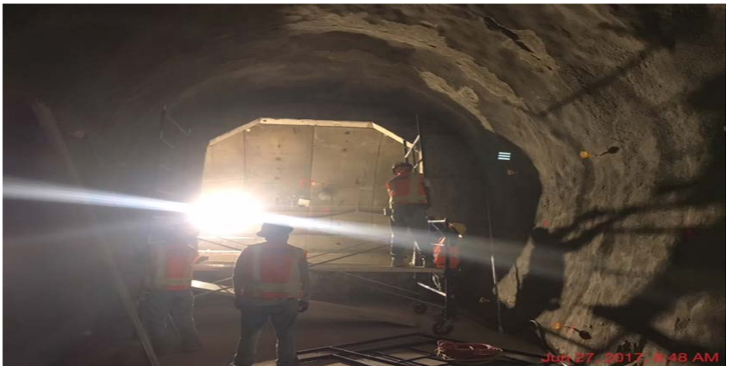
TUNNELING – Smoothing shotcrete completed at CP-5 for waterproofing.
