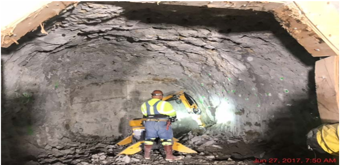
TUNNELING – Excavation of jet-grouted soils at CP-4.
