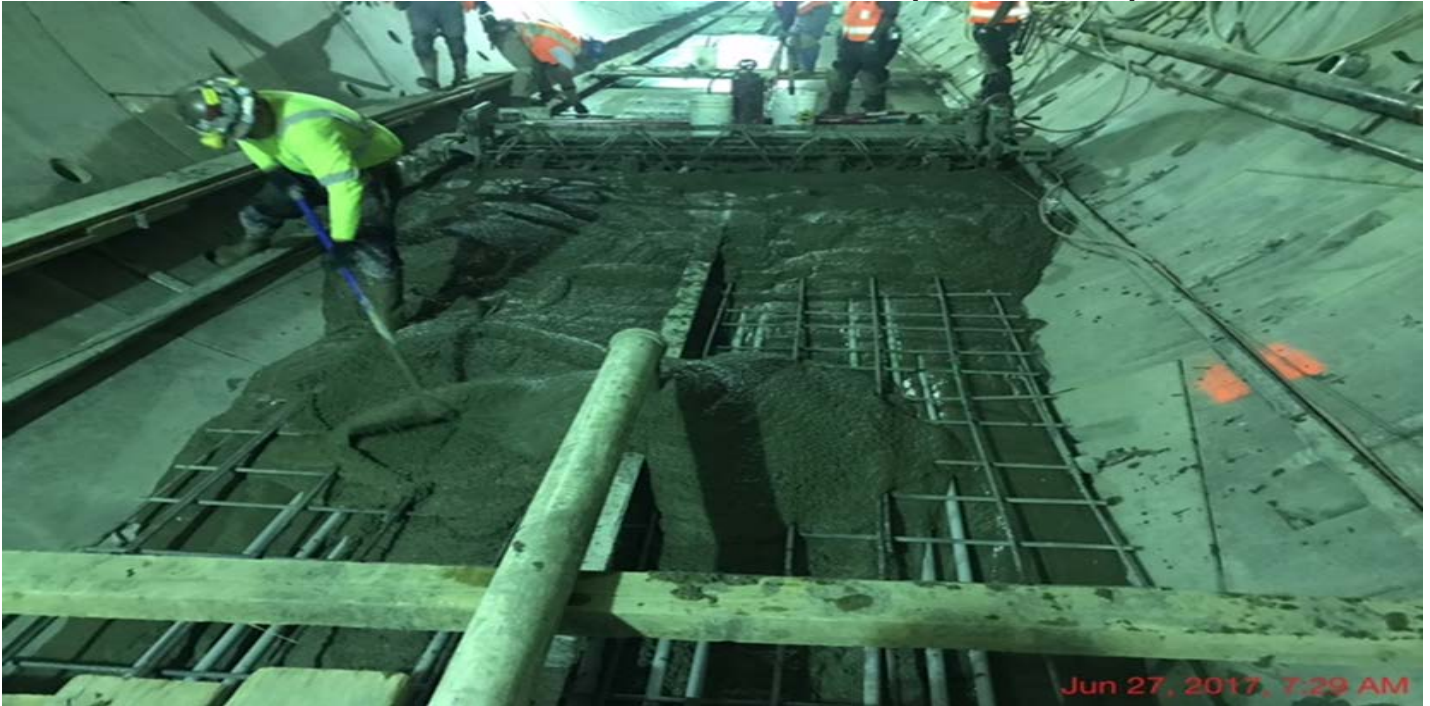
TUNNELING – Placement of NB Tunnel Invert section 10.
