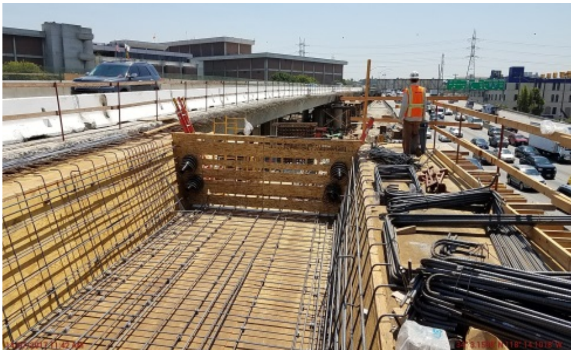
Frame 1 soffit/stem rebar installation.
