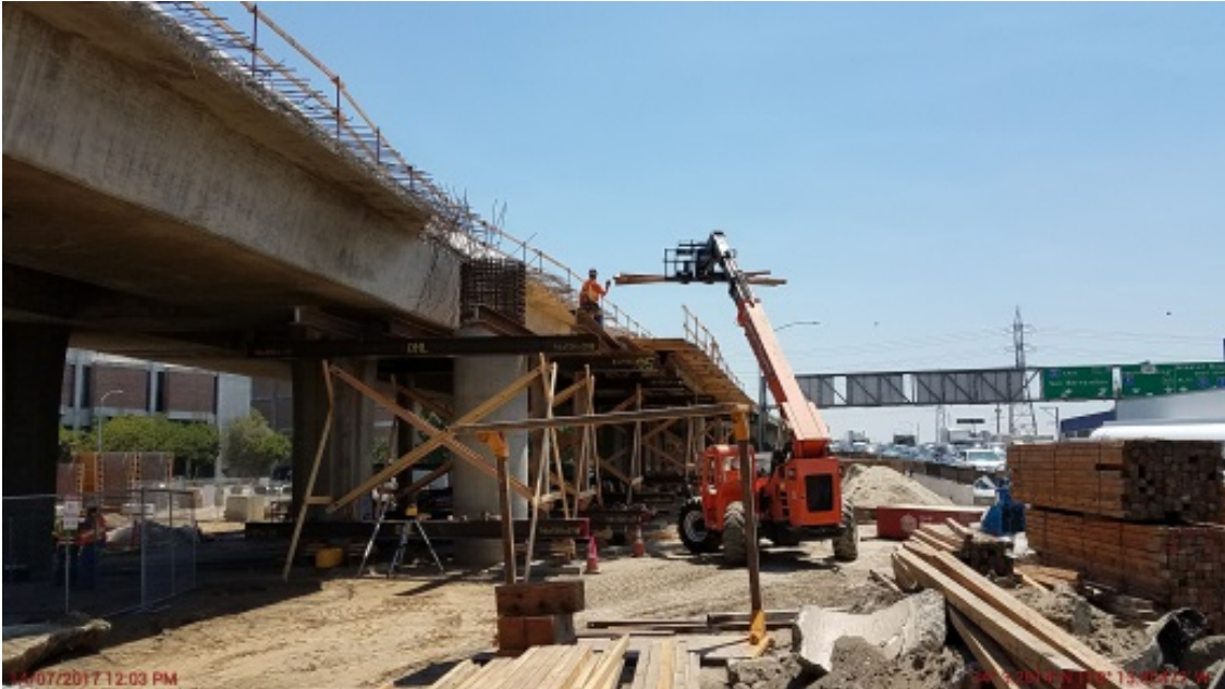
Frame 3 Falsework installation.
