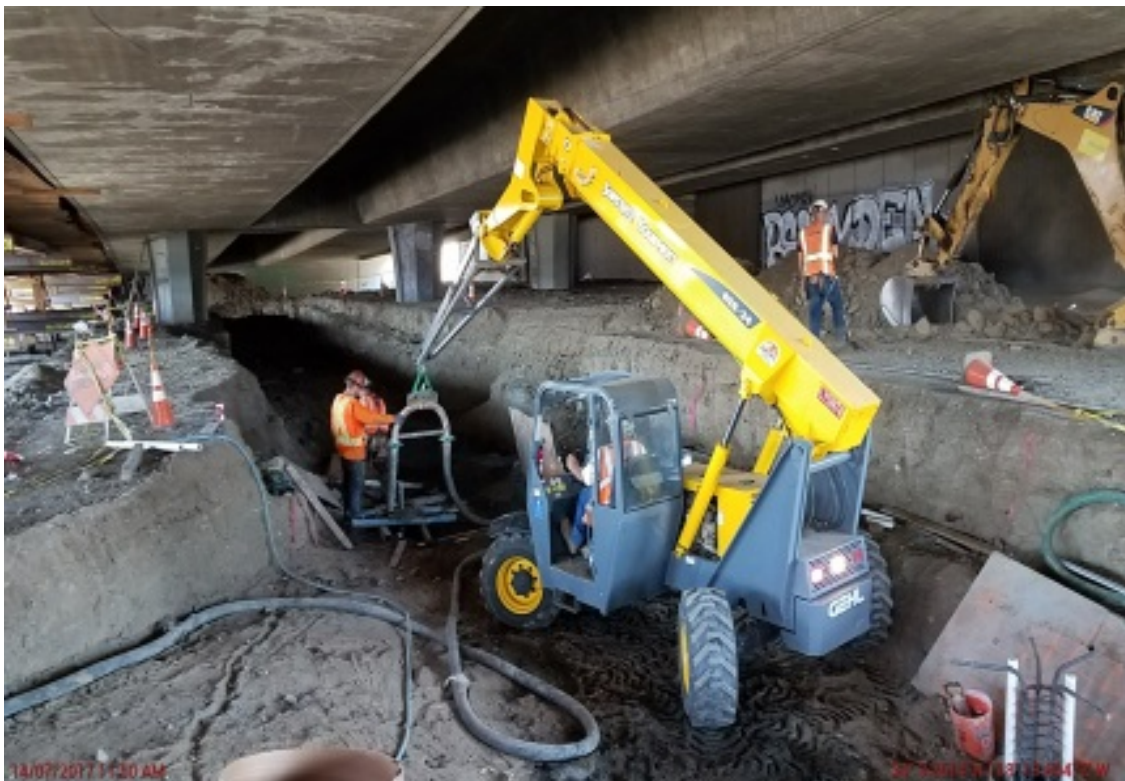
Pedestrian overcrossing piles.
