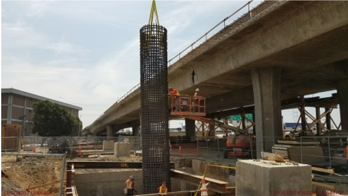
Column cage at Bent 6.
