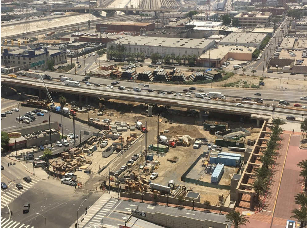
Photo provides an aerial view of the jobsite from the south side of the Metro Gateway Building.
