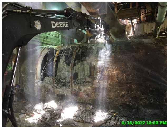
LA County storm drain demo and removal at 2 nd /Broadway
