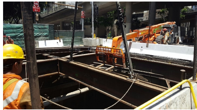
Preparation for Gantry Crane and TBM Retrieval
