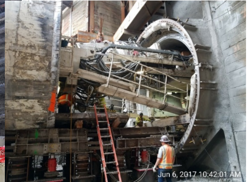
TBM crossing (walkthrough) at Grand Av Arts/Bunker Hill Station
