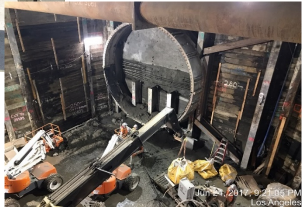
Installing fiberglass rebar at tunnel eye
