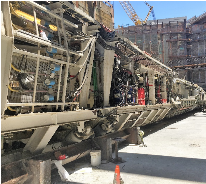
TBM in Grand Av Arts/Bunker Hill Station
