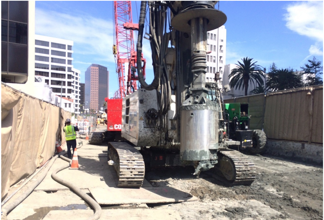
Wilshire/La Cienega Piling Operation in Progress
