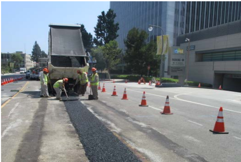
LAWDP water relocation work in Century City
