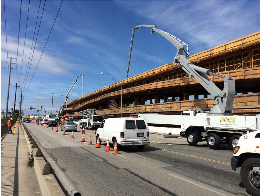
Contractor placing concrete for I-405 bridge span.
