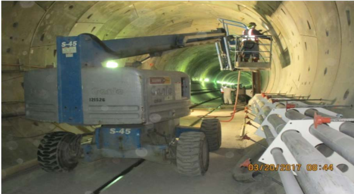
Check grouting at Cross Passage 4 – SB Tunnel.
