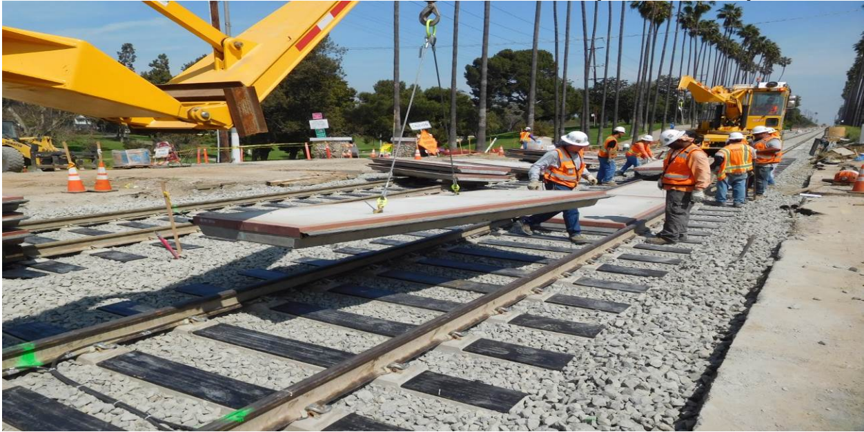
Centinela Avenue grade crossing - Crossing panel installation.
