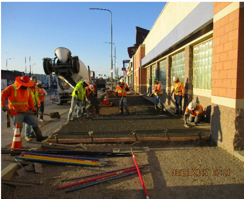
Park Mesa – Placement of west sidewalk between 54 th and 57 th St.
