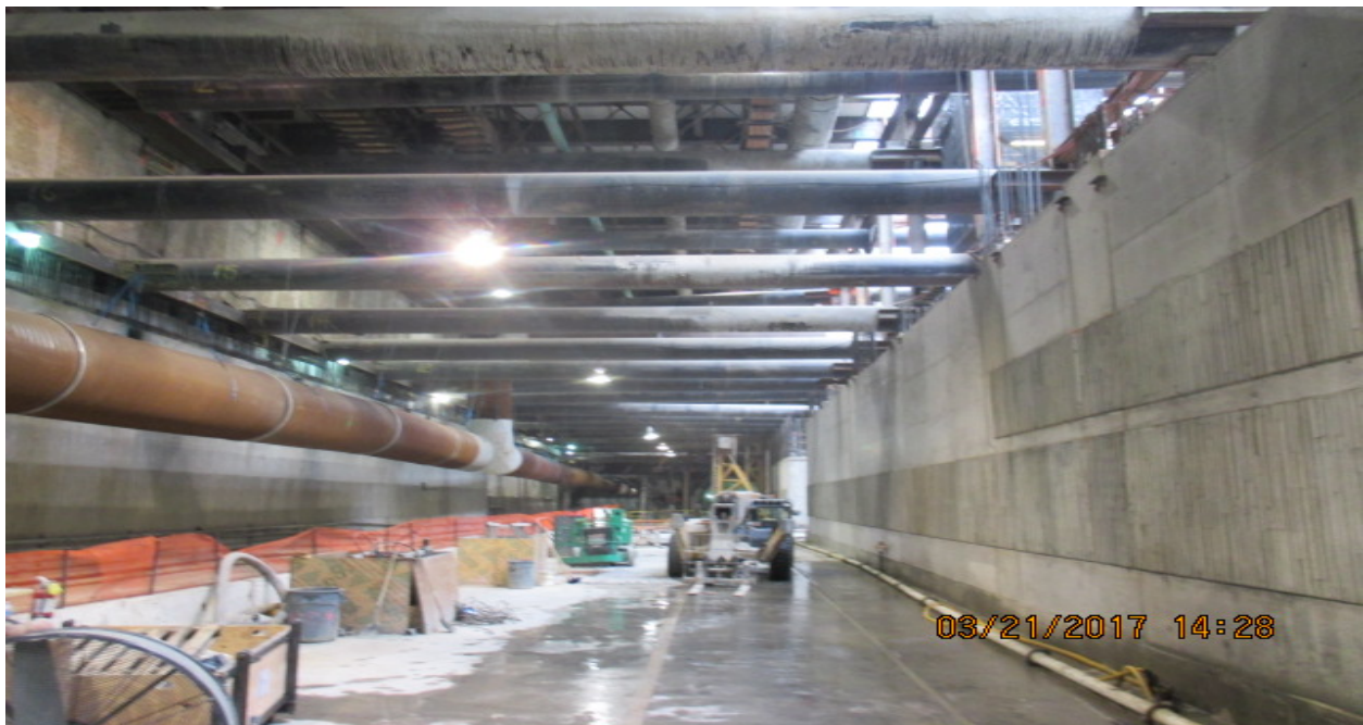
Completed section of lower interior wall in MLK Jr. Station.
