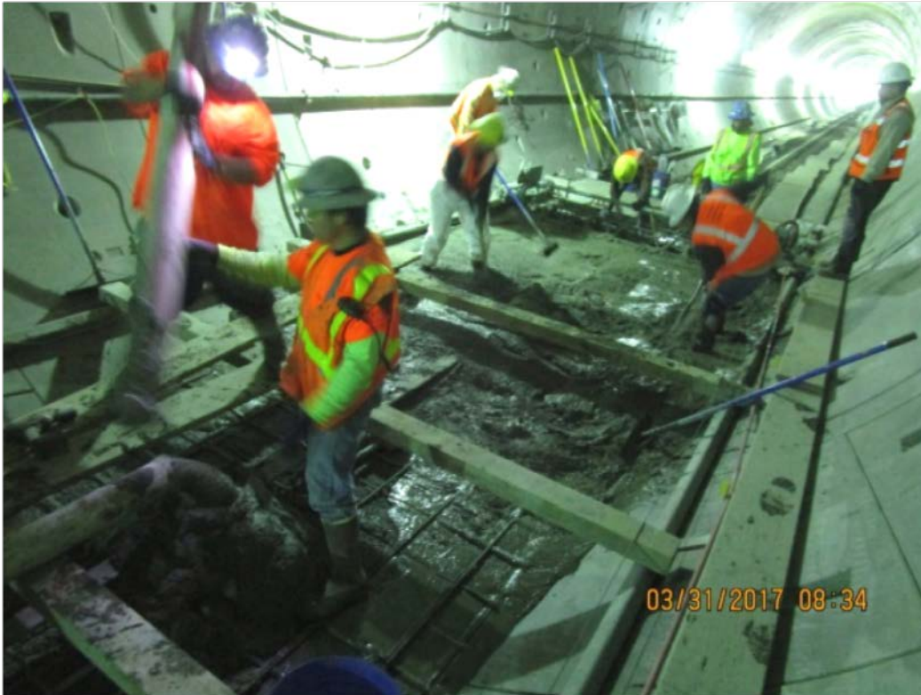
Placement of SB Tunnel invert.
