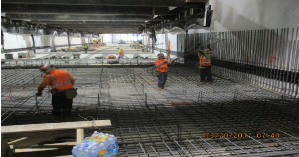
. UG4 – Installation of rebar for invert section I-23.
