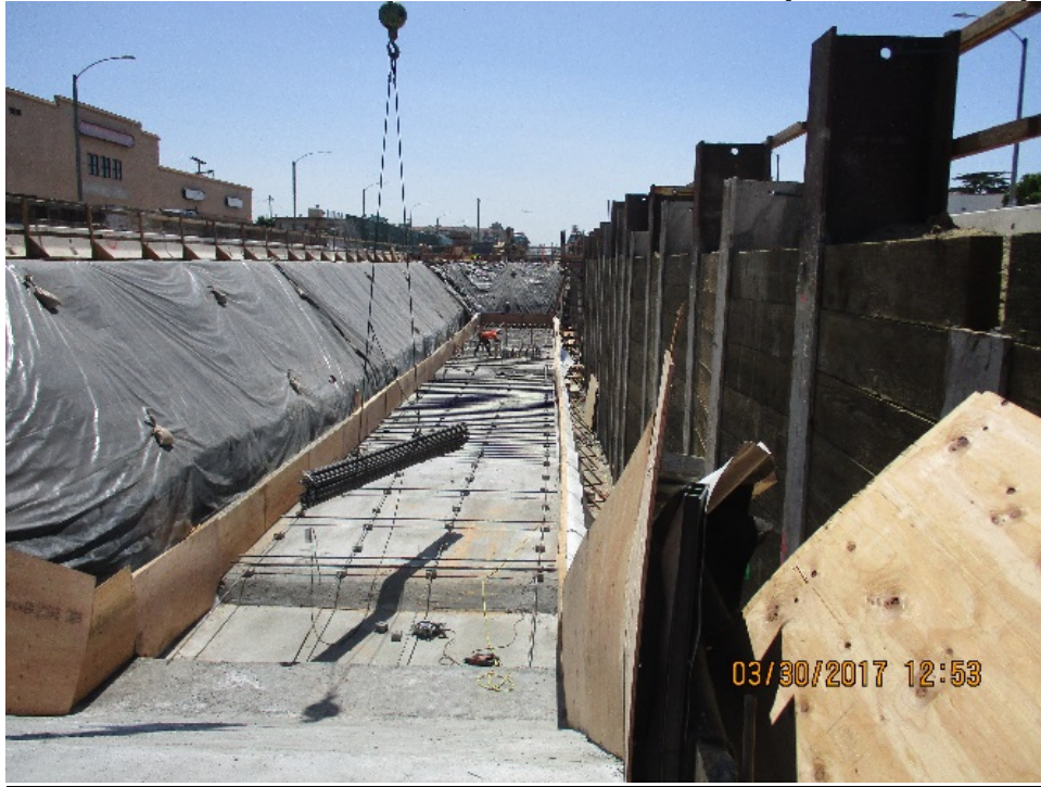
Hyde Park Station – Rebar installation for TC&C room invert slab.
