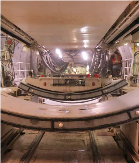
Concrete tunnel segments prepped for installation
