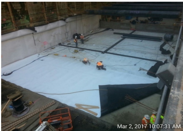
HDPE Installation at 2nd/Hope Station
