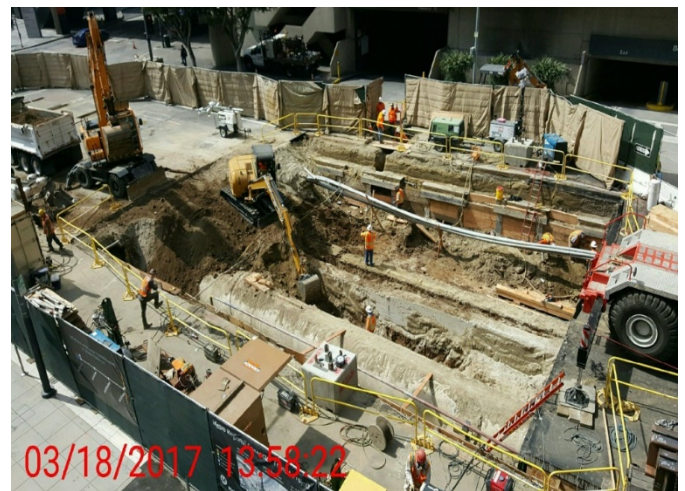
Excavation for deck beam installation over weekend closure
