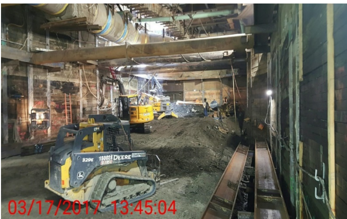
Excavation to bottom water level under Flower St. decking
