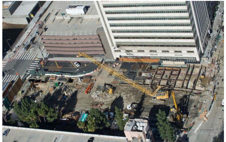
Decking progress on 2nd Street
