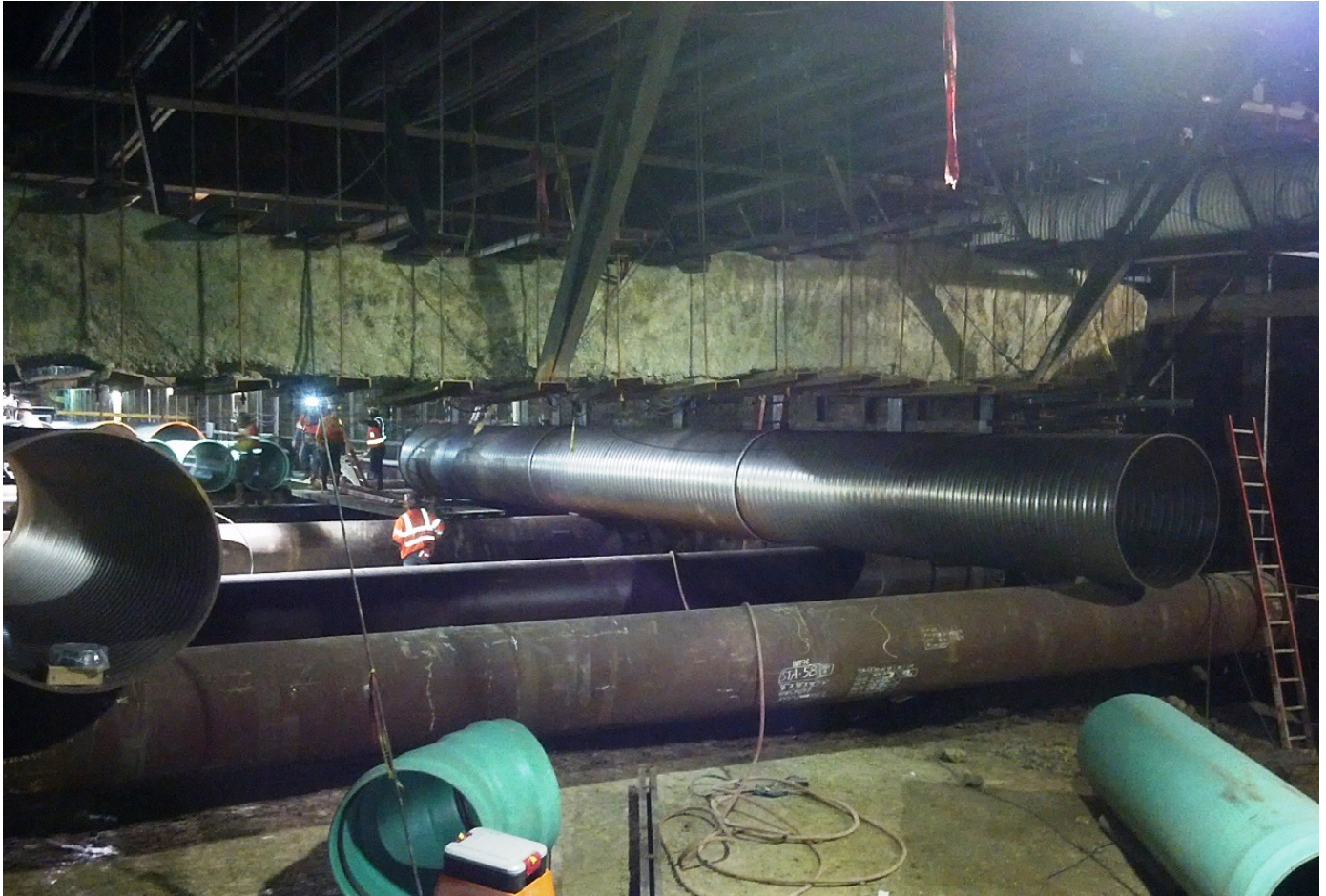
Connecting Ventilation System Pipes under the Wilshire/La Brea Station Deck
