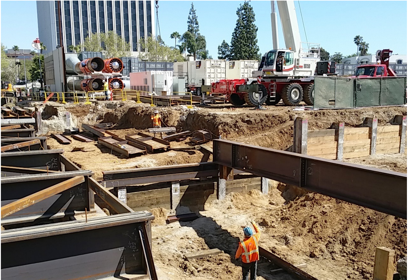
Placement of Deck Beam #63 in the Wilshire/Fairfax South Yard
