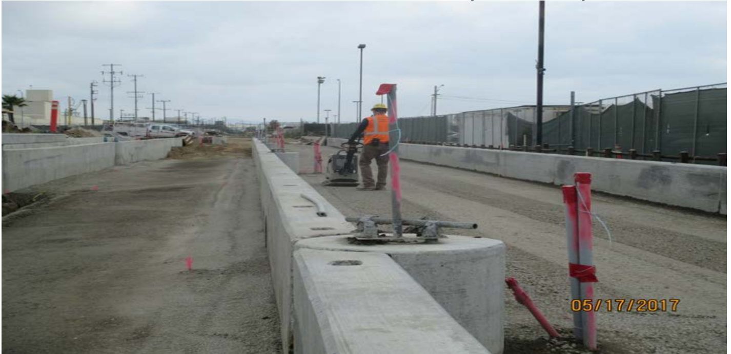
96 th STATION ACCOMODATIONS – Sub Ballast placement and compaction underway.
