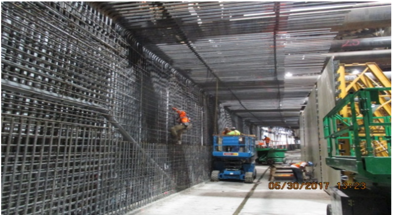
UG4 – Installation of rebar for walls adjacent to invert section I-26.
