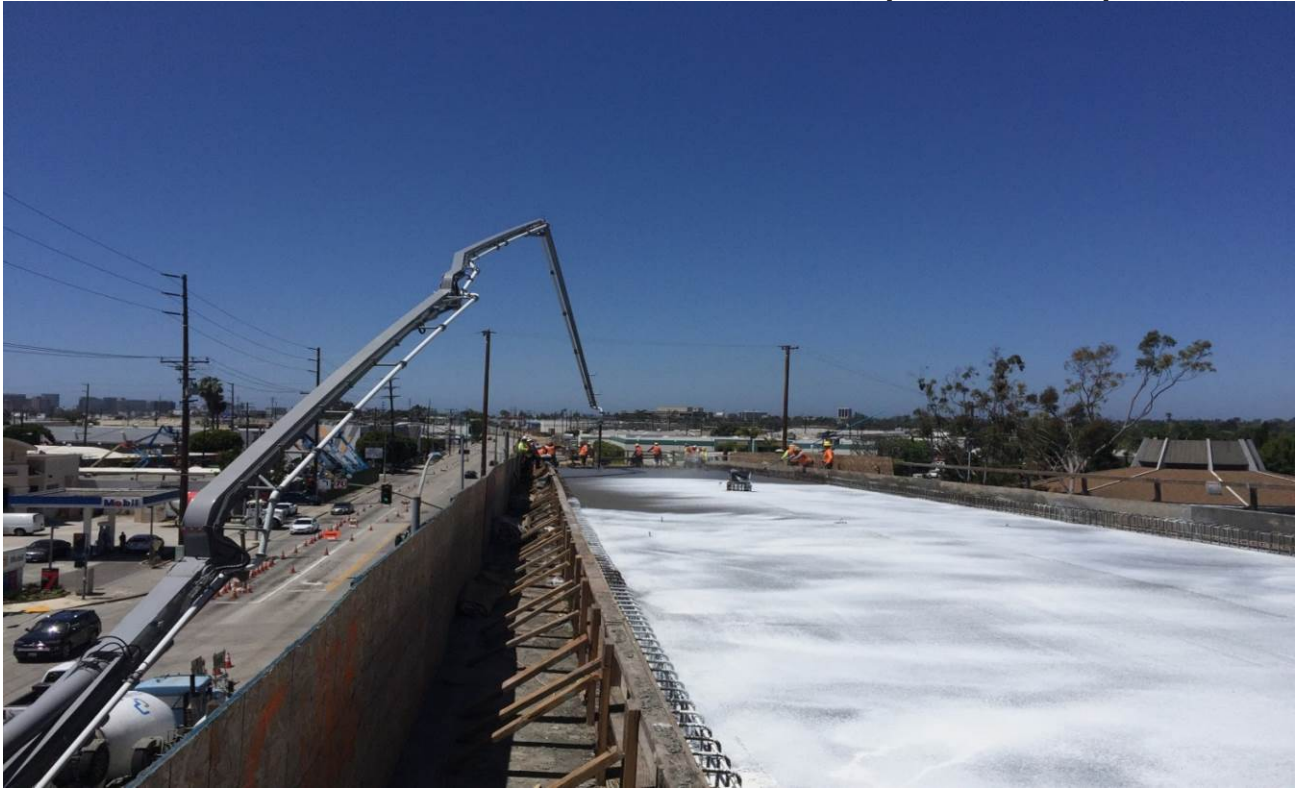
(AG-5) I-405 BRIDGE - I-405 Bridge concrete placement in progress.
