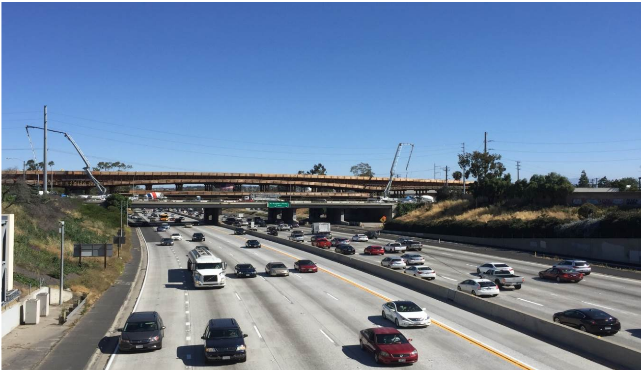
AG-5 I-405 BRIDGE - I-405 Bridge concrete placement in progress.
