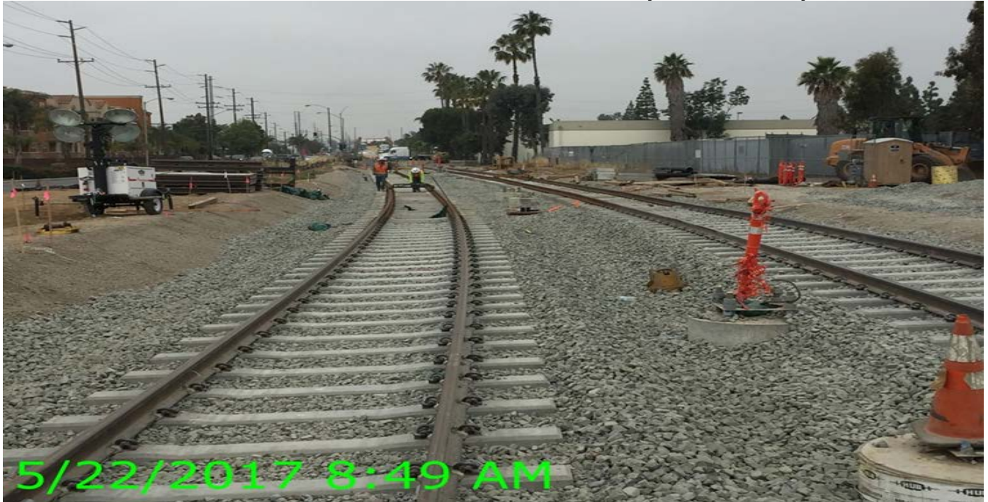
Ballasted track work between Oak and Cedar.
