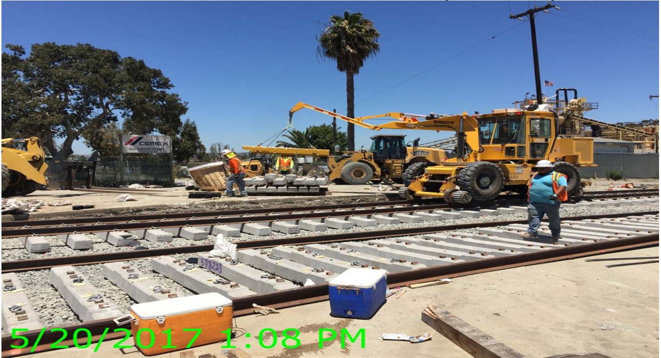
CEDAR GRADE CROSSING - Setting ties.
