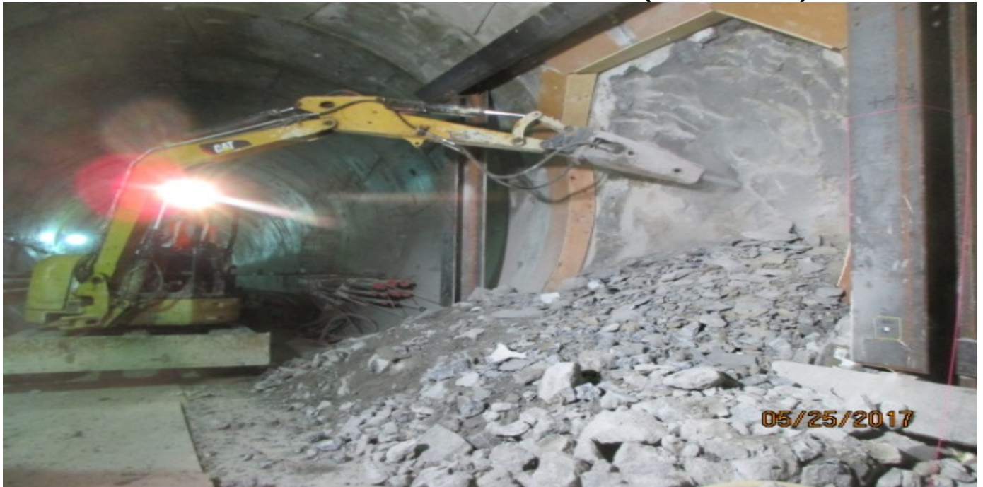
TUNNELING – Excavating into Cross Passage 5.
