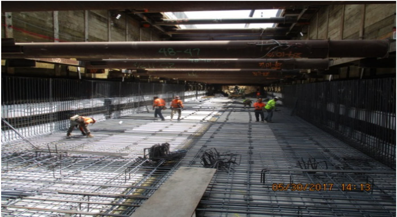
UG#3 Installation of invert rebar north of 63rd St.
