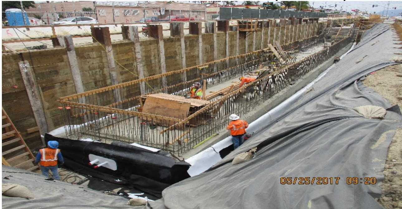
HYDE PARK STATION- Removing formwork from TC&C room invert placement.
