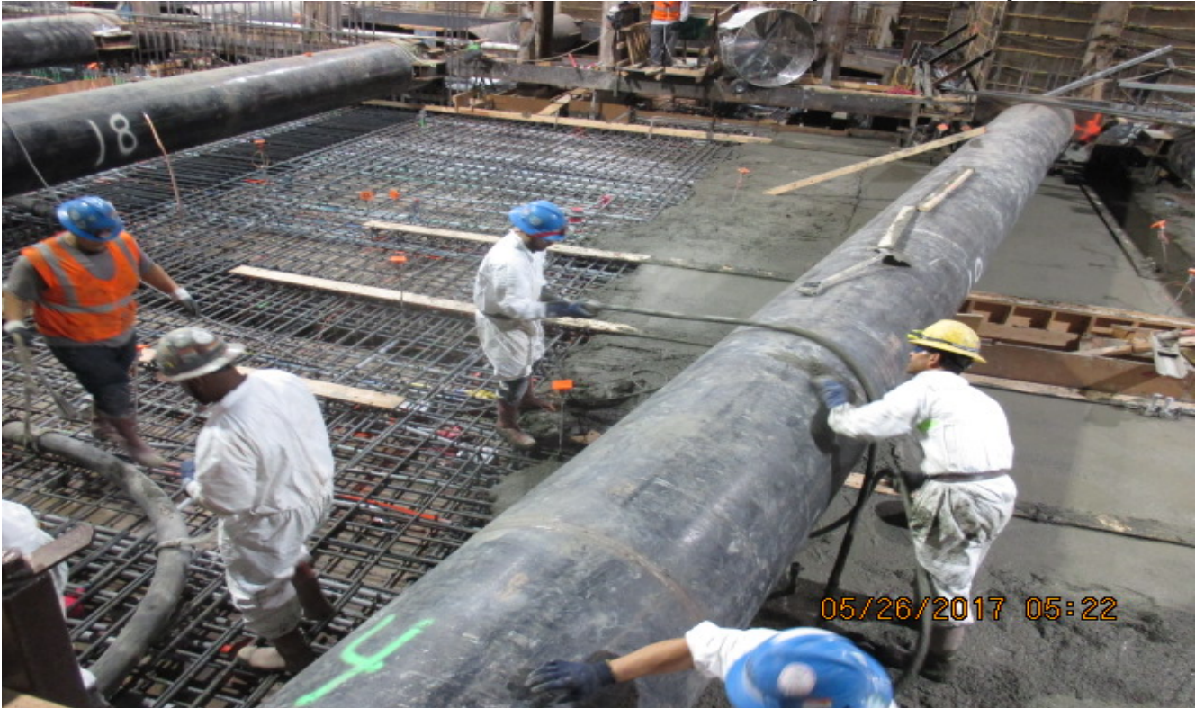
LEIMERT PARK STATION – Placement of concourse deck section C-2.
