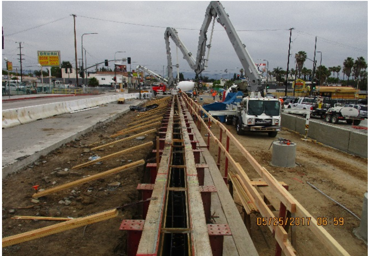
PARK MESA – Placement of ballast wall near 48th St.
