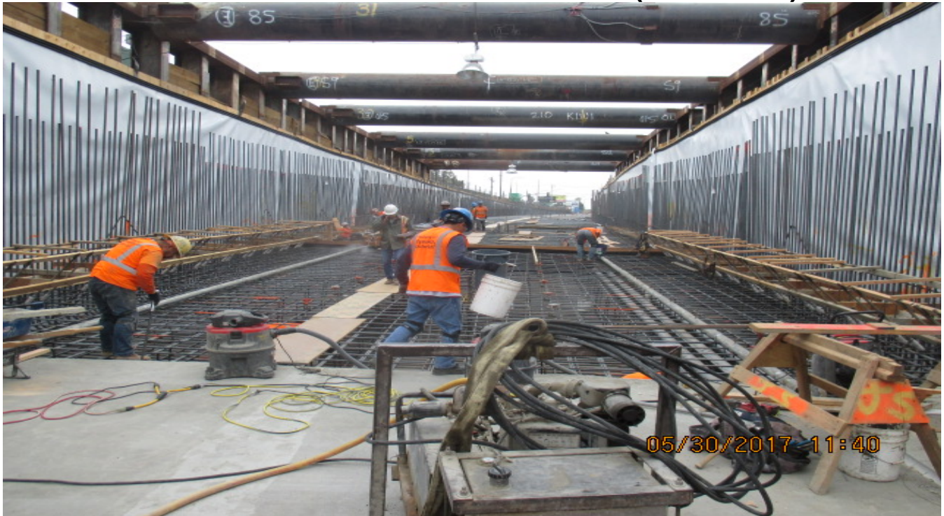
UG4 – Installation of rebar for invert section I-10.
