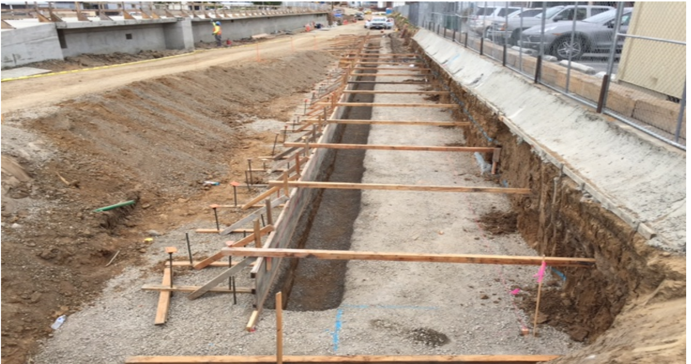
WESTCHESTER STATION – Forming of the South bound platform footing.
