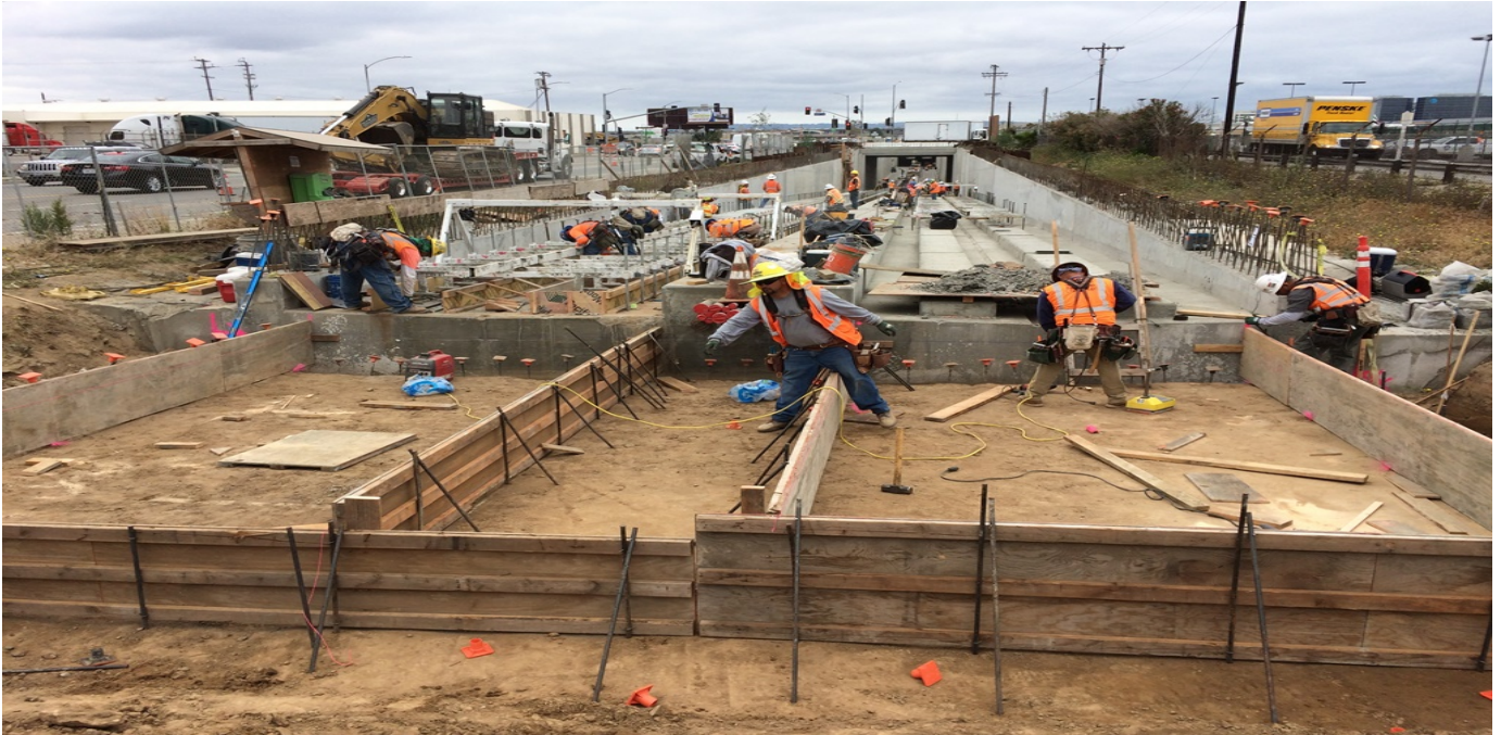
UG1 - Formwork installation for the northern approach slabs.
