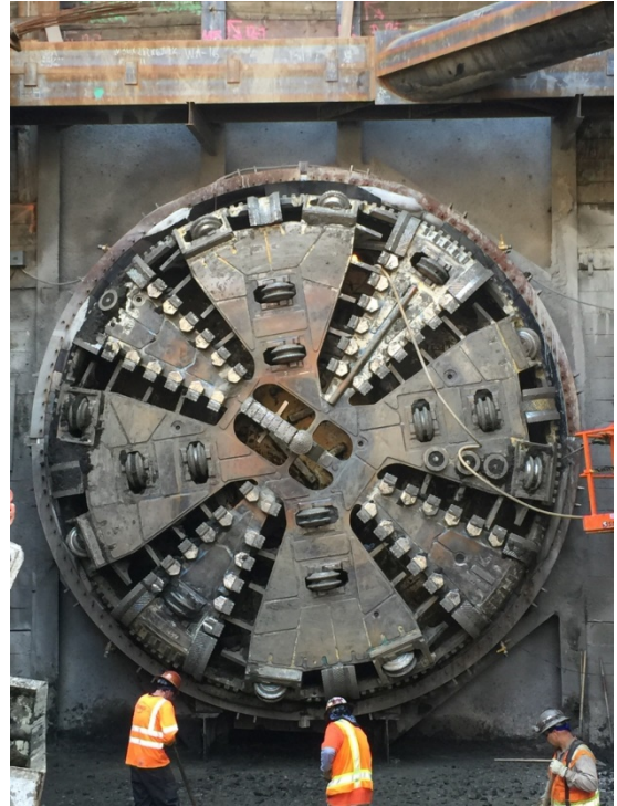
TBM cutter head cleaned
