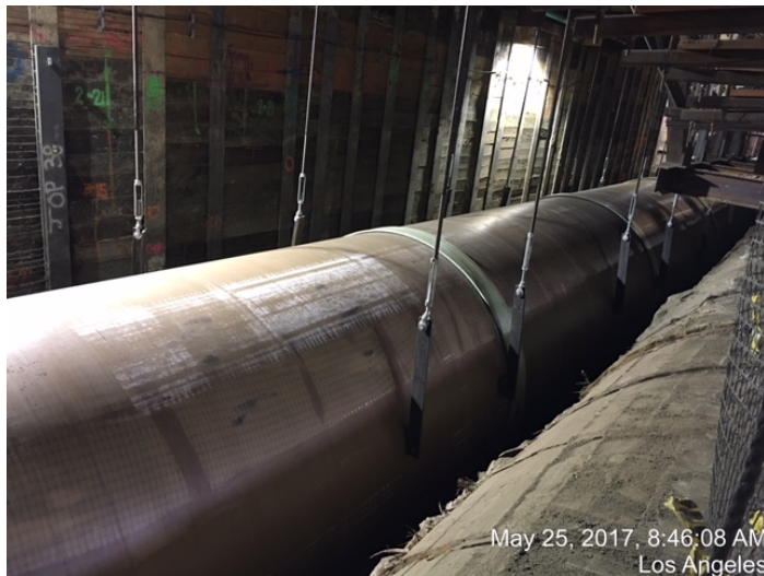
LA County storm drain (Hobas) pipe lowered for installation
