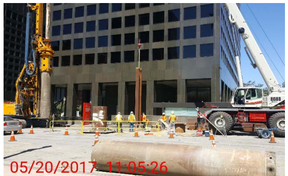
Pile installation in front of City National Plaza
