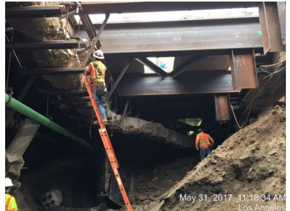
Utility hanging along Historic Broadway Station SOE
