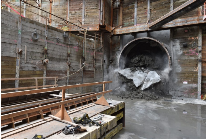
TBM breaking through at Grand Av Arts/Bunker Hill Station
