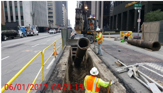
Pile trenching to remove newly abandoned 24" waterline
