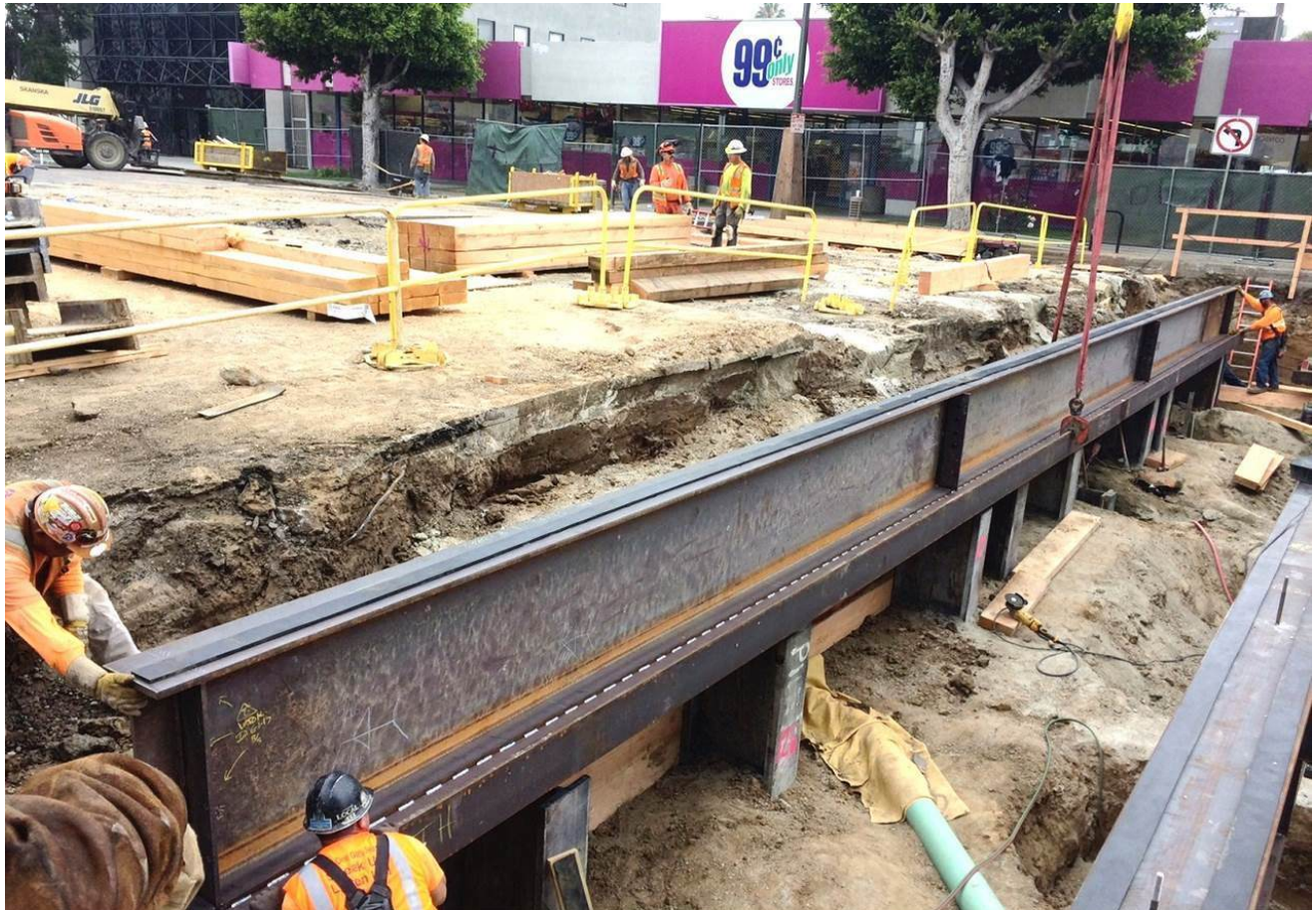
Wilshire/Fairfax Decking Operation in Progress
