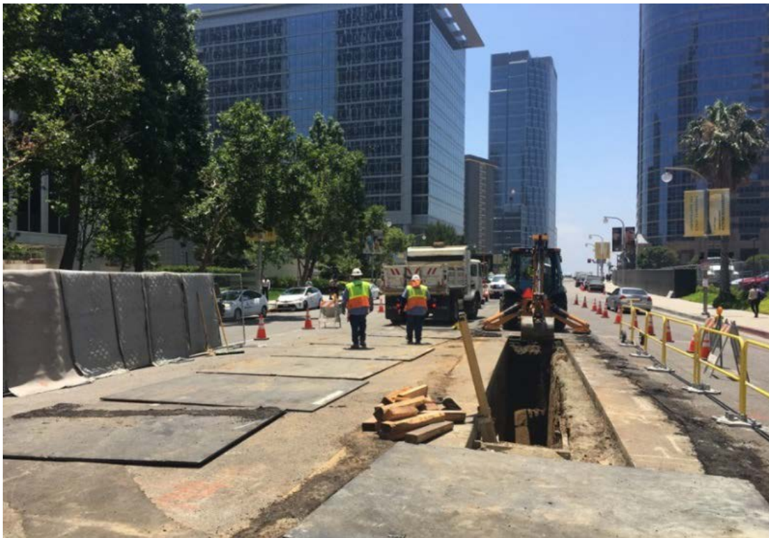
LADWP water relocation work in Century City
