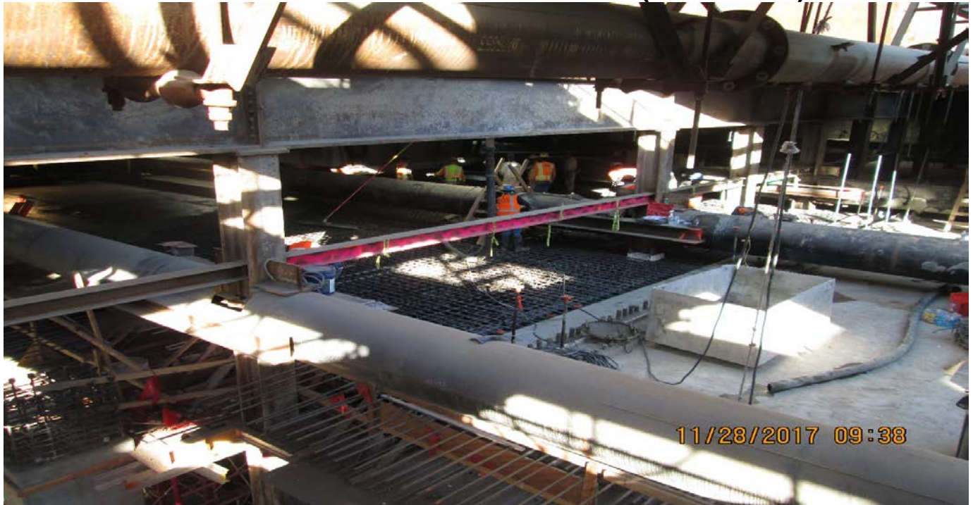
EXPOSITION/CRENSHAW STATION – Placement of concrete for roof deck section K-7.
