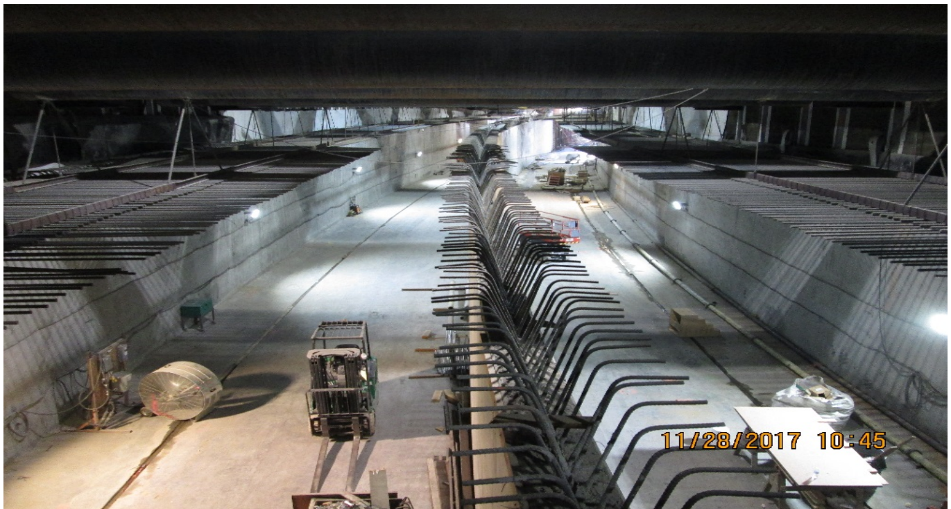
UG4 – East, center, and west wall progress along the Guideway.
