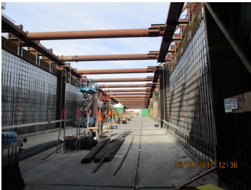
UG3 – Rebar installation along walls north of 60 th St.
