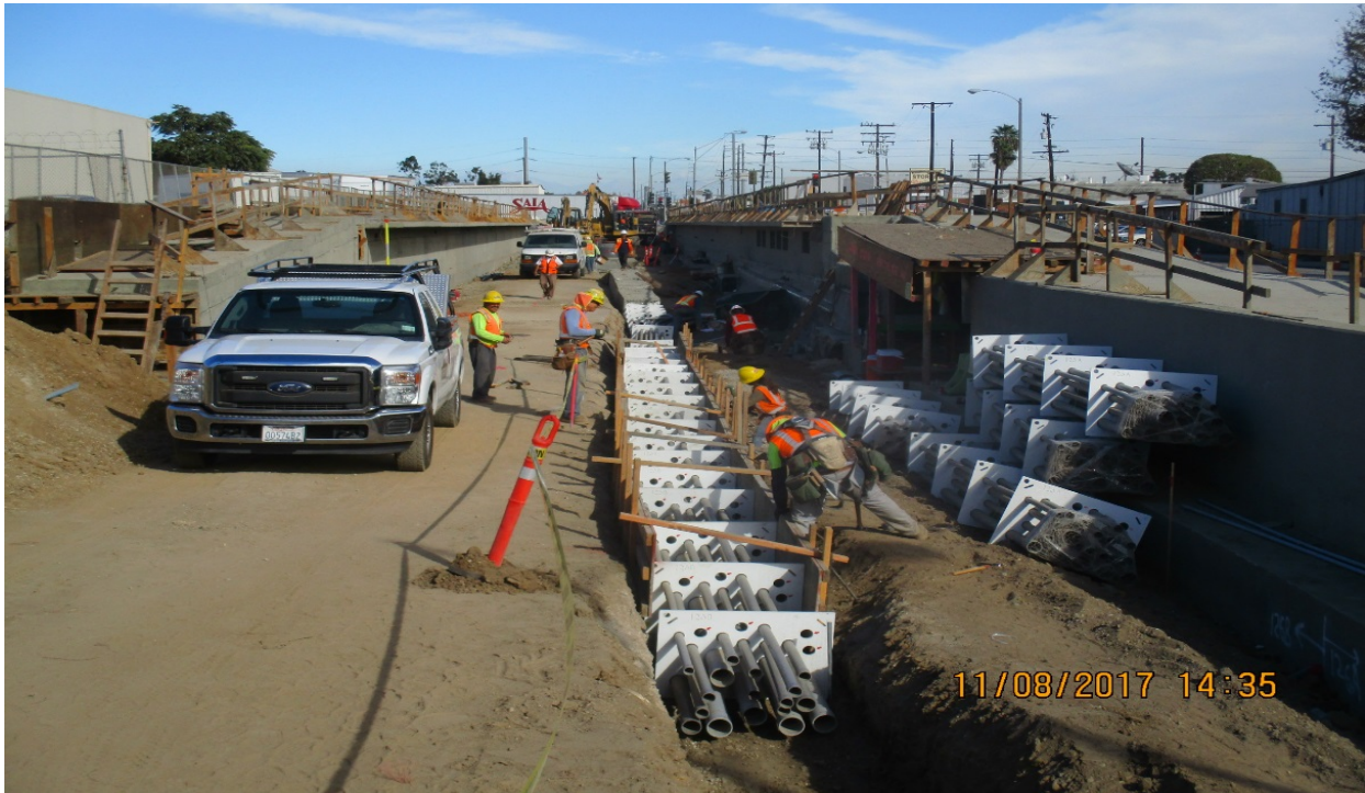
HINDRY STATION - Forming for electrical duct bank between platforms.
