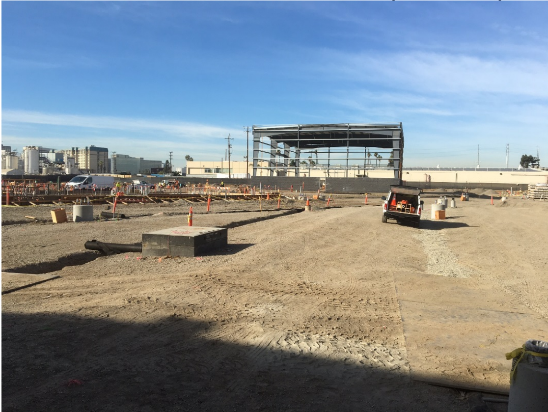
SOUTHWESTERN YARD MAINTENANCE FACILITY – Material storage building construction.
