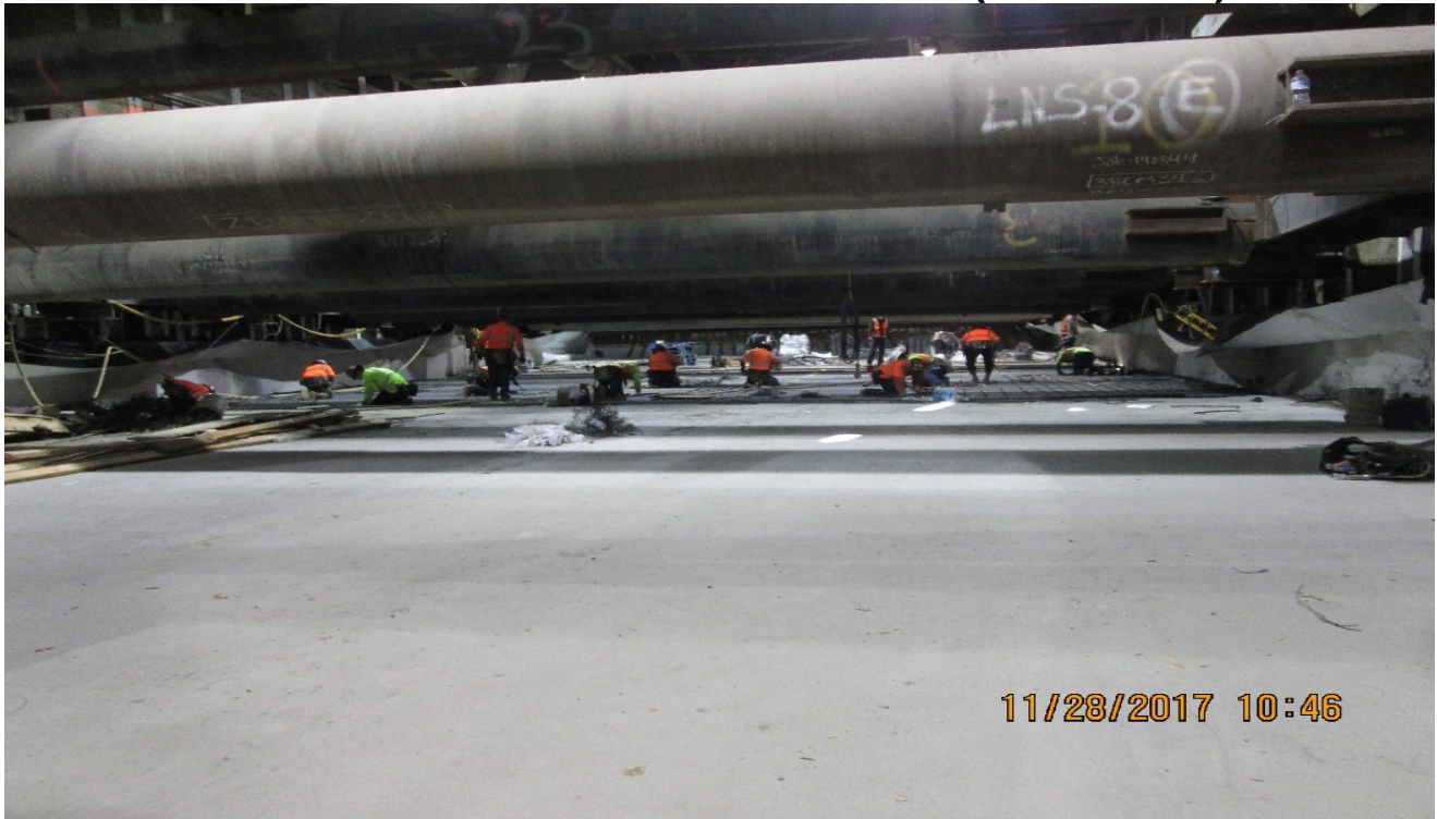
UG4 – Installing rebar for roof section R-27.
