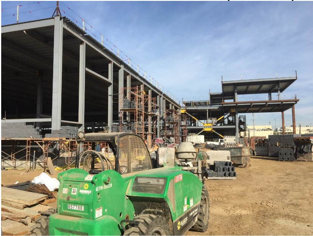
SOUTHWESTERN YARD MAINTENANCE FACILITY – Main shop construction.
