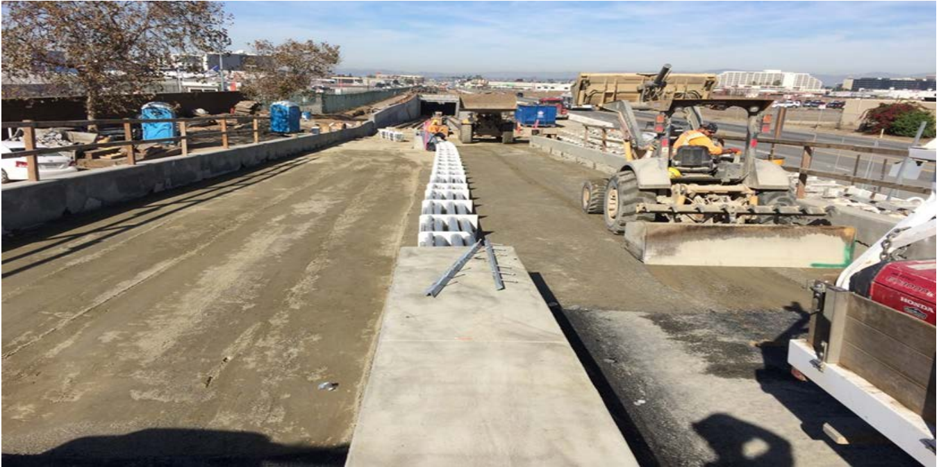
MSE 29L&R – Asphalt cap subgrade fine grading from STA 30+50 to 32+09.
