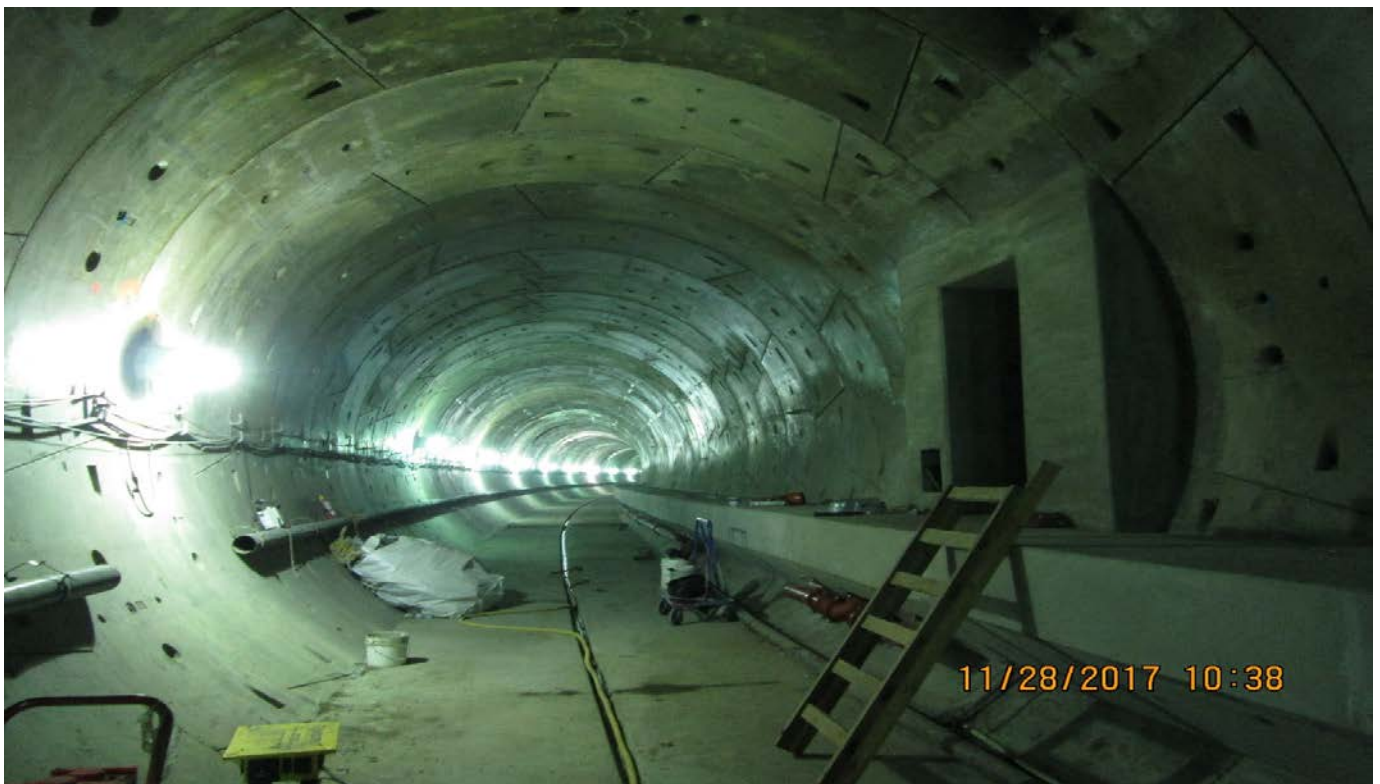
TUNNELING – SB Tunnel at entrance to Cross Passage 5.
