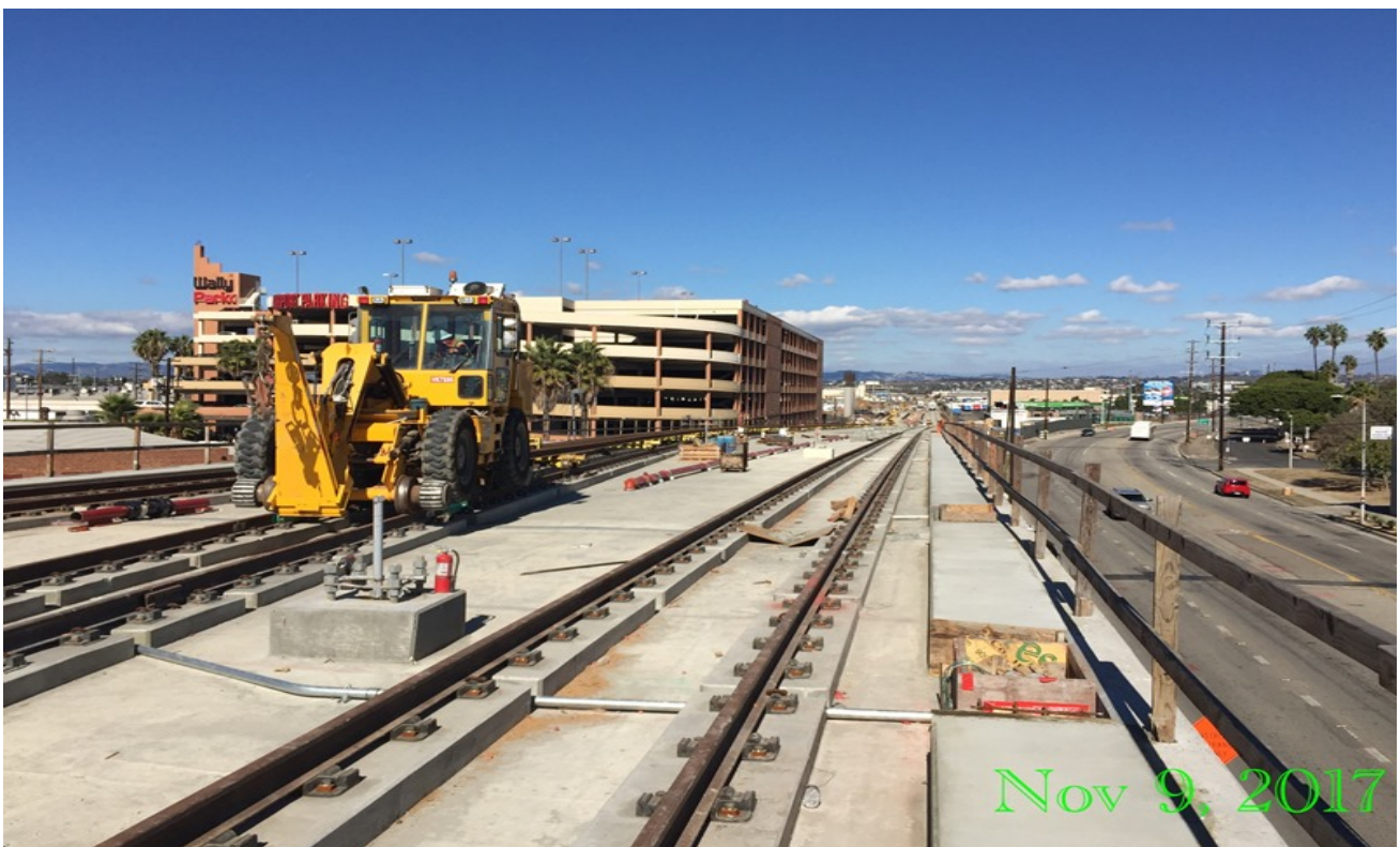
MSE 75L&R: Crew moving 115 # R.E running rail on track-3 SB.
