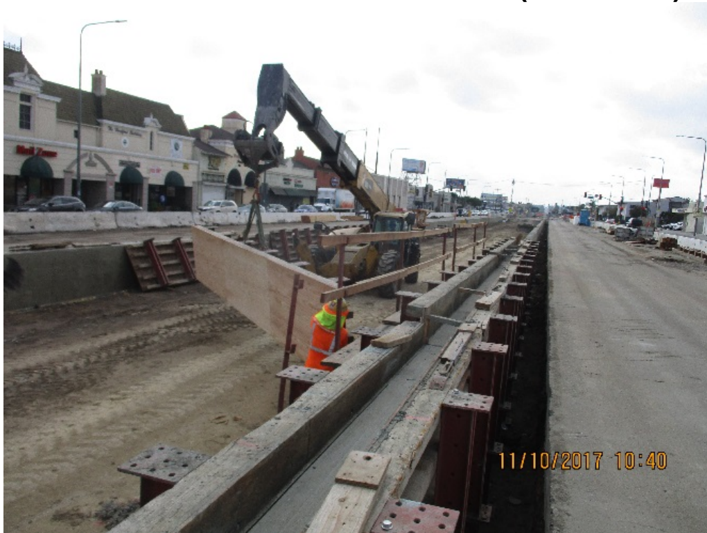
PARK MESA – Removing ballast wall formwork between 54 th and 57 th St.
