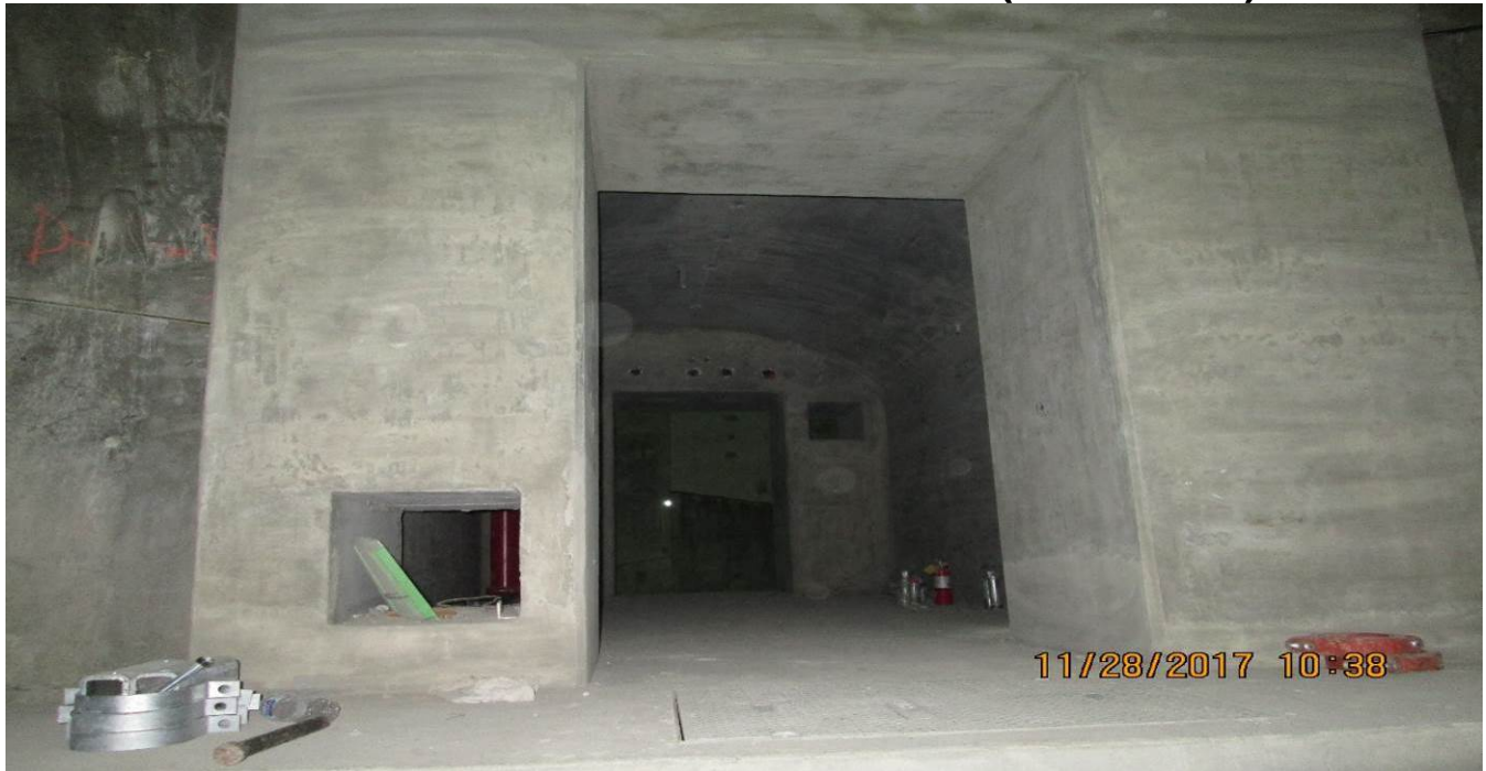
TUNNELING – Looking into CP-5 from the SB Tunnel.
