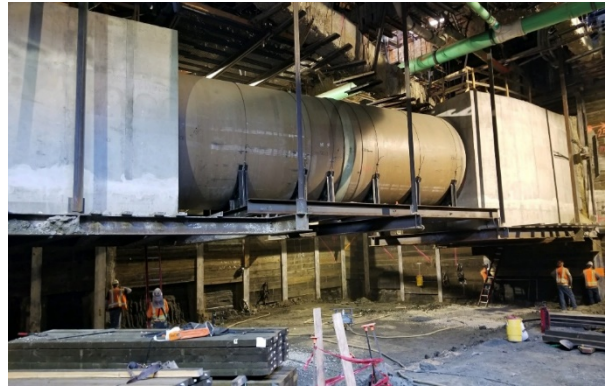
Bracing of storm drain pipe near Spring Street
