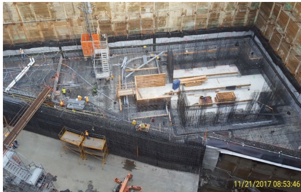
North concourse rebar and electrical installation
