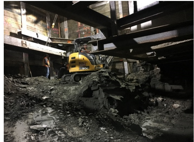
Excavation under Flower Street
