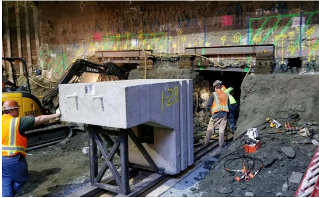
Underpinning activities underway
