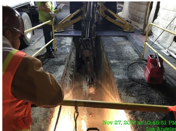
Excavation for Mainline B
