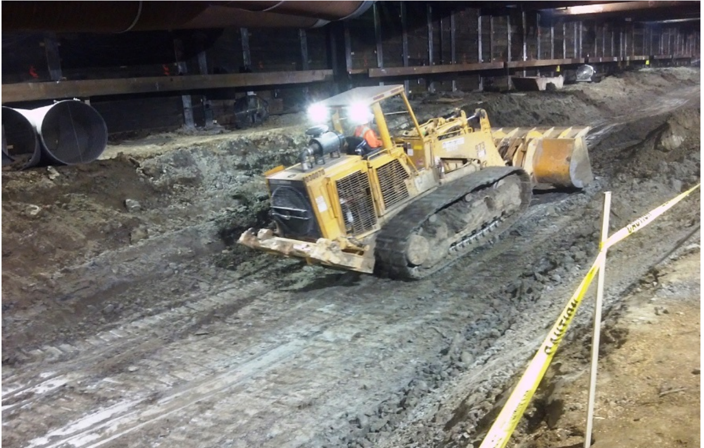
Wilshire/Western Station Excavation
