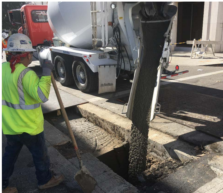
SCE Utility Relocation Work in Beverly Hills
