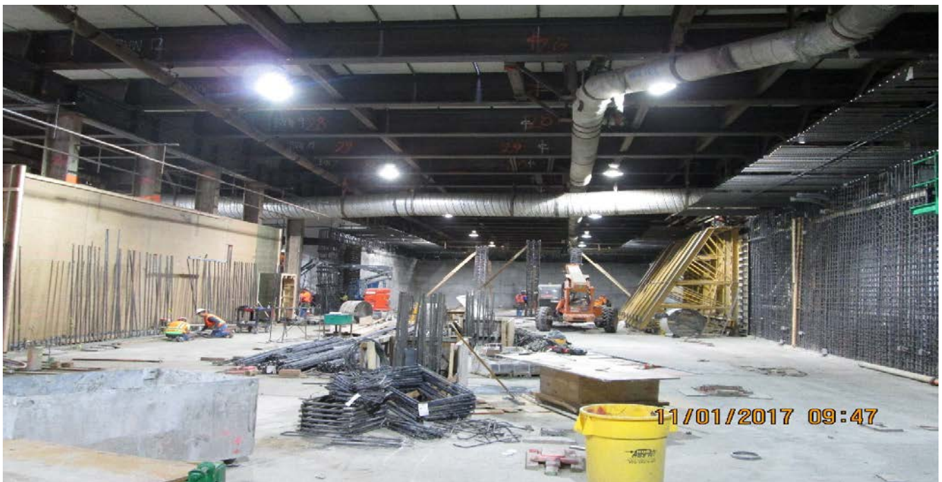
LEIMERT PARK STATION - Installing formwork and rebar along south concourse level walls.
