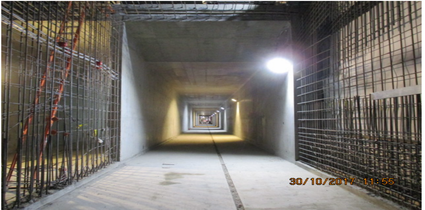
UG#3 - SB tunnel section south of 60th St.
