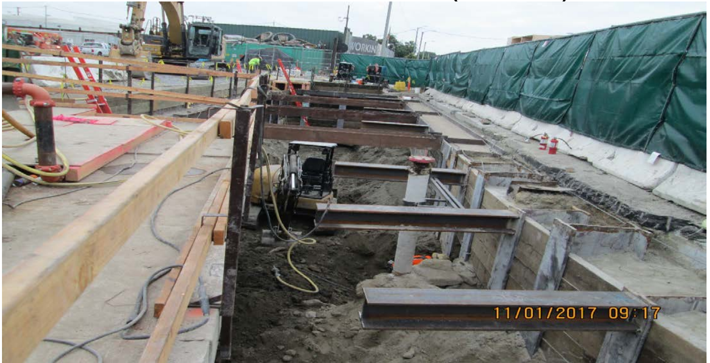
EXPOSITION/CRENSHAW STATION – Excavating at side structure “S”.
