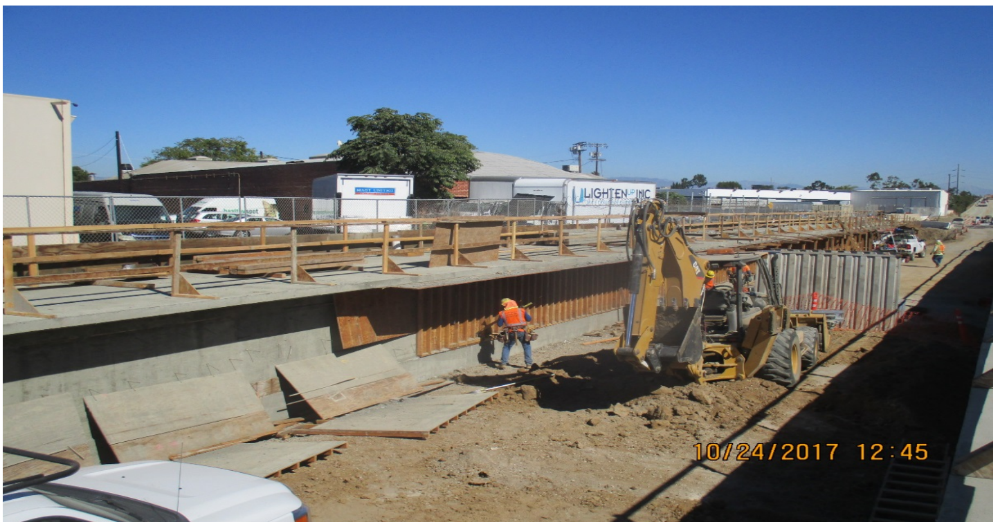
WESTCHESTER STATION – SB platform stripping of southern shear walls.
