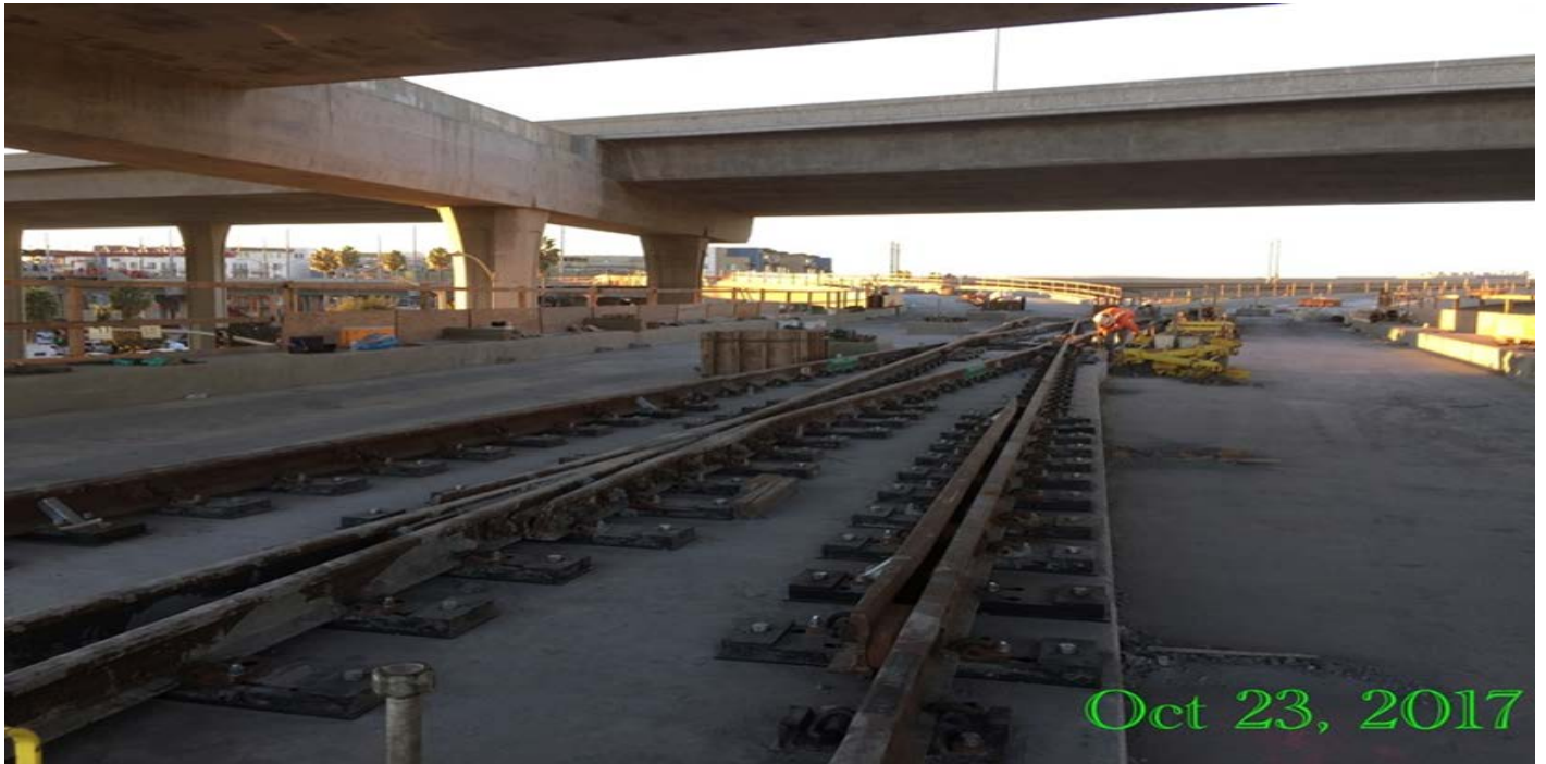
GREENLINE UNDERPASS – Crew installing slobber plate, rail fasteners and rail restraining rail at movable switches.
