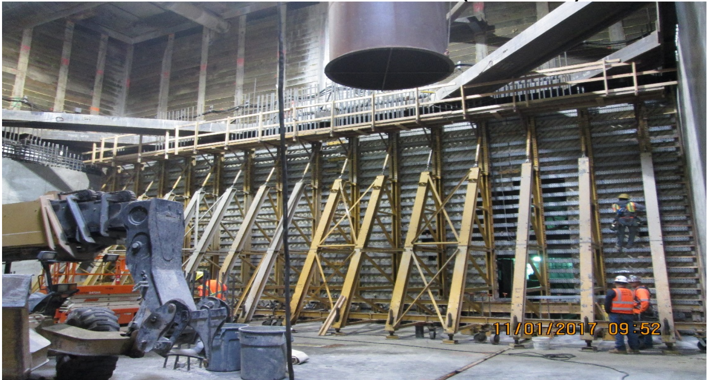
LEIMERT PARK STATION – Installing rebar for lower walls in the north hammerhead.
