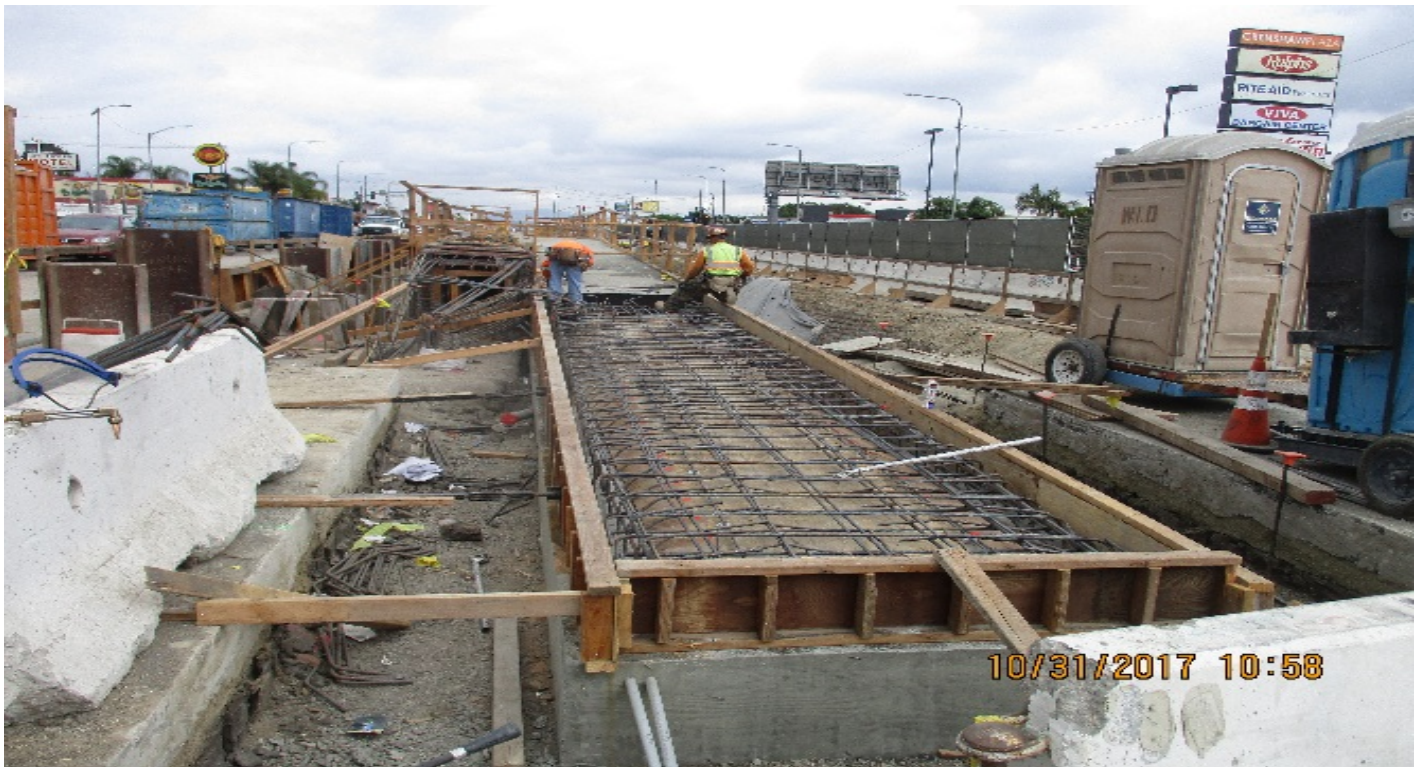
HYDE PARK STATION - Installation of rebar at station ramp.
