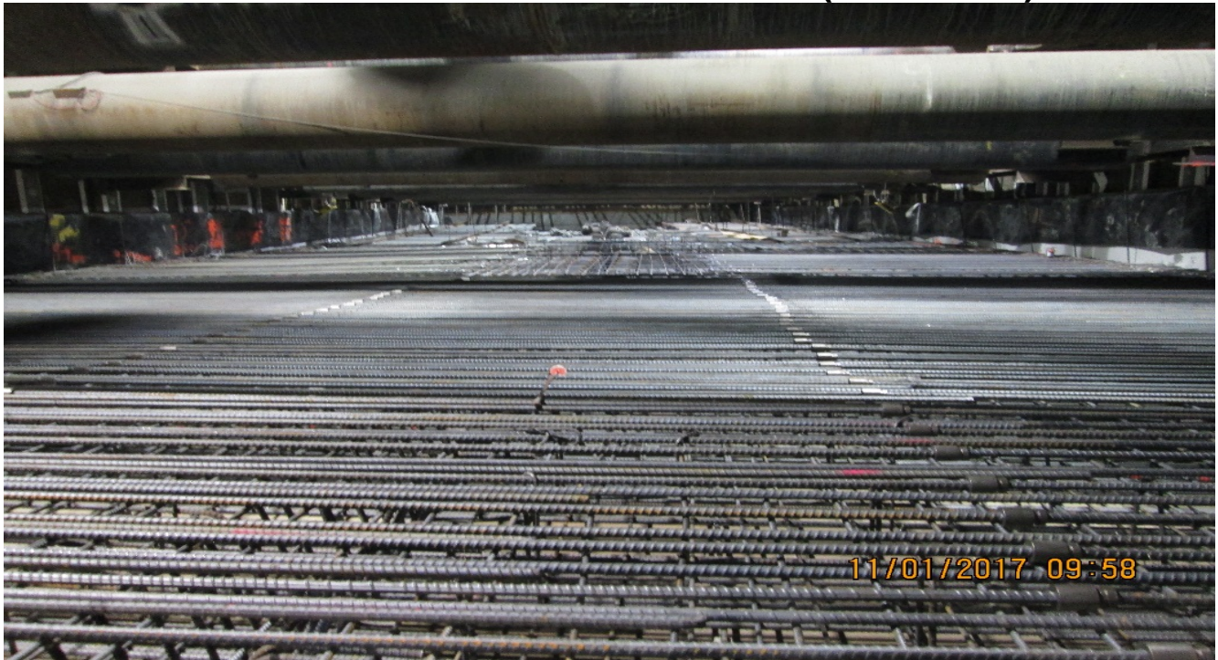
UG4 – Installing rebar for roof sections R-28 thru R-25, south of Vernon portal.
