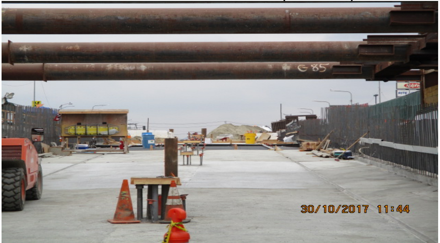
UG#3 - Approach slab at the north portal.
