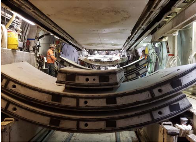
Concrete ring preparation for placement inside TBM
