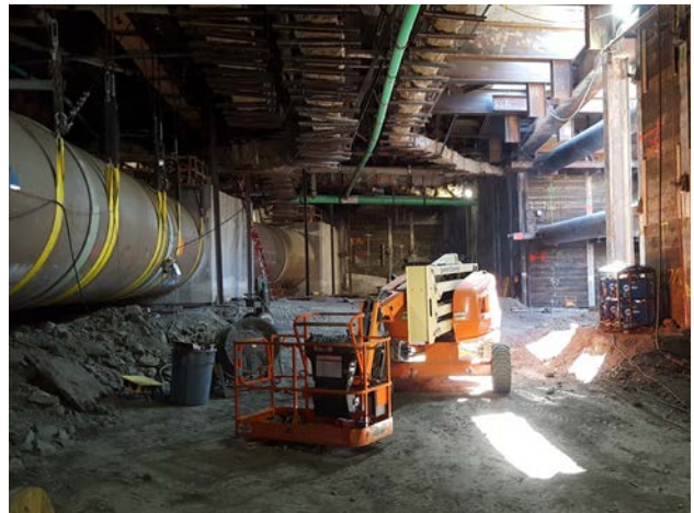
Hobas pipe with structure bracing
