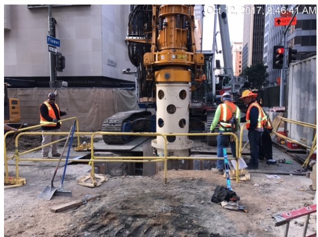
Pile installation on east side at 6th/Flower
