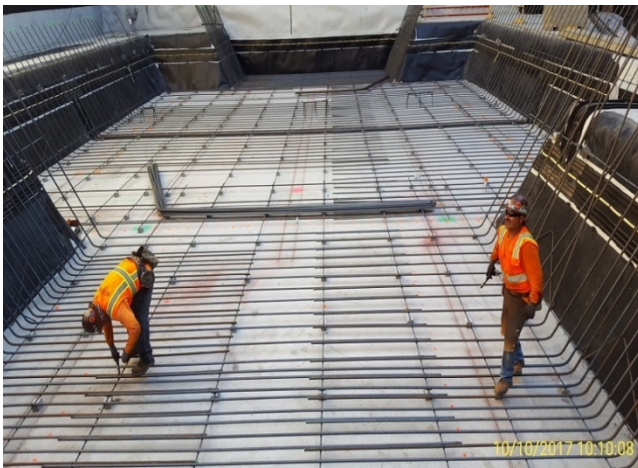
Rebar placement on Concourse Level of Grand Av Art/Bunker Hill Station
