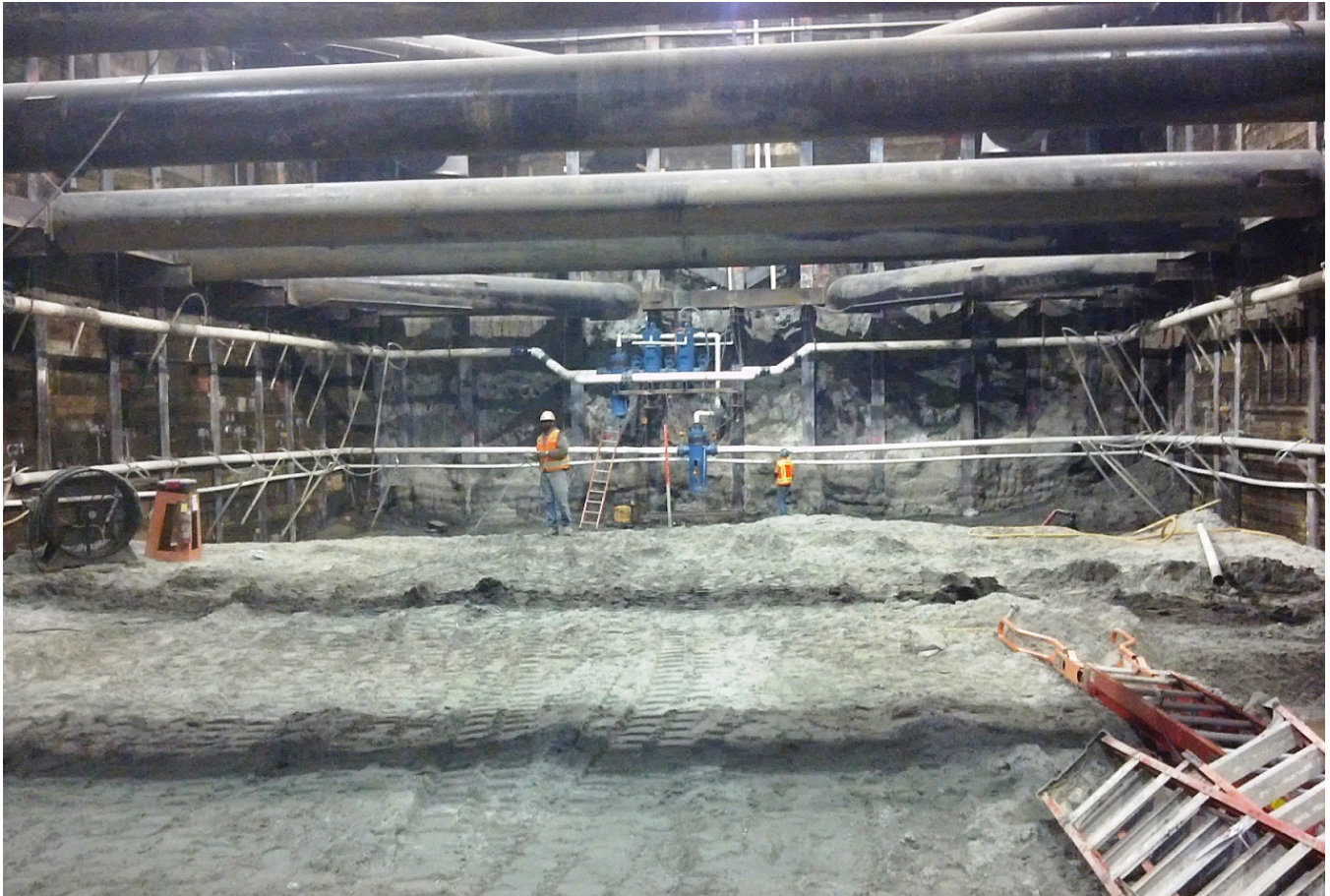
Under Deck Excavation at Wilshire/La Brea Station
