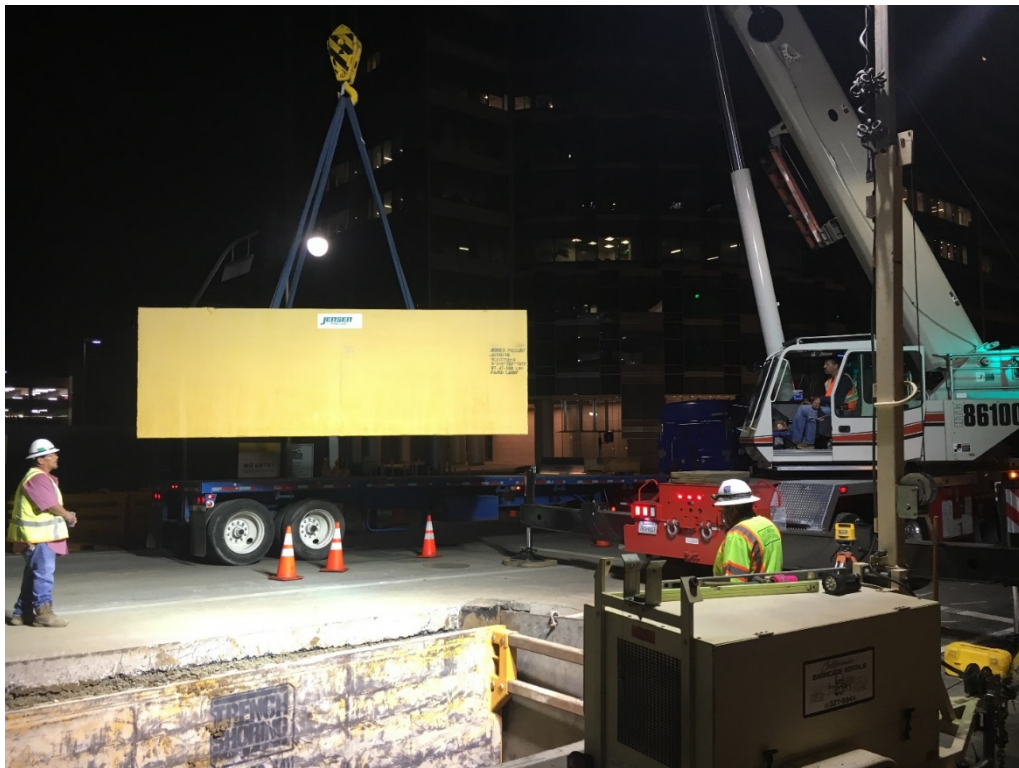
LADWP Power Vault Installation in Century City
