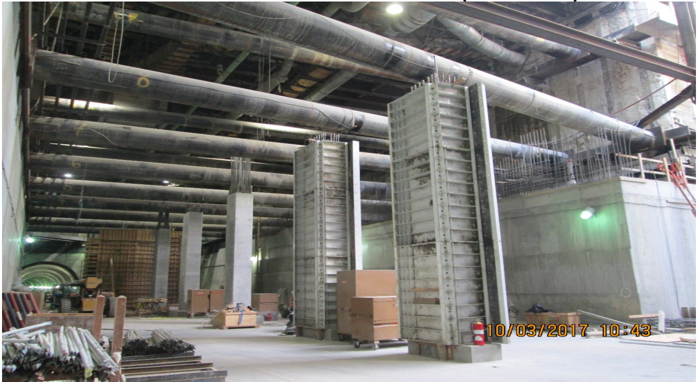
MARTIN LUTHER KING JR. STATION Previously placed invert level columns C6.
