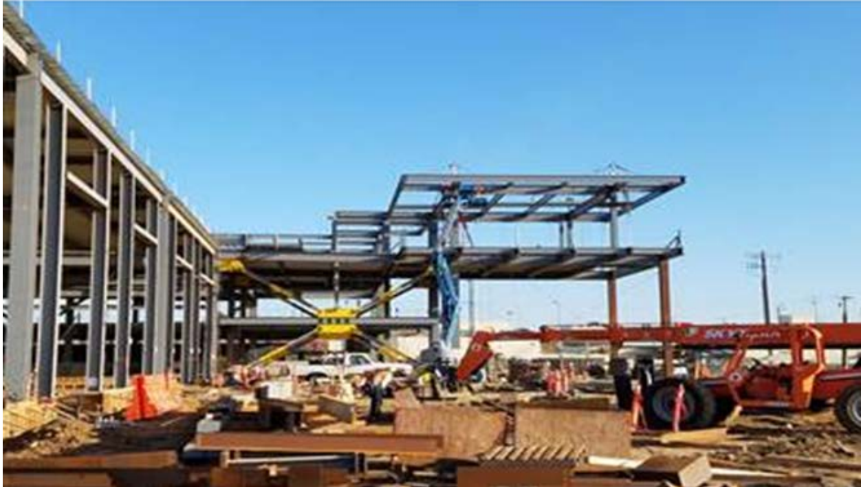
Southwestern Yard - Main shop building with control tower.
