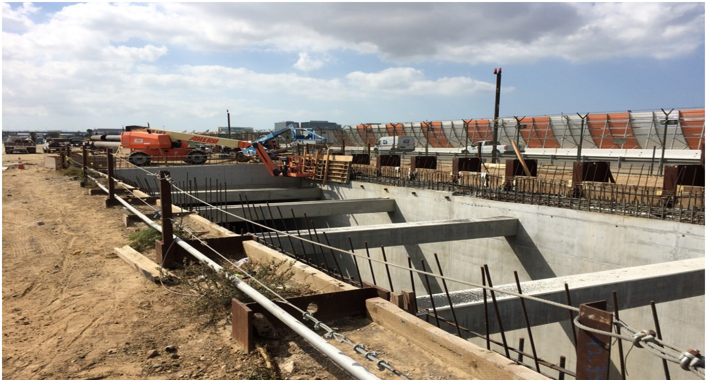
UG#1 - Concrete barrier formwork installation on the west U-Wall STA 50+00 to 50+38.
