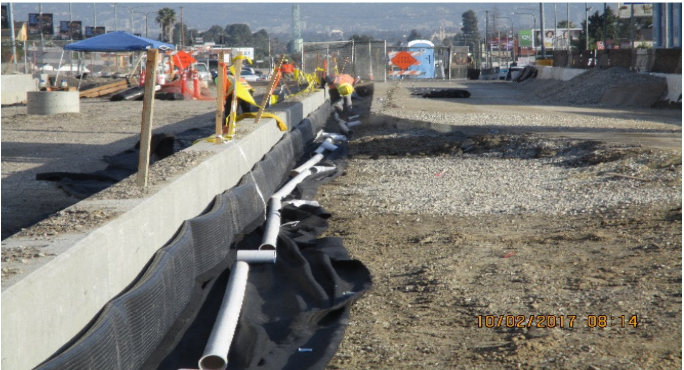
PARK MESA – Installing ballast wall drain between 52nd and 54th St.
