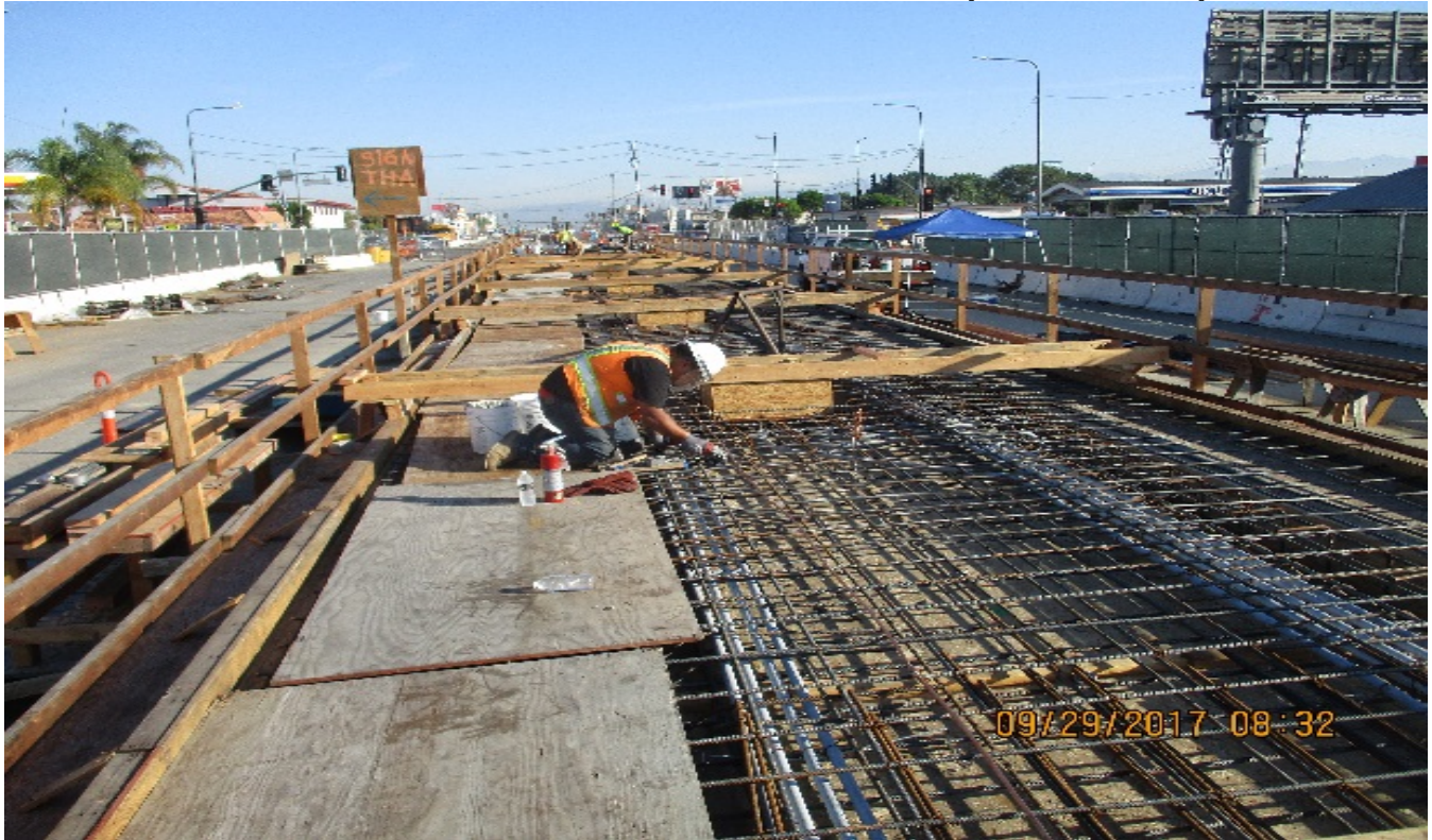
HYDE PARK STATION- Installation of electrical components in the platform deck.
