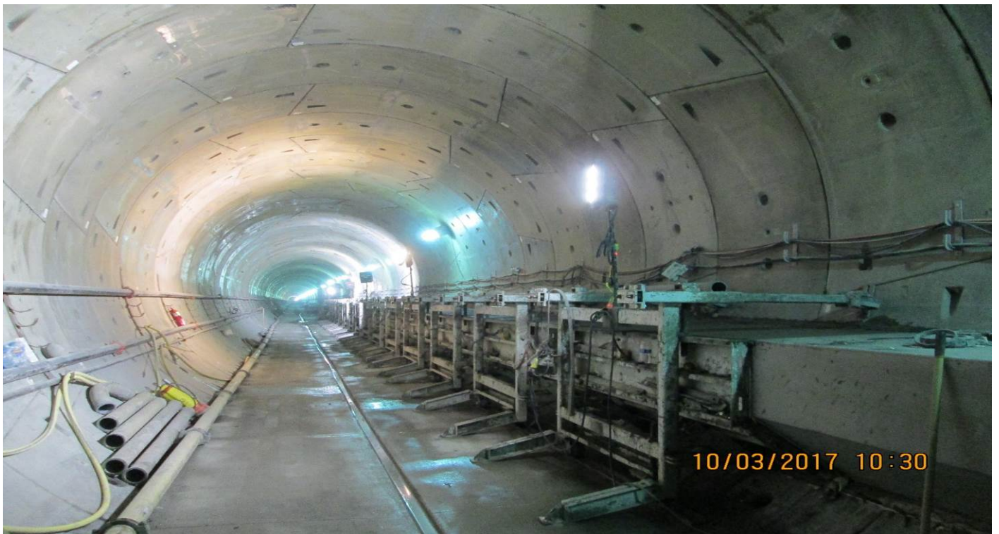
TUNNELING – Placement of NB Tunnel Walkway section 13a.
