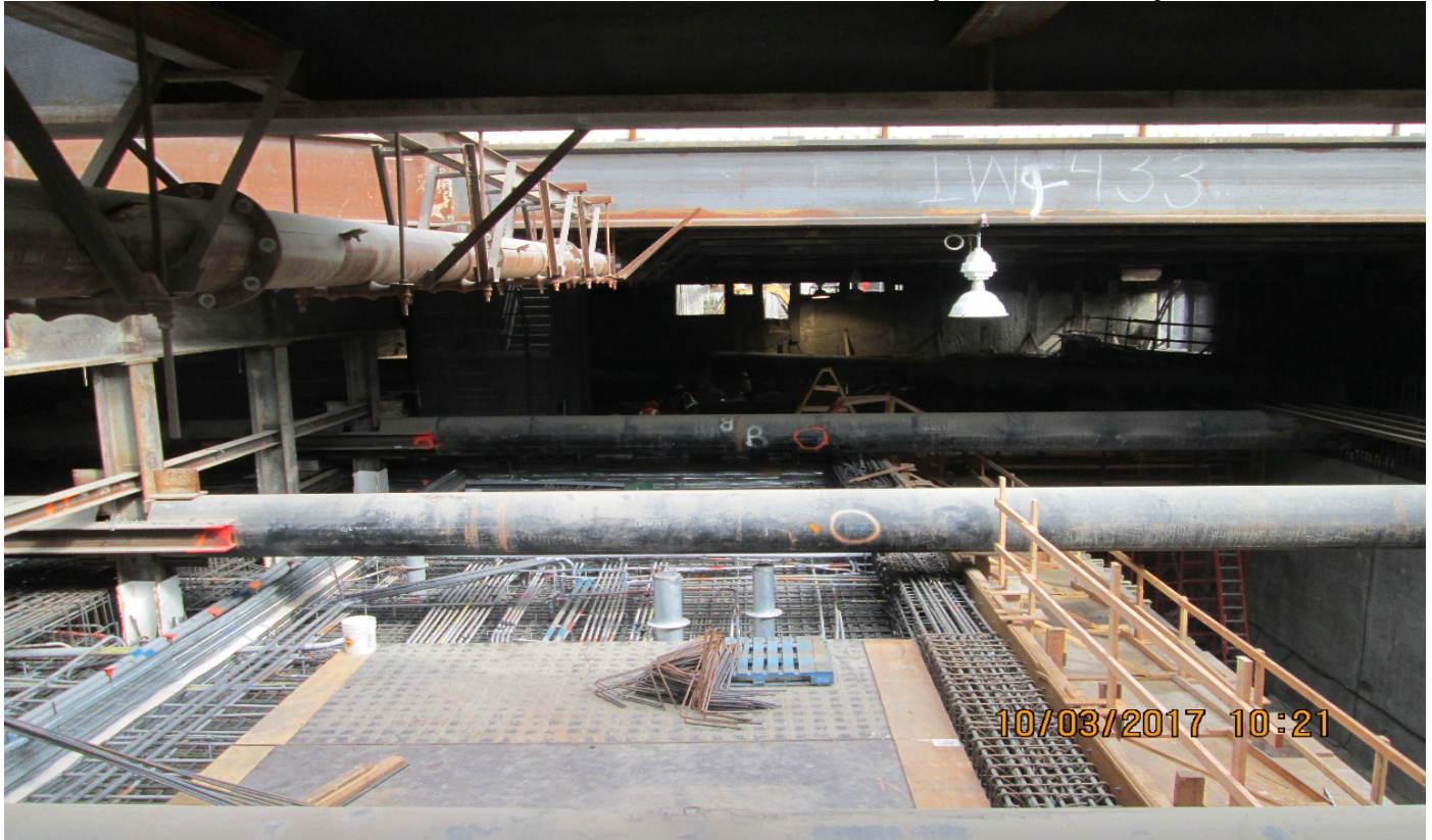
EXPOSITION/CRENSHAW STATION – Installing rebar for Roof Slab Phase 1.
