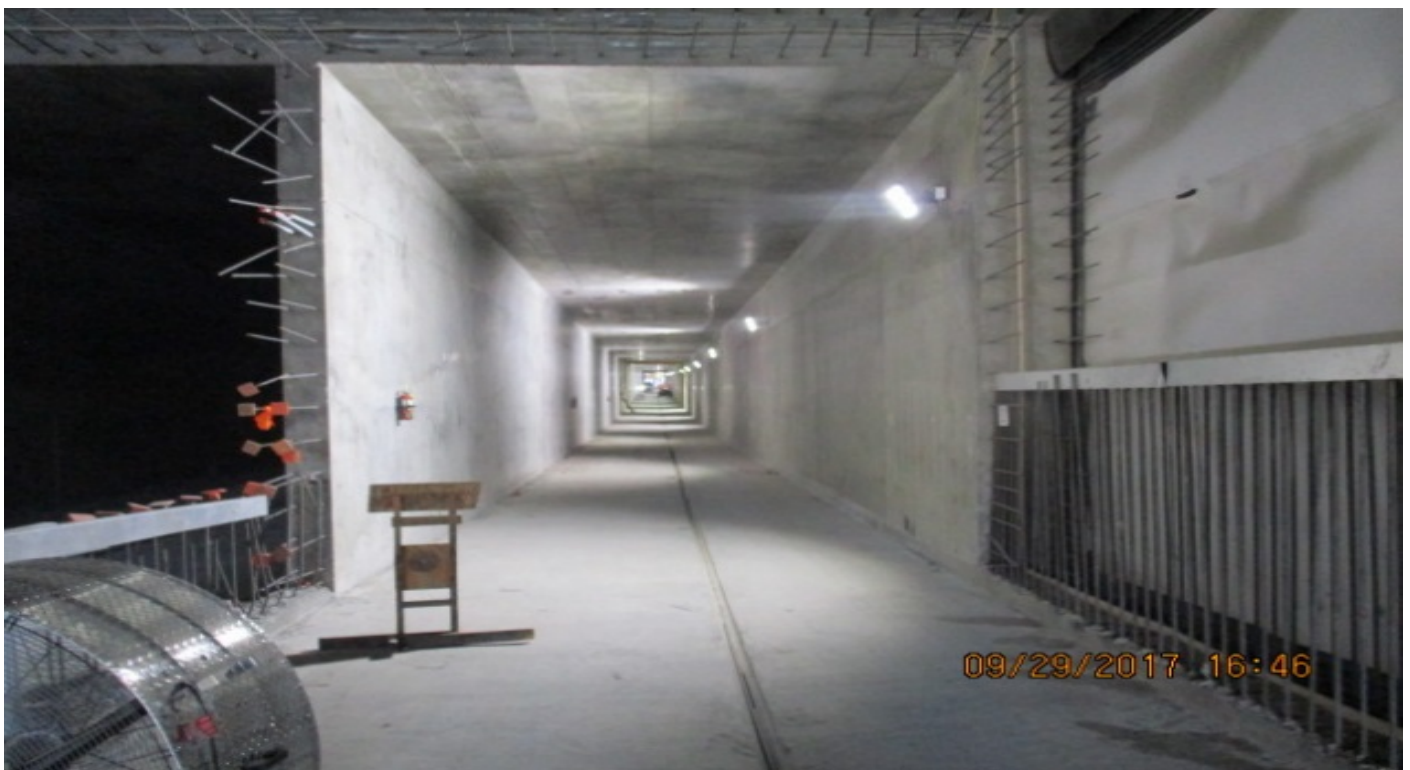
UG#3 - SB tunnel section south of 60th St.
