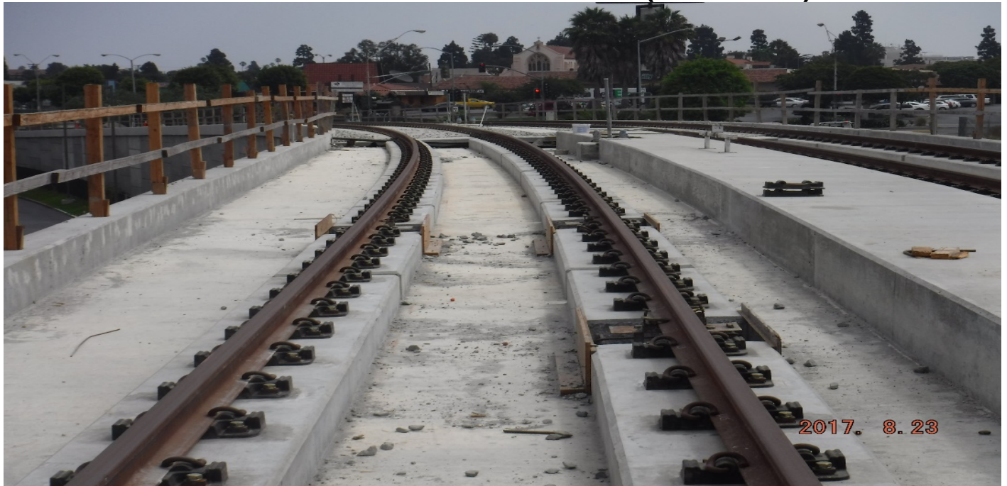
(AG-6) LA BREA BRIDGE - Bridge superstructure complete, DF track plinth in-place.
