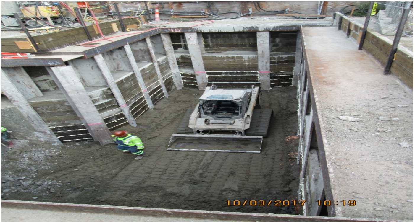
EXPOSITION/CRENSHAW STATION – Excavating at side structure “Q”.
