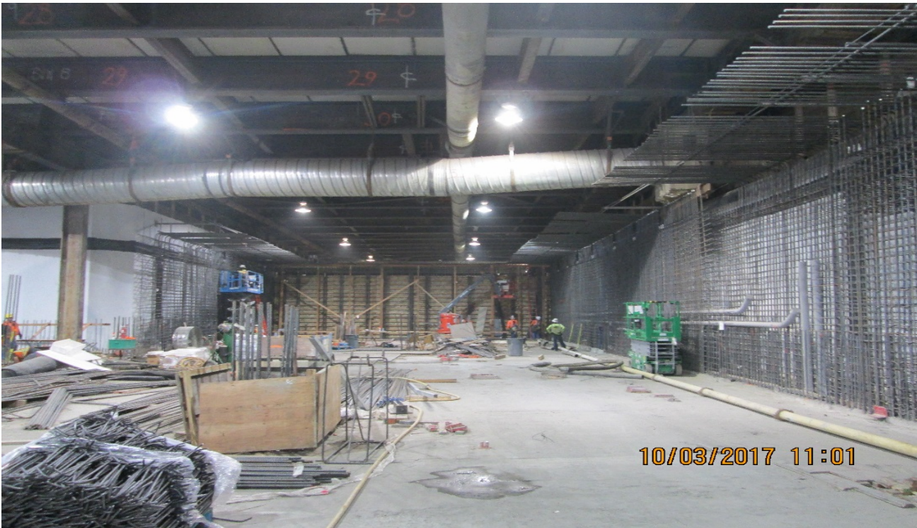
LEIMERT PARK STATION - Installing rebar along south concourse level walls.
