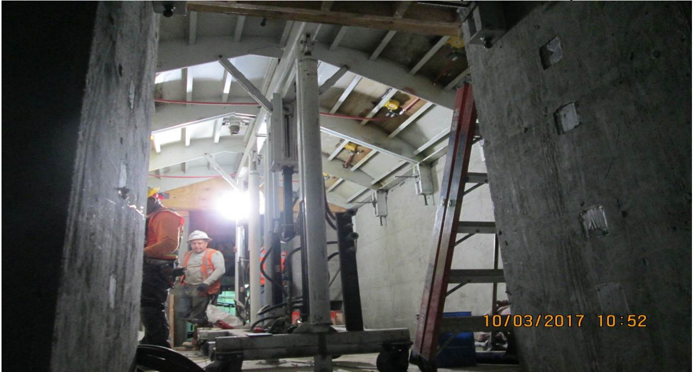
TUNNELING – Erecting arch section formwork at CP-5.
