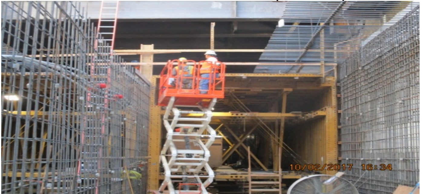
UG#3 - Installation of formwork for traveler section 47.
