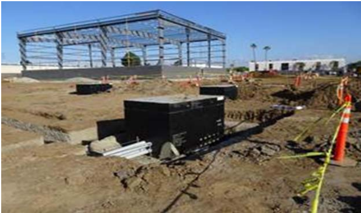
Southwestern Yard - Underground ductbank, vaults and material storage building.
