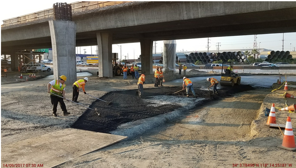
Pave Vignes ramps for opening.
