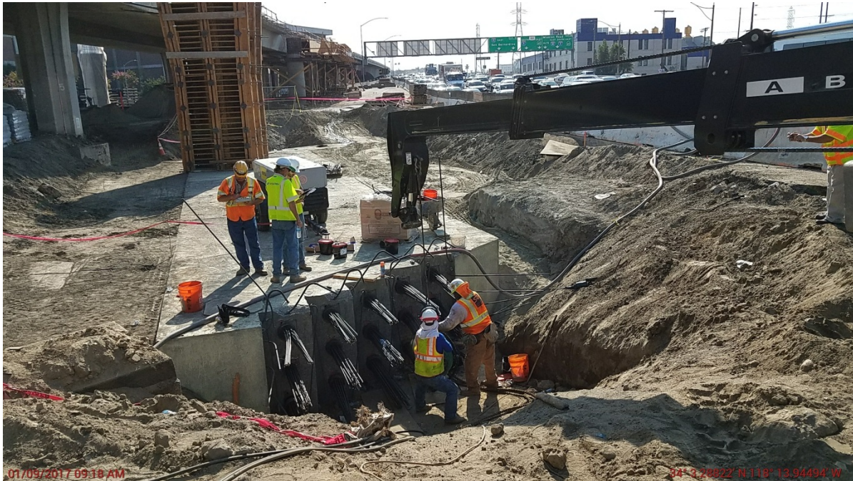
Post Tension at Bent 5 RT.
