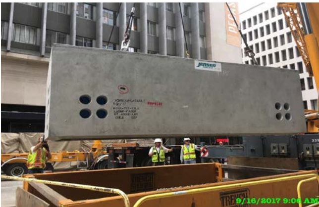
Installation of Vault 621 on Flower north of Wilshire
