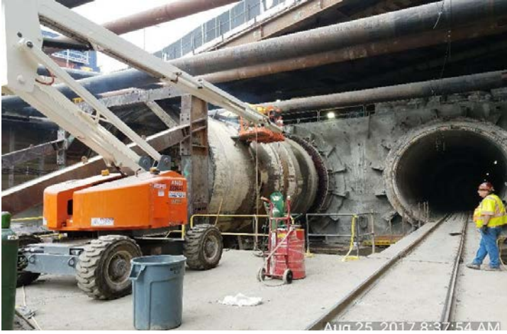
Welding TBM Shield in preparation for re-launch
