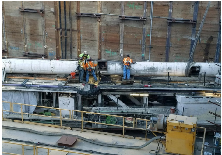
TBM screw replacement installation
