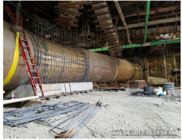
Hobas rebar cage forming at Historic Broadway
