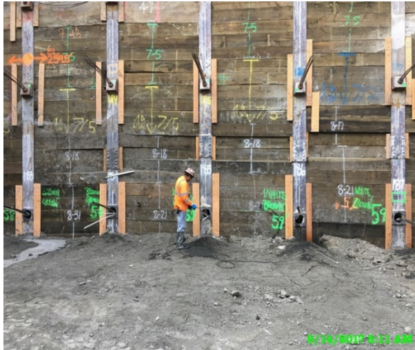
Grouting tie-backs at Level 3 Wall F
