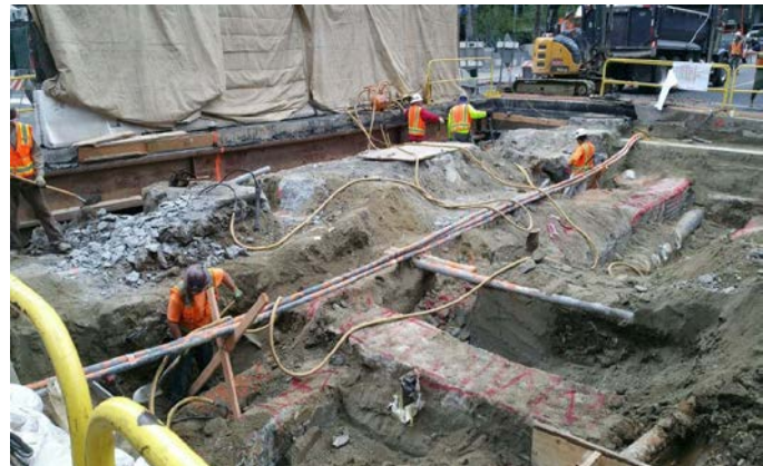
Excavation in preparation for deck beam installation
