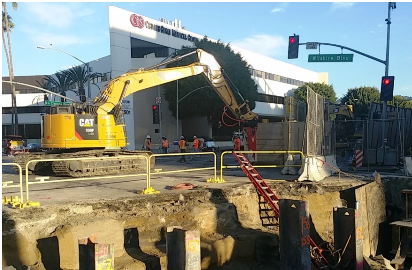
Decking Operation at Wilshire/La Cienega Station
