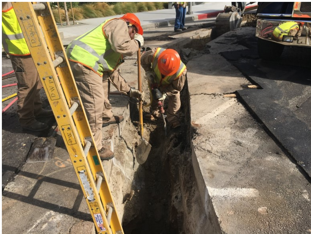
LADWP Power Work in Century City
