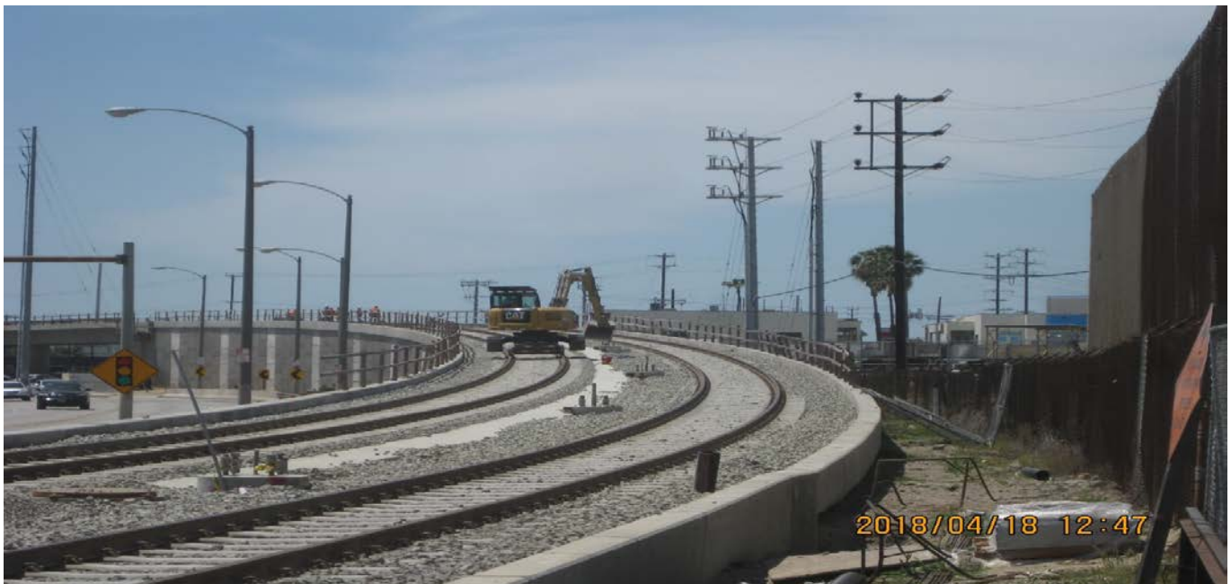
MSE 122L&R – Track 4 top ballast dressing.
