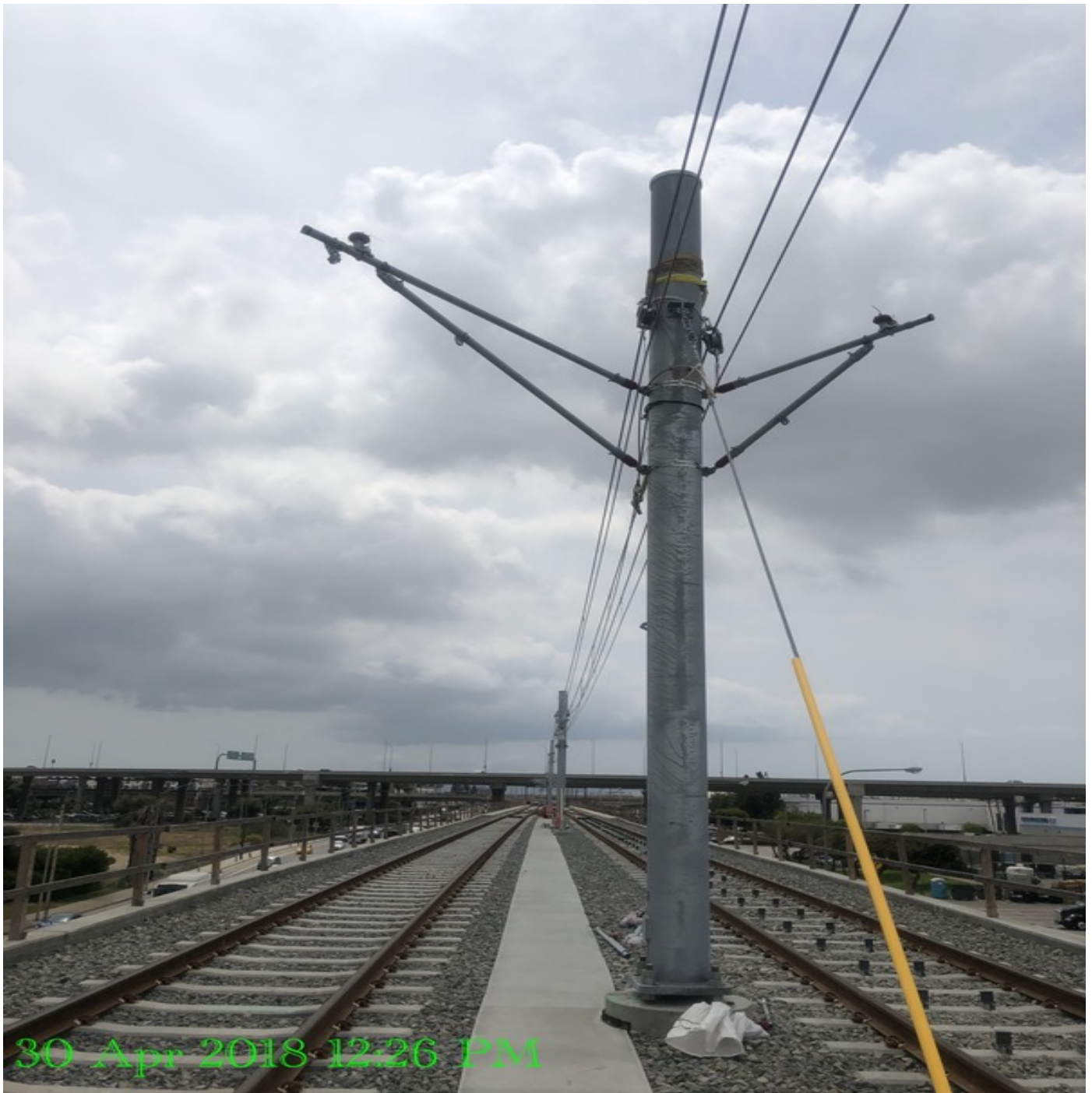
GREENLINE UNDERPASS – Installing 350 MCM contact wire run WR-04 from OCS pole.
