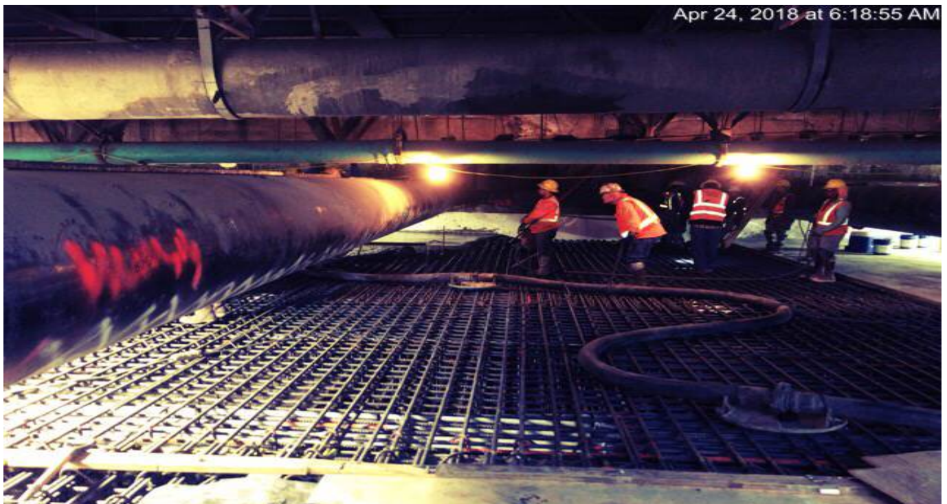
MARTIN LUTHER KING JR. STATION – Rebar at roof section R-12.
