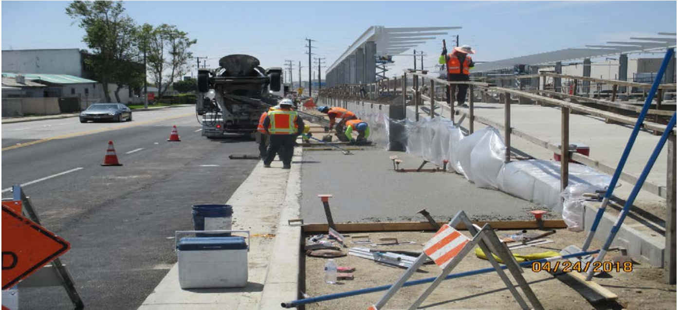
WESTCHESTER STATION - Placing concrete for the sidewalk along the Westchester Station.
