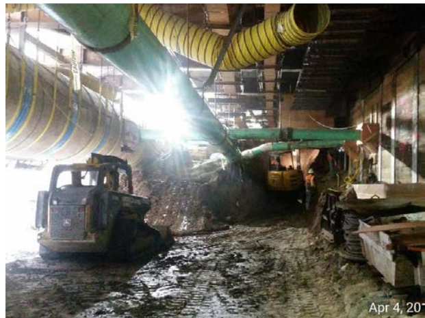
Excavation near South Access Shaft at 5th/Flower
