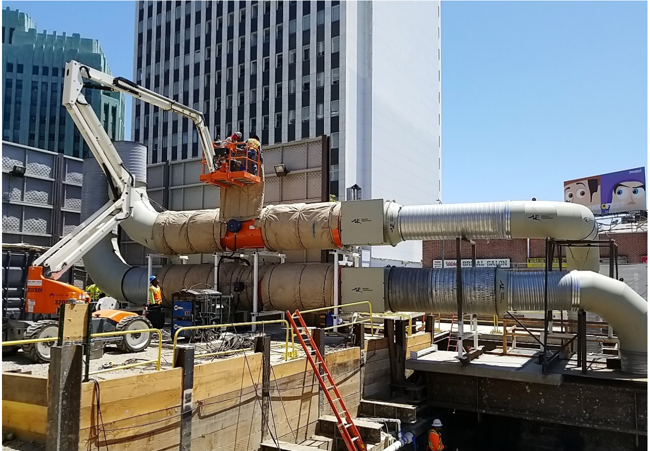
Wilshire/Western TBM Retrieval Shaft Ventilation Equipment Installation
