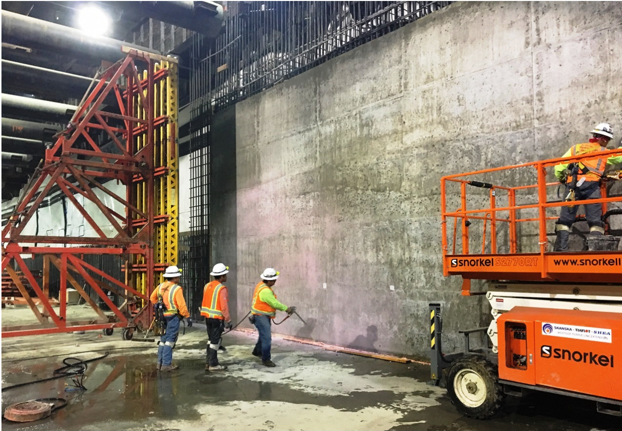
Wilshire/La Brea Station Wall Pours
