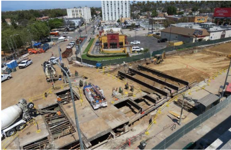
Removing street decking at Vernon Ave/Crenshaw Blvd .
