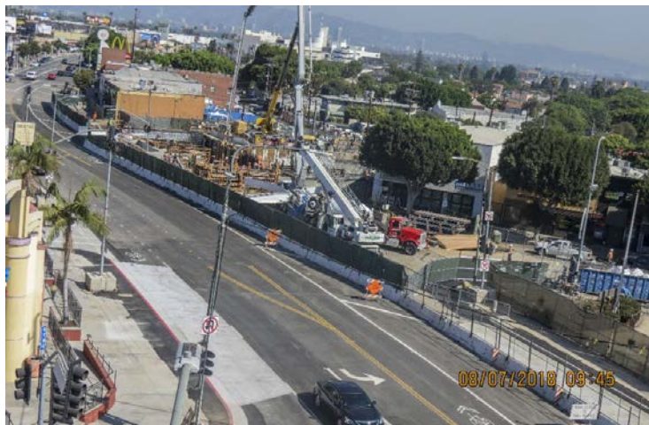
Street restored at Leimert Park Station.
