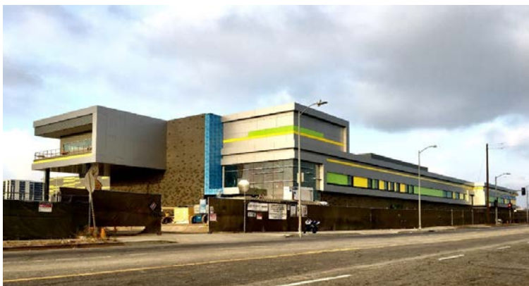
Southwestern Yard Main Shop Building.
