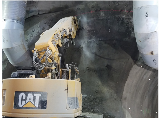
Excavation of SEM Cavern upper center drift
