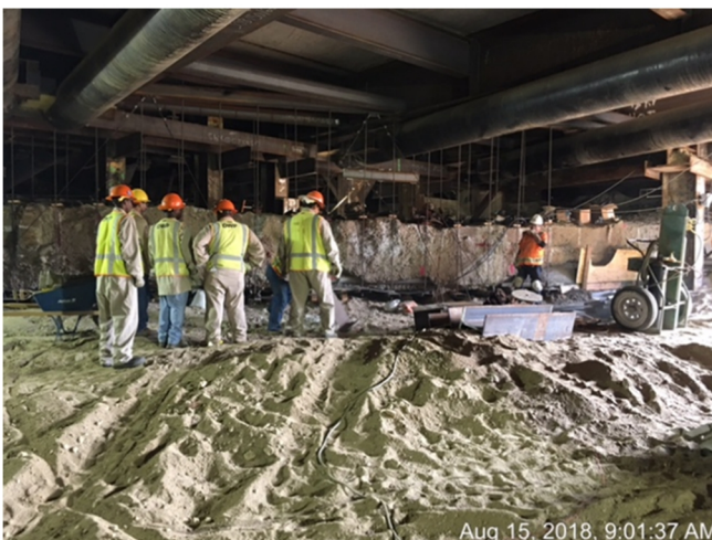
DWP onsite to patch duct bank at Wye and 1 st Street
