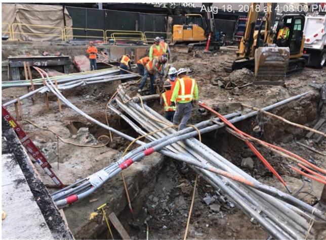
Excavation for deck beams on Flower St
