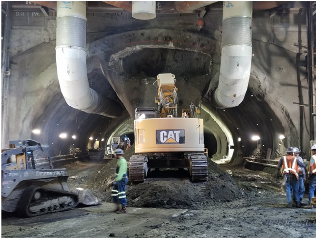
Excavation of SEM Cavern upper center drift
