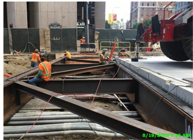
Welding deck beams on Flower St
