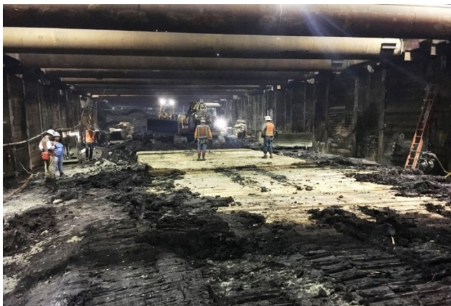
Crane Pads Set near Wilshire/Fairfax Subgrade
