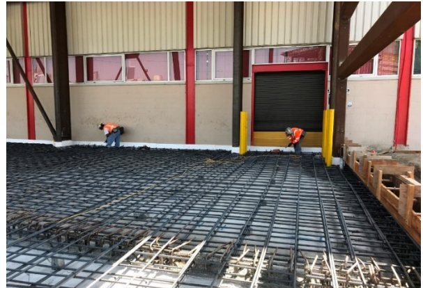
Division 20 Building – Slab on Grade Activities
