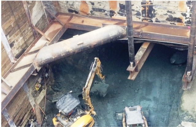
Excavation under the BRS at Wilshire/Western
