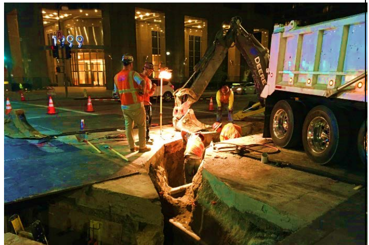
AT&T Utility Trench Work in Century City
