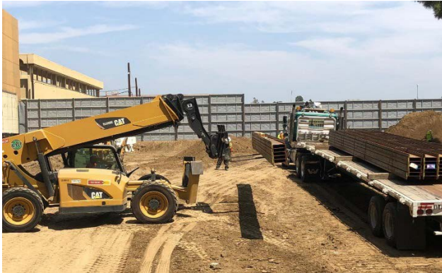
Unloading Steel Posts for Sound Wall at 1940 CPE
