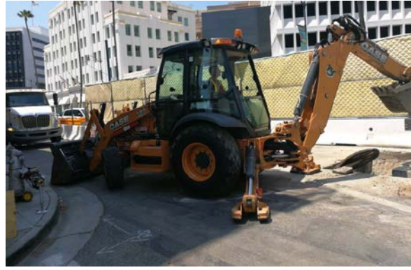
SCG Gas Pipe Excavation in Beverly Hills
