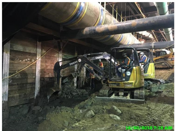
12/20/2018 7:15 AM Excavation and lagging towards bottom level under Flower St
