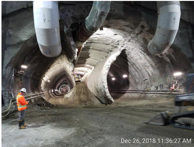
Dec 26, 2018 11:36:27 AM Demolition of temporary center wall in SEM Cavern
