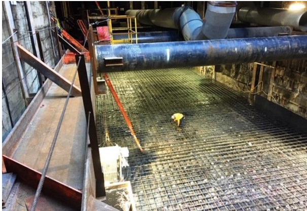
Rebar Installation at Wilshire/Western Retrieval Shaft
