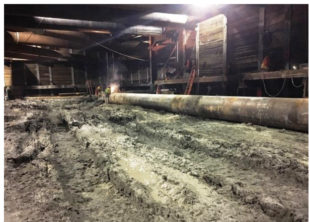
Welding Struts at Wilshire/La Cienega Station
