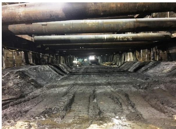
Fine Grading at Wilshire/Fairfax Station
