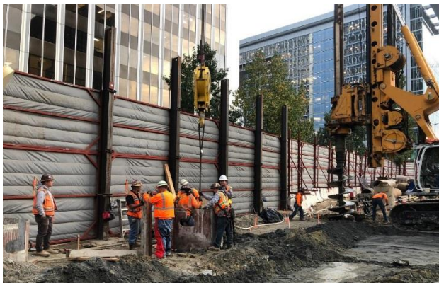
TBM Launch Box Pile Installation in Century City
