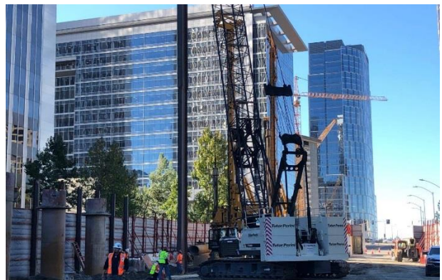
TBM Launch Box Pile Installation in Century City
